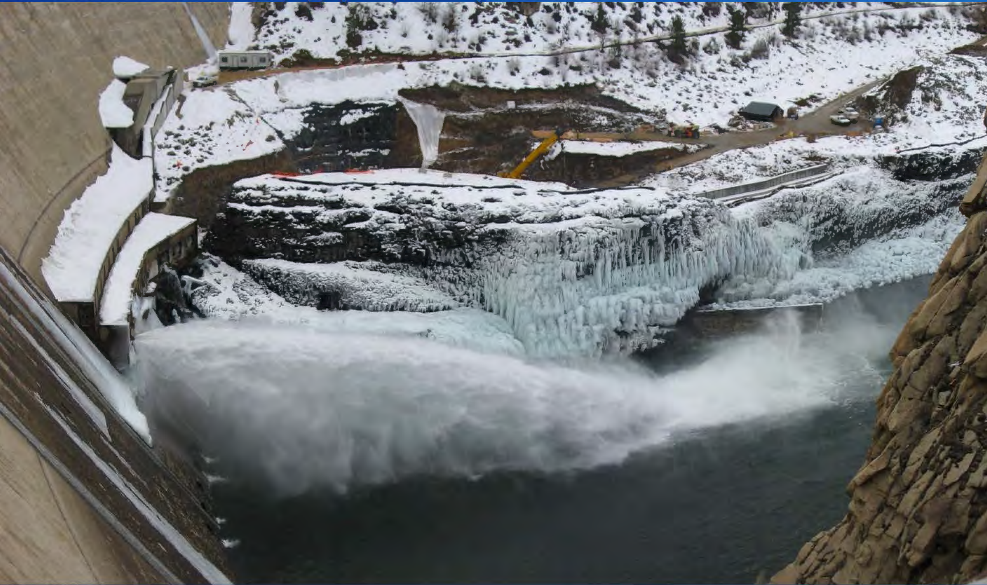
Arrowrock Dam – February, 2009
