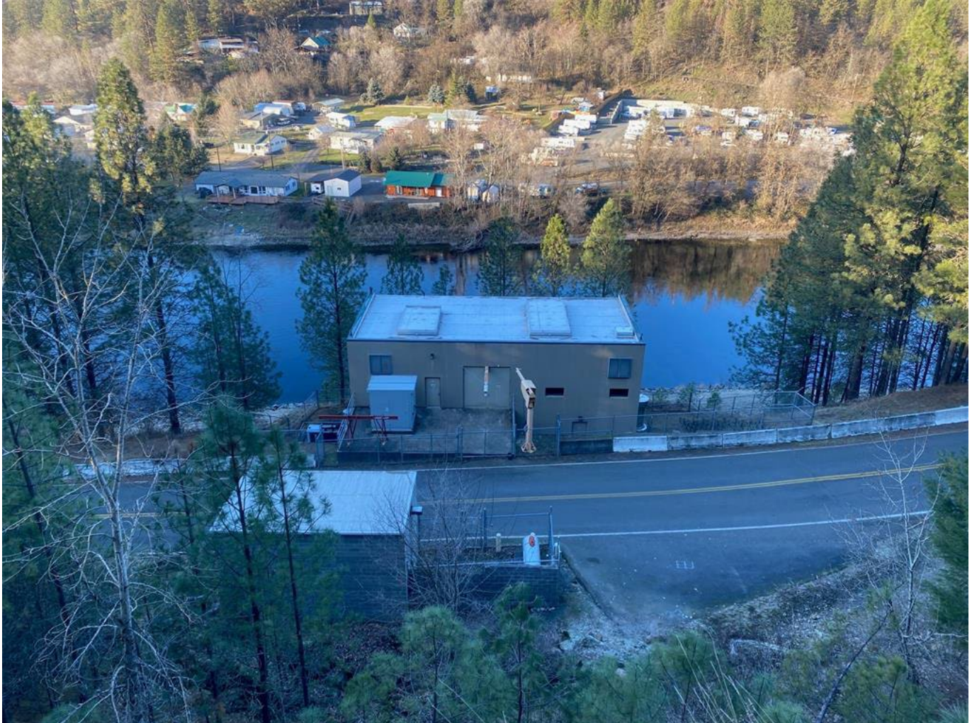
Figure 1: Dworshak Small Hydro Power Plant
