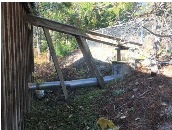
LIFT STATION #2 EXTERIOR DISCHARGE PIPE TO LAGOON
