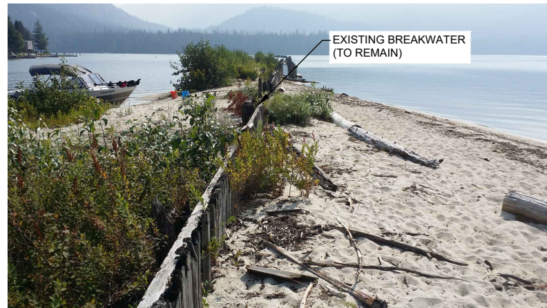
GROUND PHOTO 4 EXISTING BREAKWATER (LOOKING WEST)
