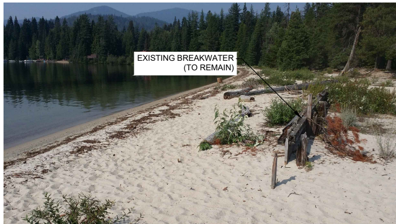
GROUND PHOTO 5 EXISTING TIMBER BREAKWATER (LOOKING WEST)
