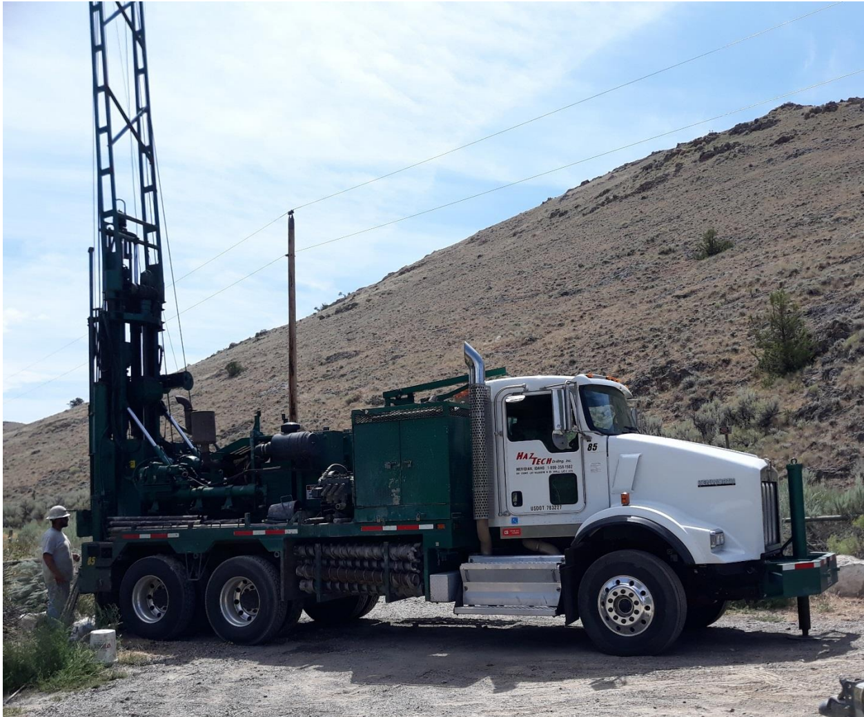
Figure 22. Well rig set up at the Stennett site.
