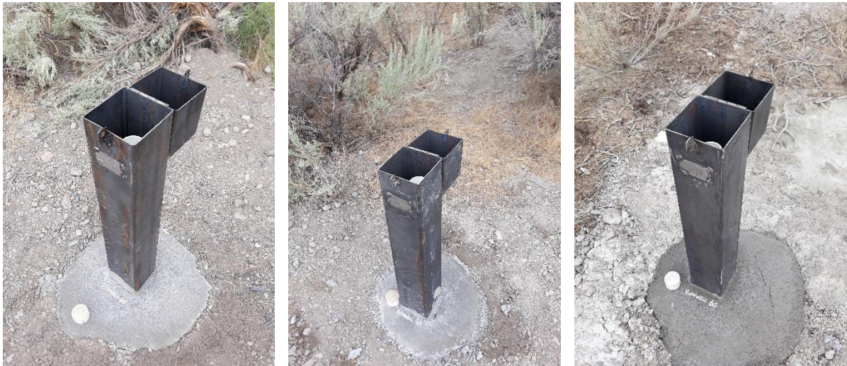
Figure 19. Final wellhead completions at the Rothwell site.
