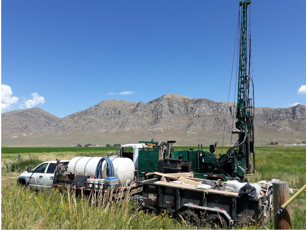
Figure 8. Drill rig set up at the PU Ranch site.
