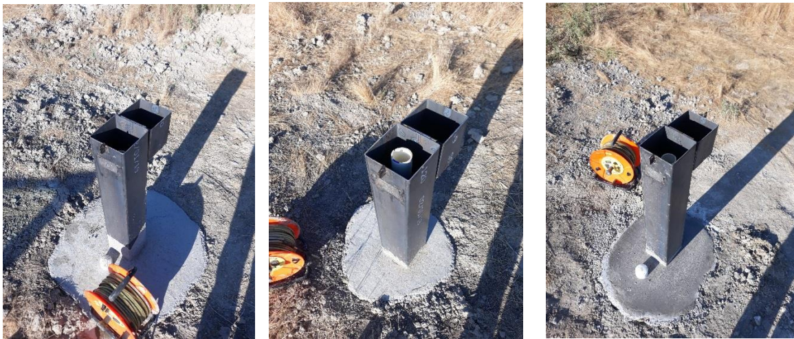
Figure 5. Final well completions at the Walker site.
