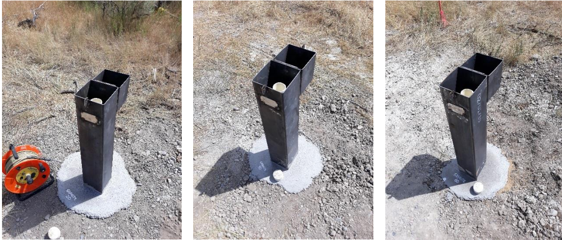
Figure 12. Final wellhead completions for the Granite Trust wells.
