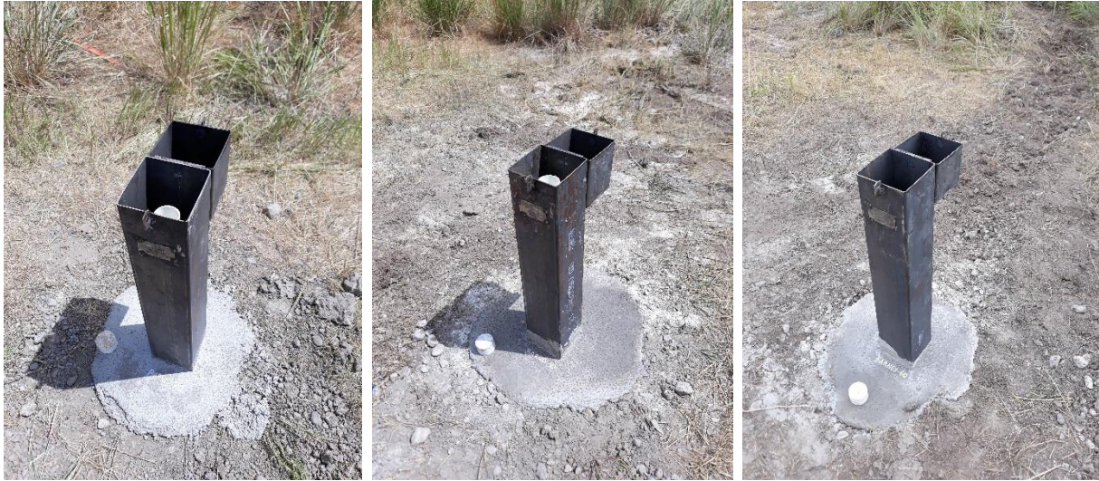
Figure 15. Final wellhead completions for the Barnes site wells.
