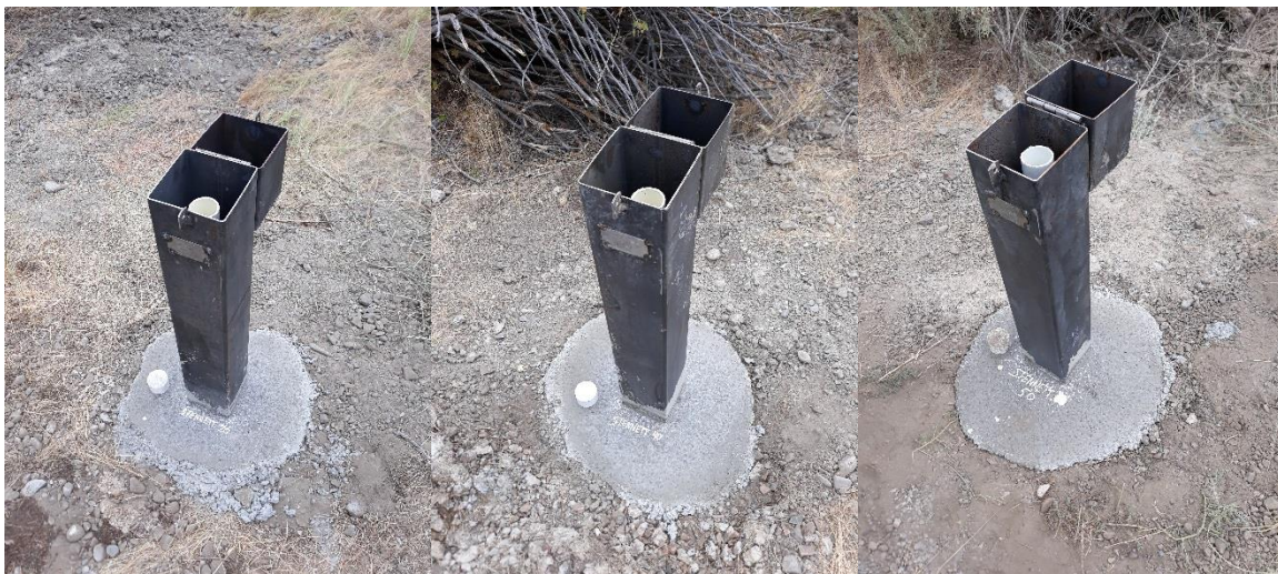
Figure 23. Final wellhead completions at the Stennett site.
