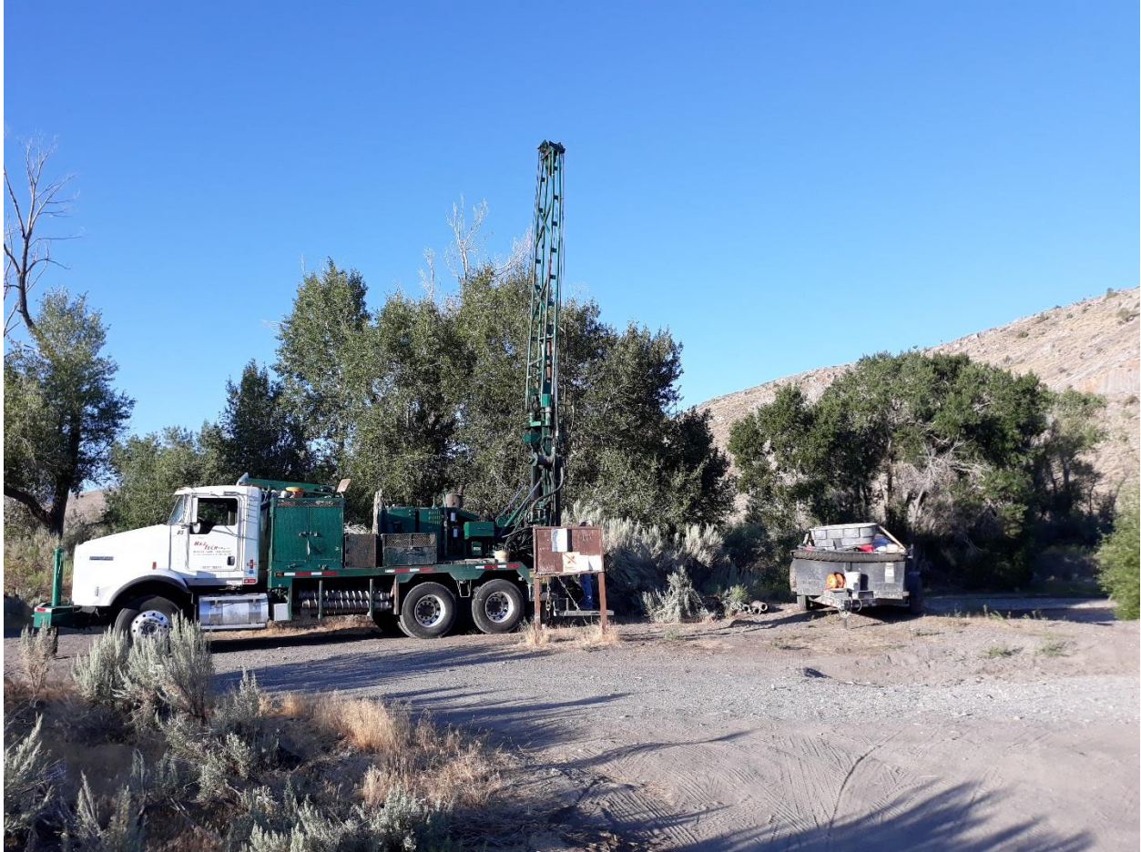
Figure 18. Drill rig at the Rothwell site.
