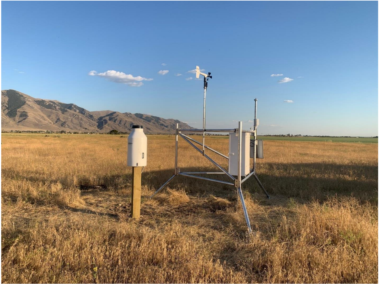
Figure 4. Agrimet weather station installed north of Moore in September 2019.
