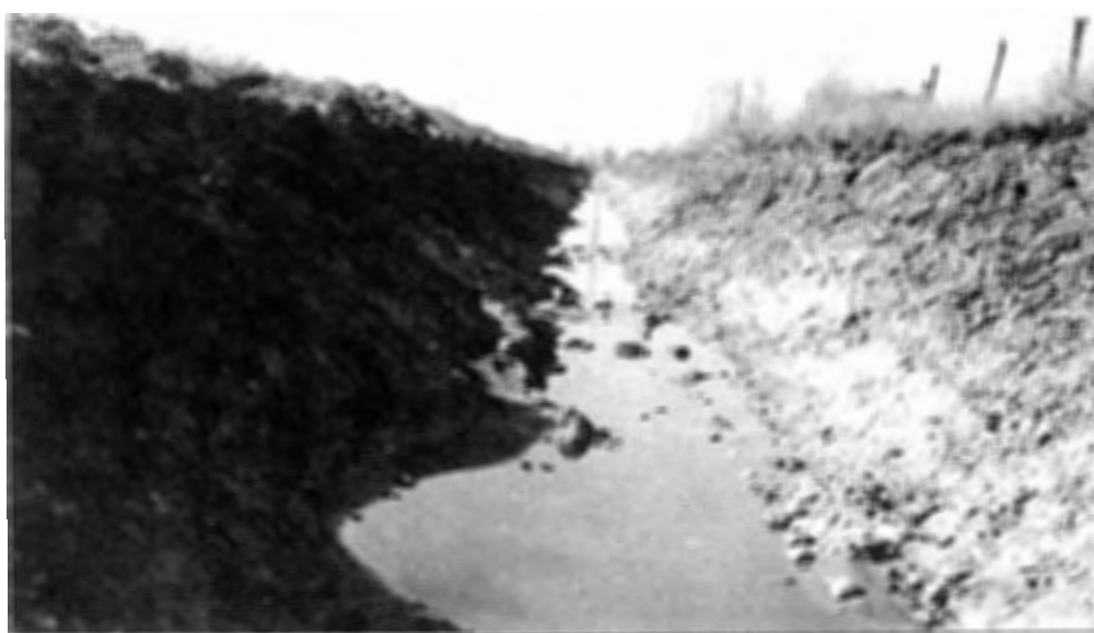
Figure 10. Looking west along open drain, from the north east corner of the farm. Drainable strata of sand and gravel is visible below a two foot soil cap.
