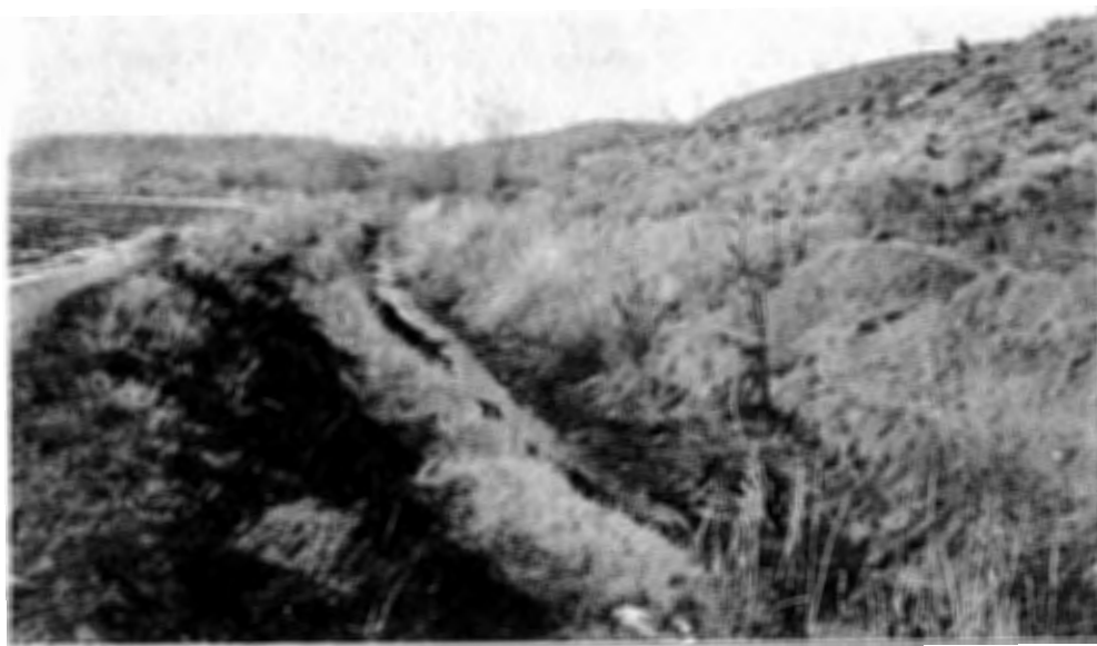
Figure 22. Looking west along the interception drain. The drain is located at the break in grade and soil change to intercept seepage water from the bench.
