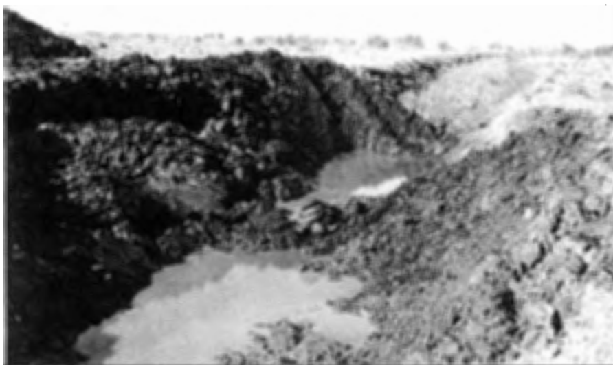
Figure 14. Looking north along partially constructed drain. Caving and sloughing tendency of drain bank is shown.
