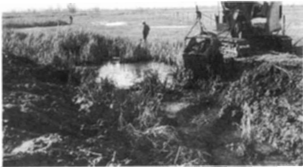
Figure 30. Looking west from south center of farm. Slough is being cleaned and deepened and will be used as an interceptor drain.
