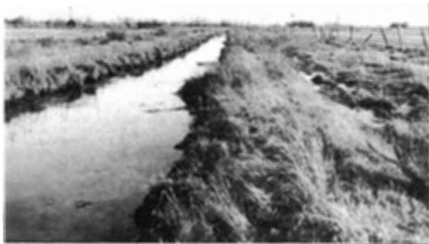
Figure 26. Looking east along shallow ditch at the north side of the farm. The ditch is 1 1/2 feet deep and approximately 12 feet wide.
