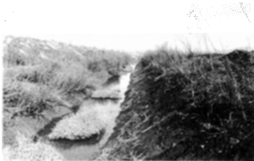
Figure 34. Looking north along section of drain that was installed during 1952. This section of drain is in slowly permeable soil.
