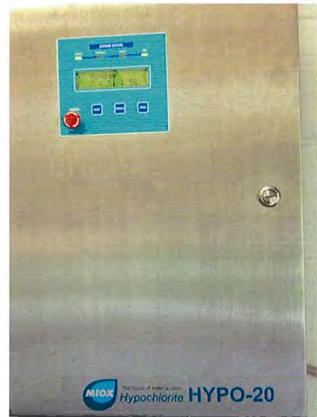
DSCN1562 – Brookwood hypochlorite generation system
