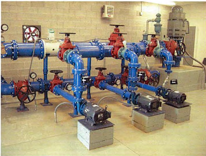
DSCN1567 – Legacy booster pumps from artesian pipe
