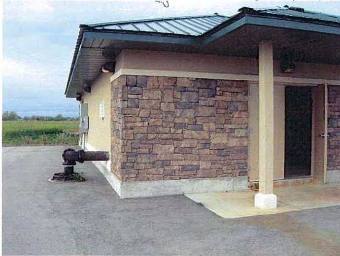
DSCN1566 – Well #4 Legacy showing pump to waste
