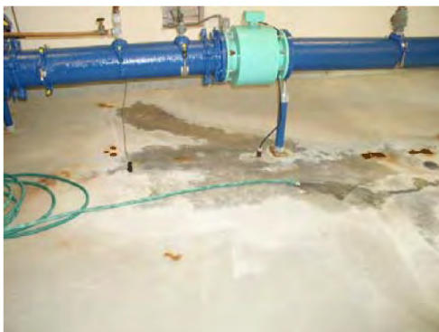
Existing Chlorine Injection Point, Well #1
