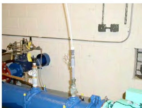
Existing Chlorine Injection Point for Well #3
