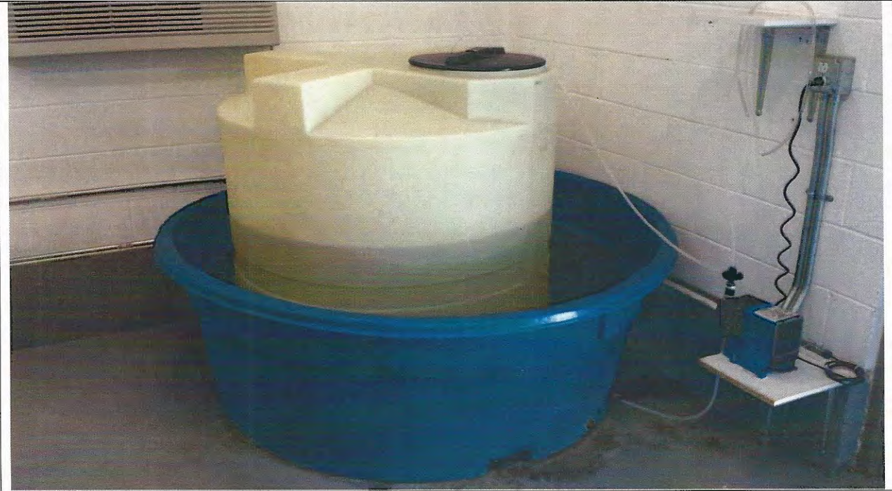
Photo 3: Chlorine Tank with Secondary Containment & Metering Pump for Well #5
