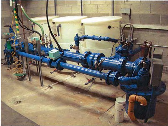
DSCN1565 – Lexington well, piping and chlorination
