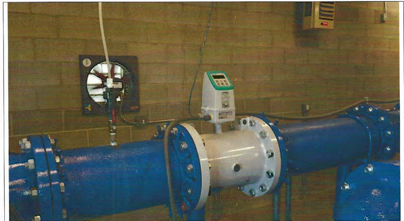
Photo 4: Chlorine Injection Port with Flow Meter
