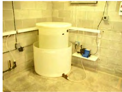
Chlorine tank with secondary containment and metering pump along west wall
