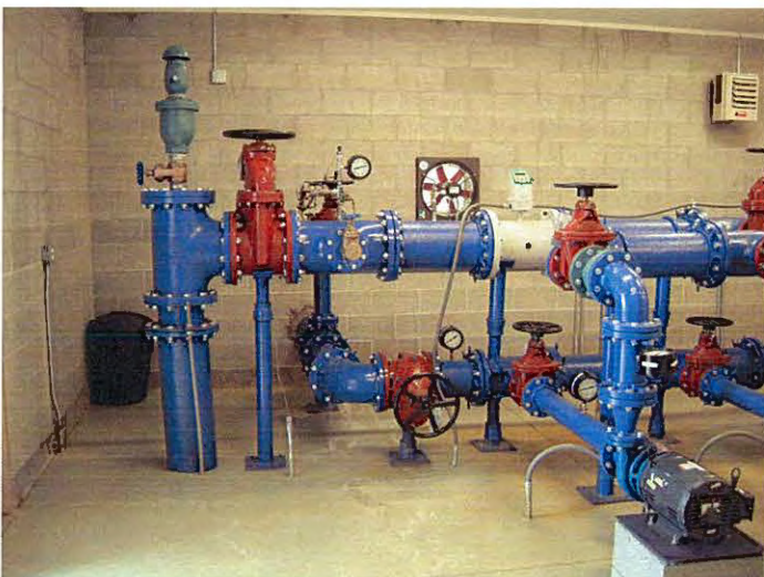
DSCN1568 – Legacy discharge to system and pump to waste
