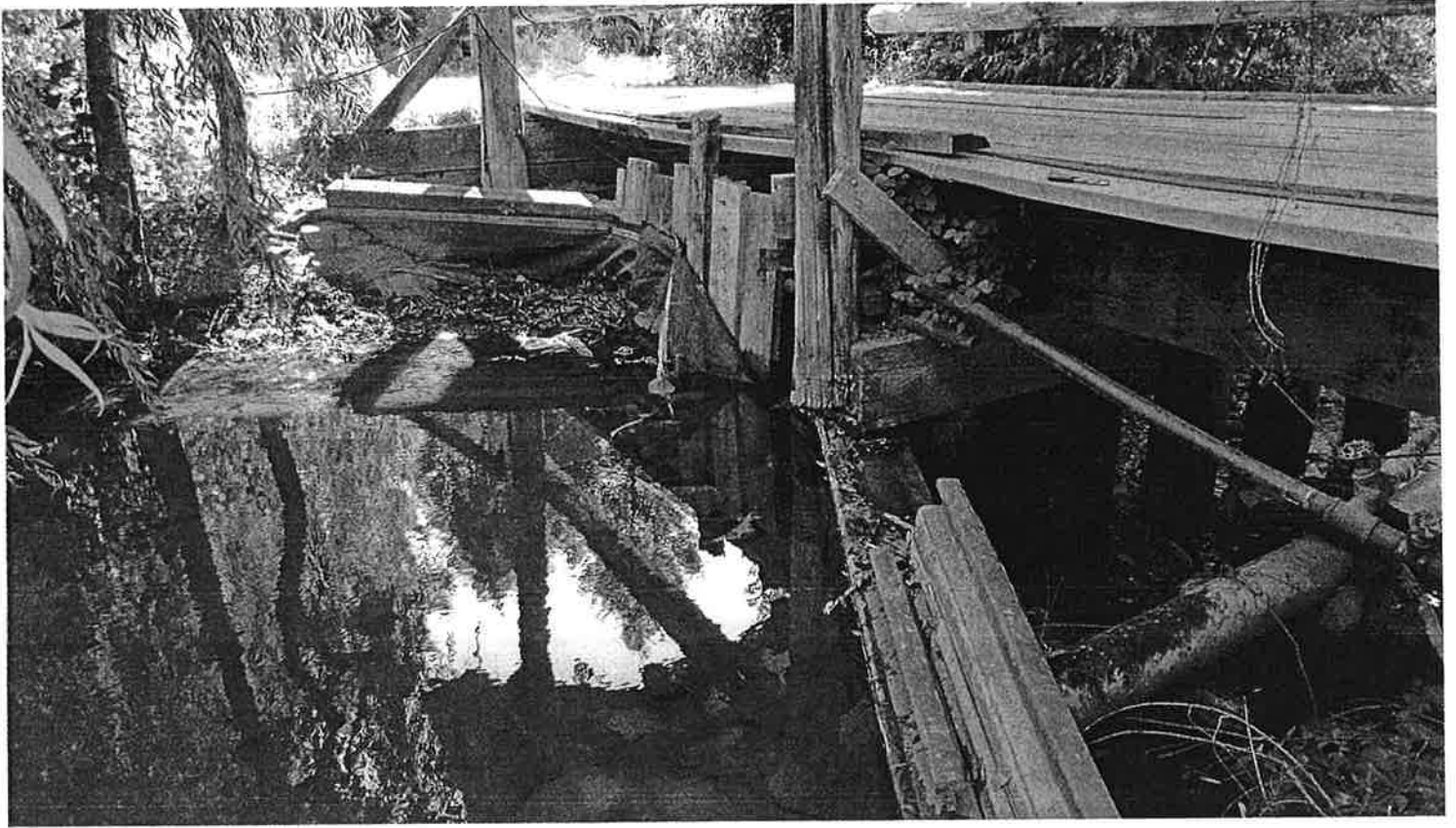
Sylte dam at Bridge
