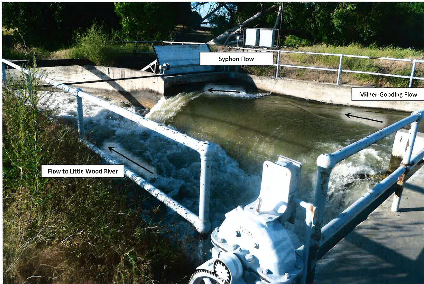
Figure 11: Photograph taken on July 22 nd of the bifurcation, where the Milner-Gooding Canal can inject water into the Little Wood River or flow through a syphon tube under the Little Wood River.
