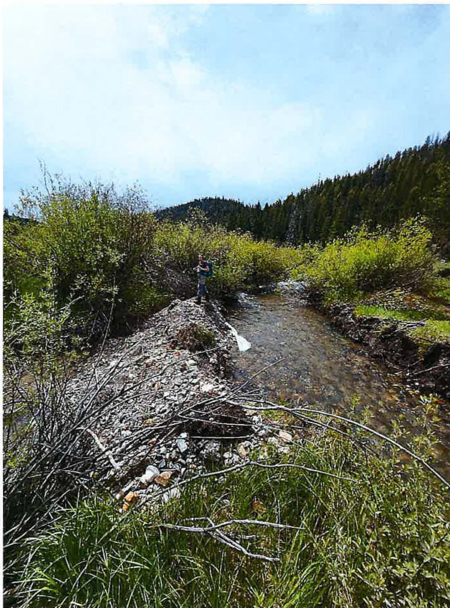
Photo 1: Earthen dam diverting all water from Panther Creek into man-made channel.
