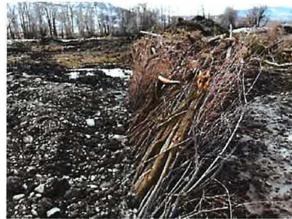
ABOVE: WILLOW TRENCH DURING CONSTRUCTION (LEMHI RIVER, ID)
