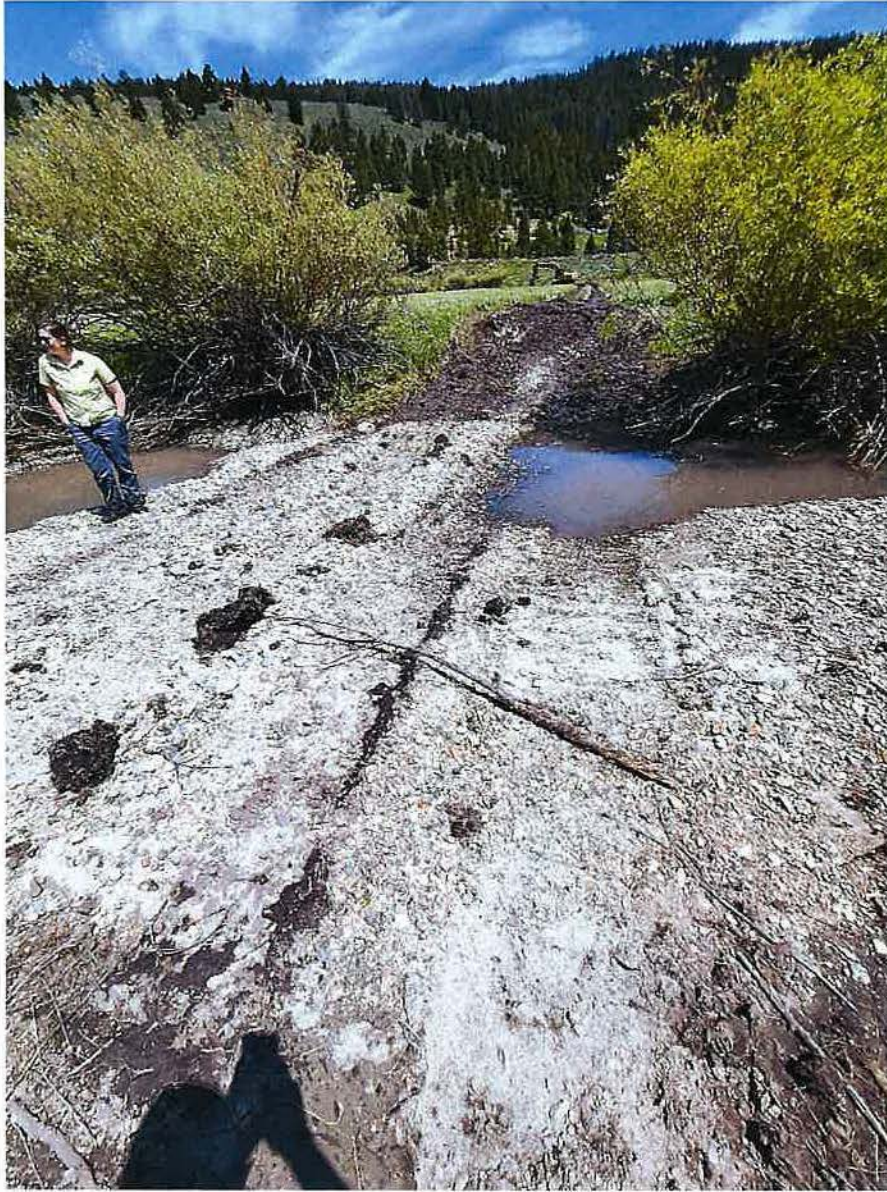
Photo 5: Creek disturbance for excavator crossing.
