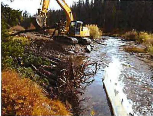
Installing rootwad base
