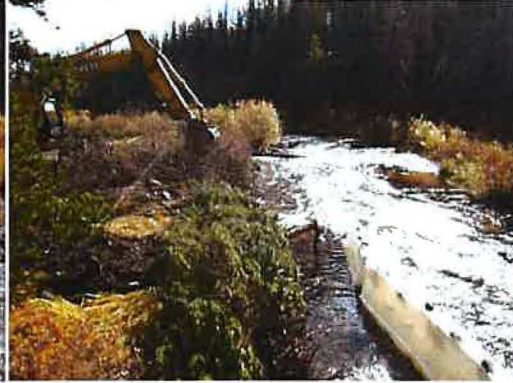
Installing willow clumps
