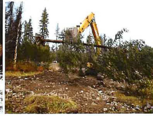
Transporting face revetment
