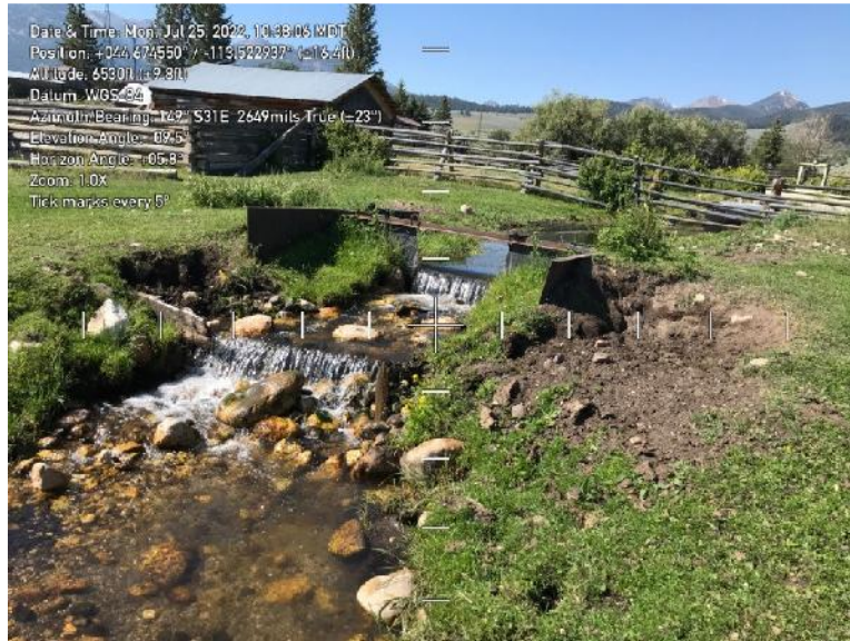
Photo 1. Cipolletti weir at Point D in Map 2. The camera was facing approximately south.
