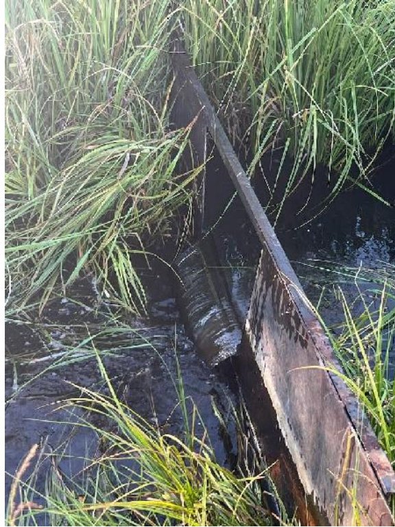
Photo 6. East Springs weir after maintenance. Photo provided by Jordan Whittaker, August 3, 2022.
