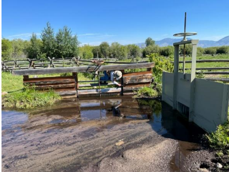
Photo 2. Green Headgate (right) and Check Structure (center).
