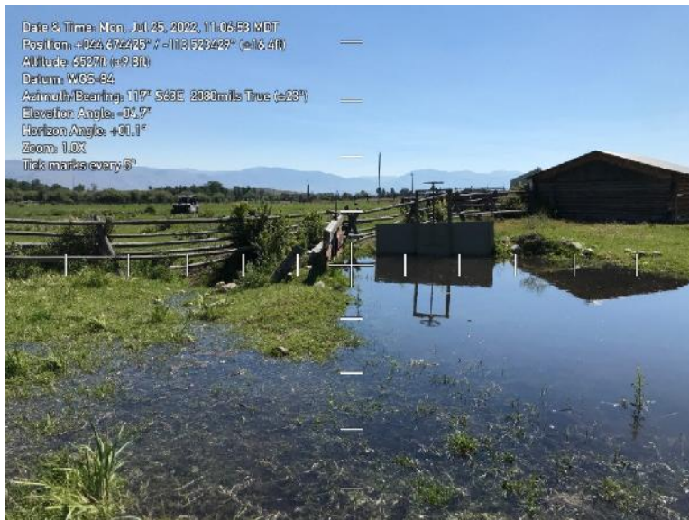
Photo 3. Water bypassing the Check Structure. The camera was facing approximately east from near Point C.
