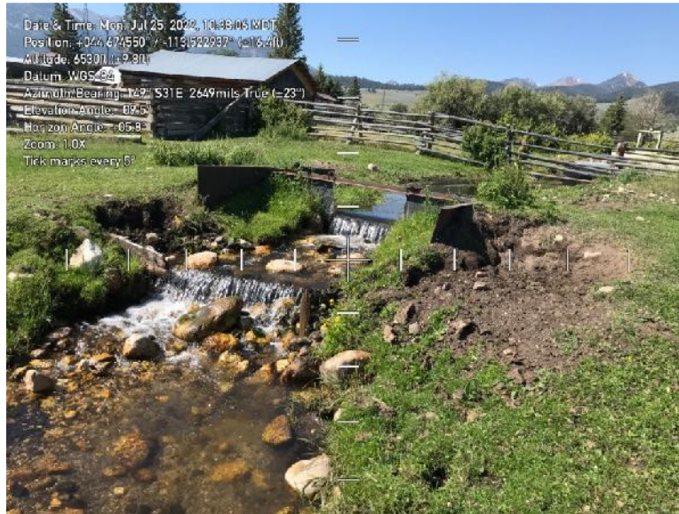
Photo 1. Cipolletti weir at Point D in Map 2. The camera was facing approximately south.
