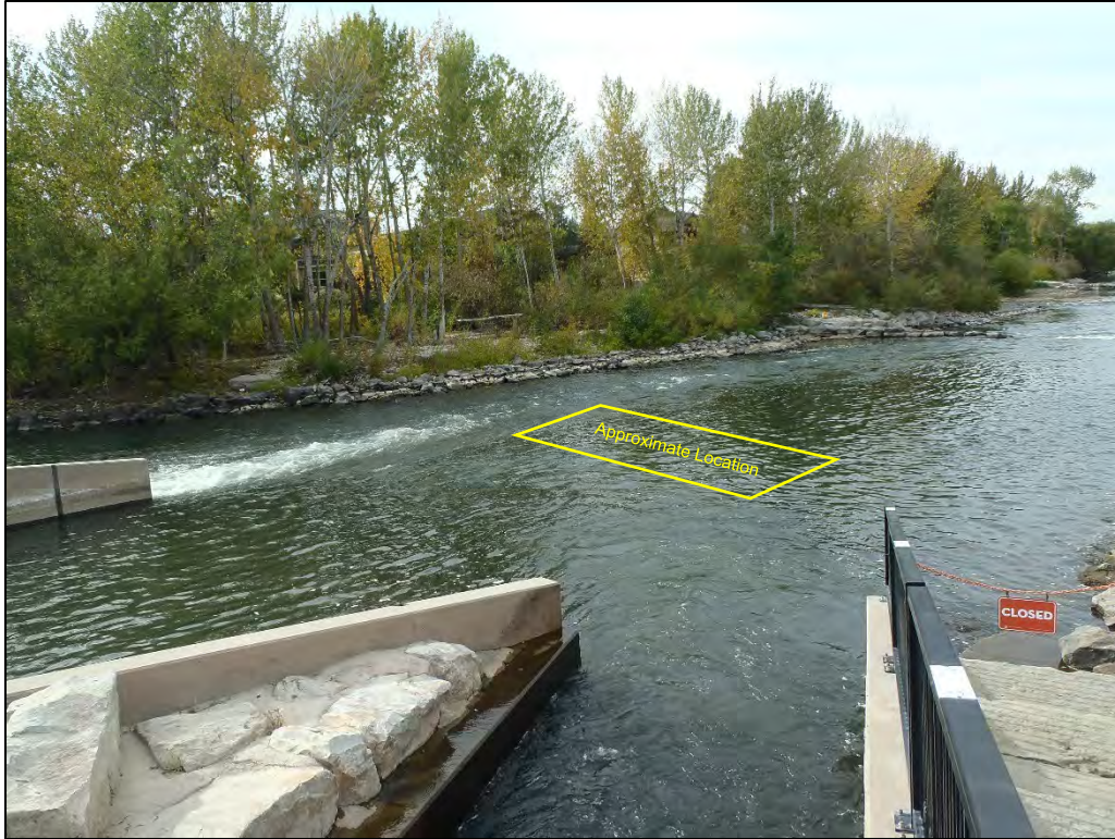
Photograph 7. New Obermeyer Weir Location Downstream of Wave Shaper looking Downstream (October 2023).
