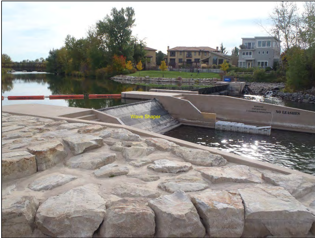
Photograph 5. Drop Structure 1 Wave Shaper looking Upstream (October 2023).
