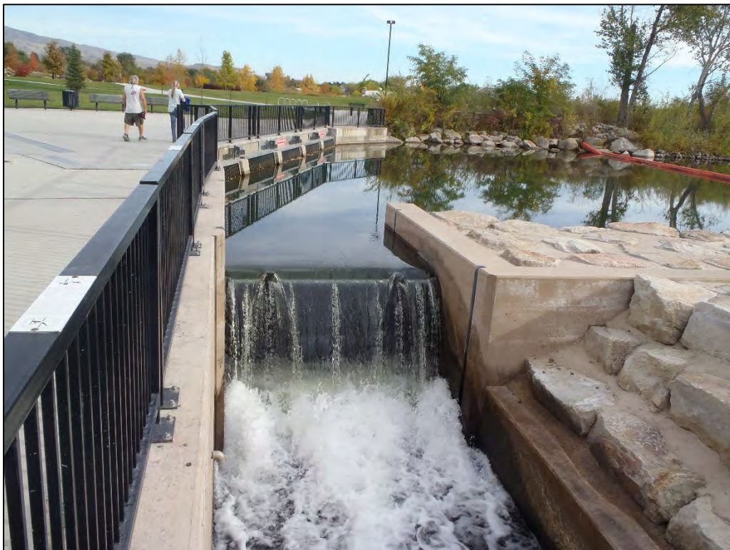
Photograph 6. Drop Structure 1 Sluiceway looking Upstream (October 2023).
