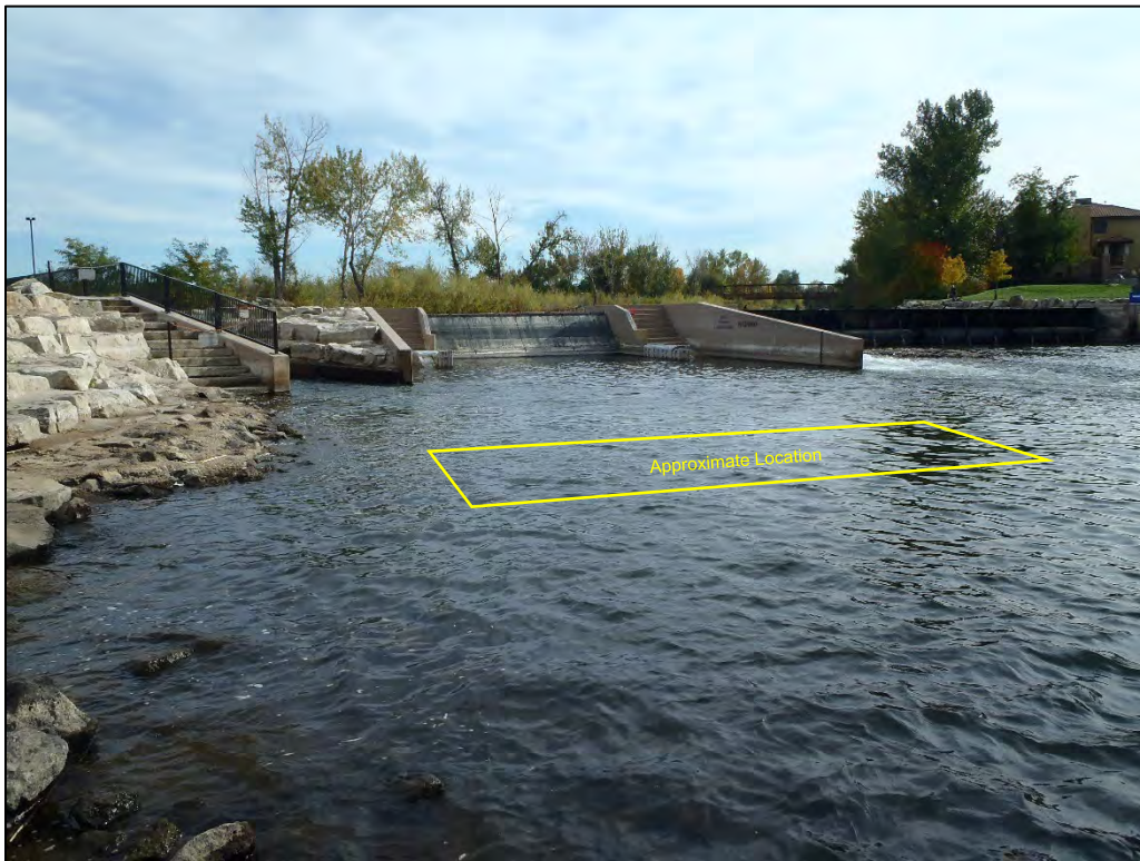
Photograph 8. New Obermeyer Weir Location Downstream of Wave Shaper looking Upstream (October 2023).
