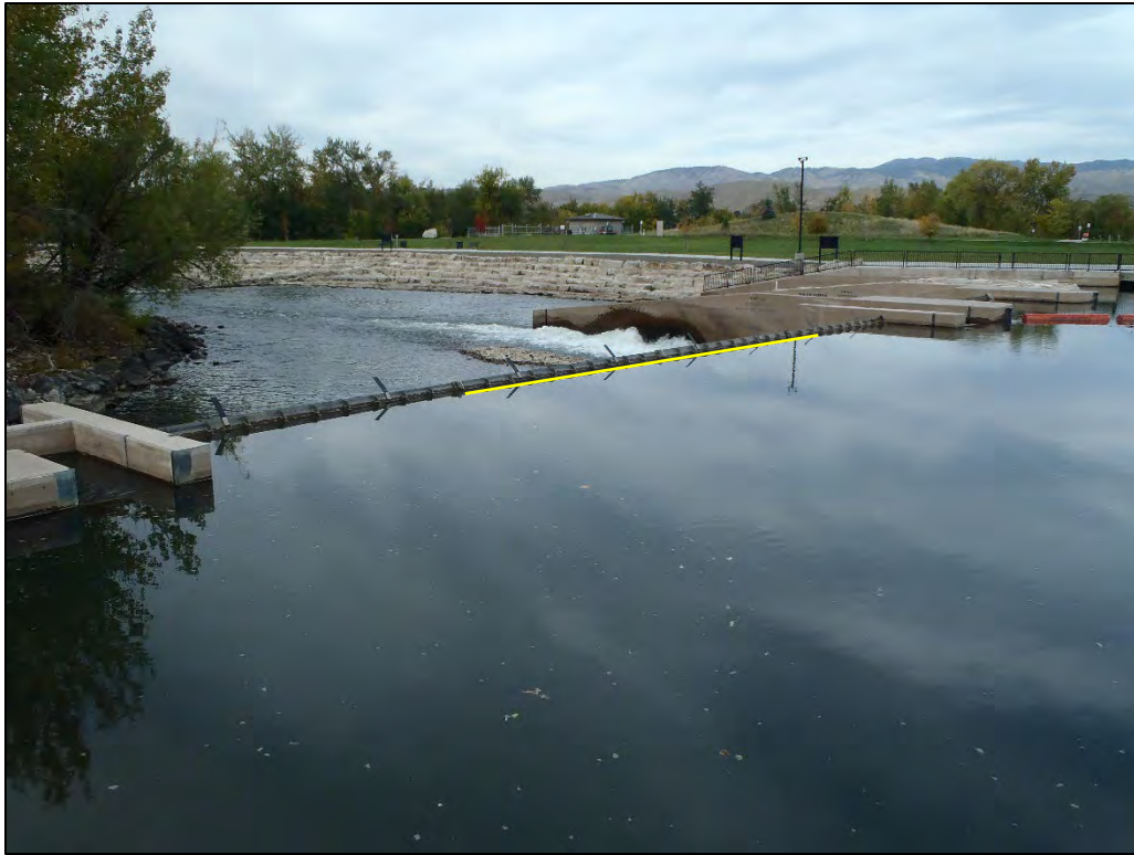
Photograph 1. Drop Structure 1 Gates 5 & 6 looking Downstream (October 2023).
