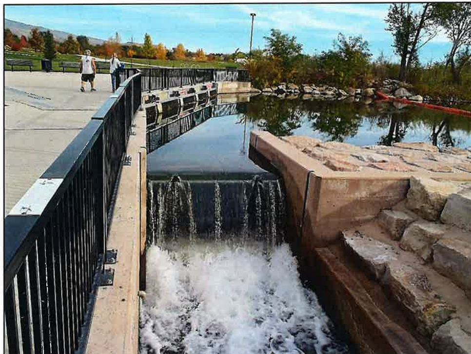
Photograph 6. Drop Structure 1 Sluiceway looking Upstream (October 2023).
