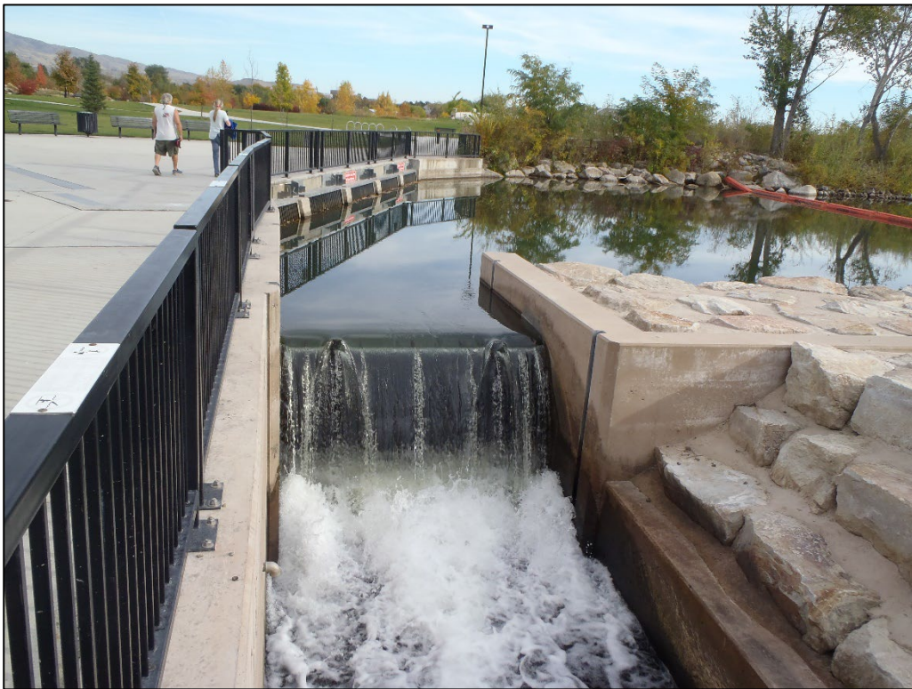
Photograph 6. Drop Structure 1 Sluiceway looking Upstream (October 2023).
