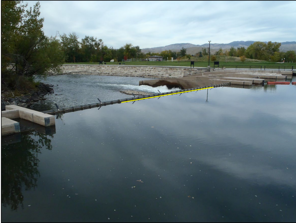
Photograph 1. Drop Structure 1 Gates 5 & 6 looking Downstream (October 2023).
