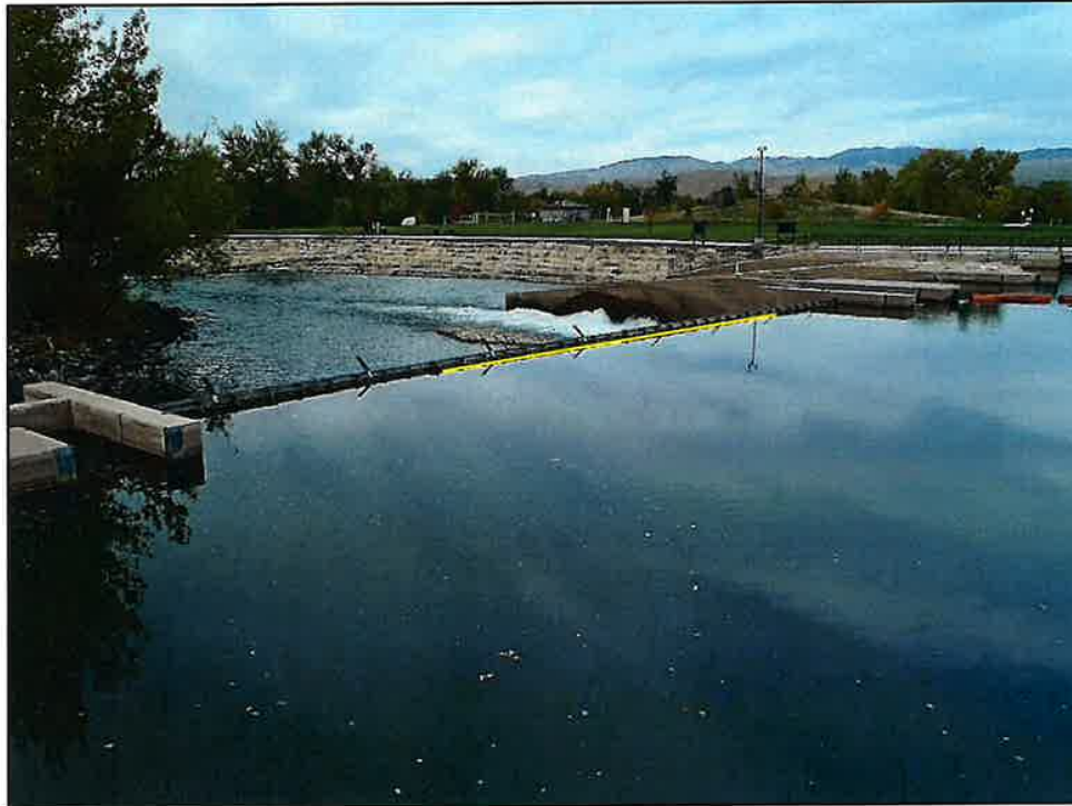
Photograph 1. Drop Structure 1 Gates 5 & 6 looking Downstream (October 2023).
