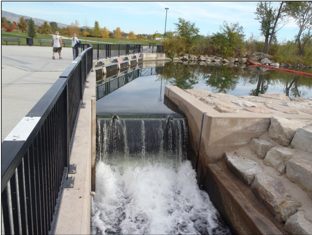
Photograph 6. Drop Structure 1 Sluiceway looking Upstream (October 2023).
