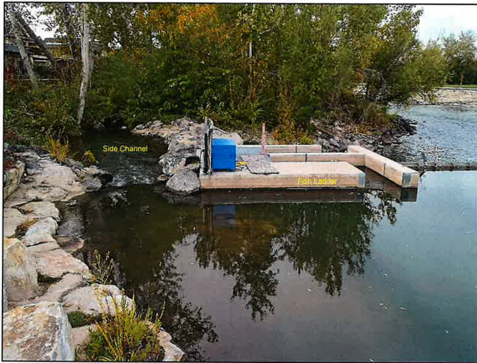
Photograph 3. Left Bank Side Channel Entrance and Fish Ladder looking Downstream (October 2023).
