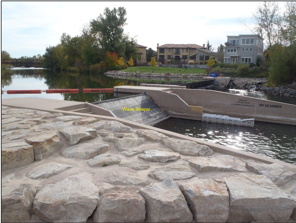
Photograph 5. Drop Structure 1 Wave Shaper looking Upstream (October 2023).
