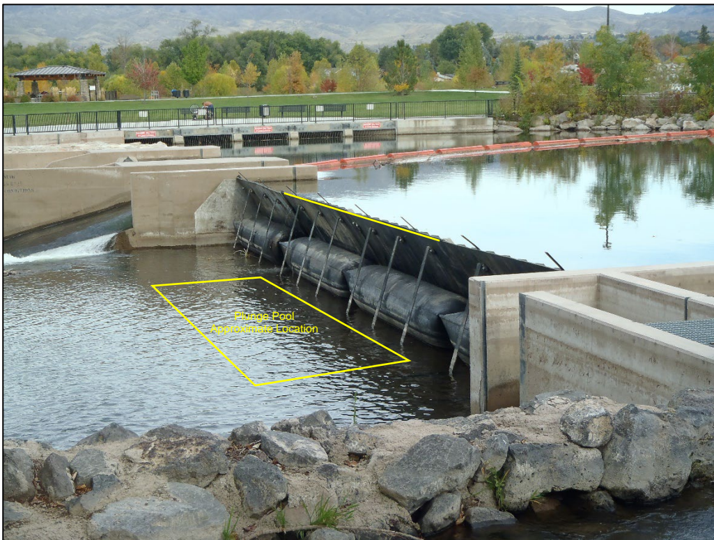
Photograph 2. Drop Structure 1 Gates 5 & 6 and Plunge Pool Area looking Upstream (October 2023).
