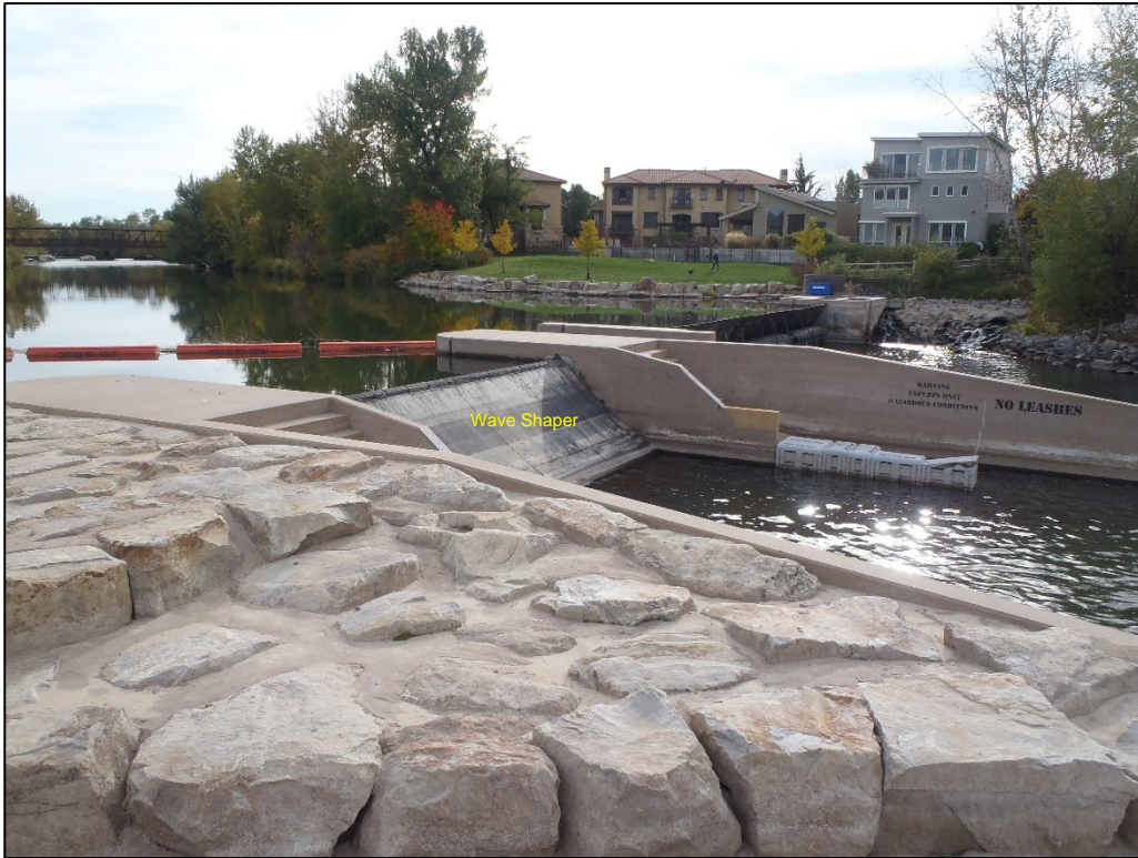
Photograph 5. Drop Structure 1 Wave Shaper looking Upstream (October 2023).
