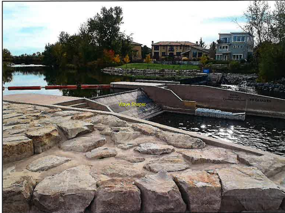
Photograph 5. Drop Structure 1 Wave Shaper looking Upstream (October 2023).
