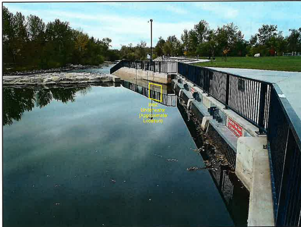
Photograph 9. Temporary Diversion Pipe Inlet above Drop Structure 1 (October 2023).
