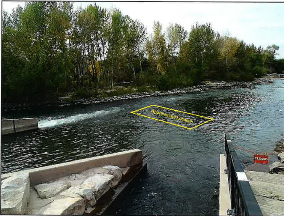
Photograph 7. New Obermeyer Weir Location Downstream of Wave Shaper looking Downstream (October 2023).
