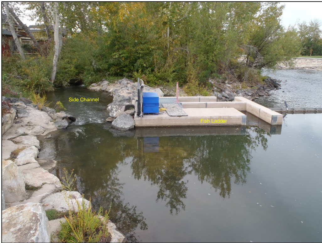
Photograph 3. Left Bank Side Channel Entrance and Fish Ladder looking Downstream (October 2023).
