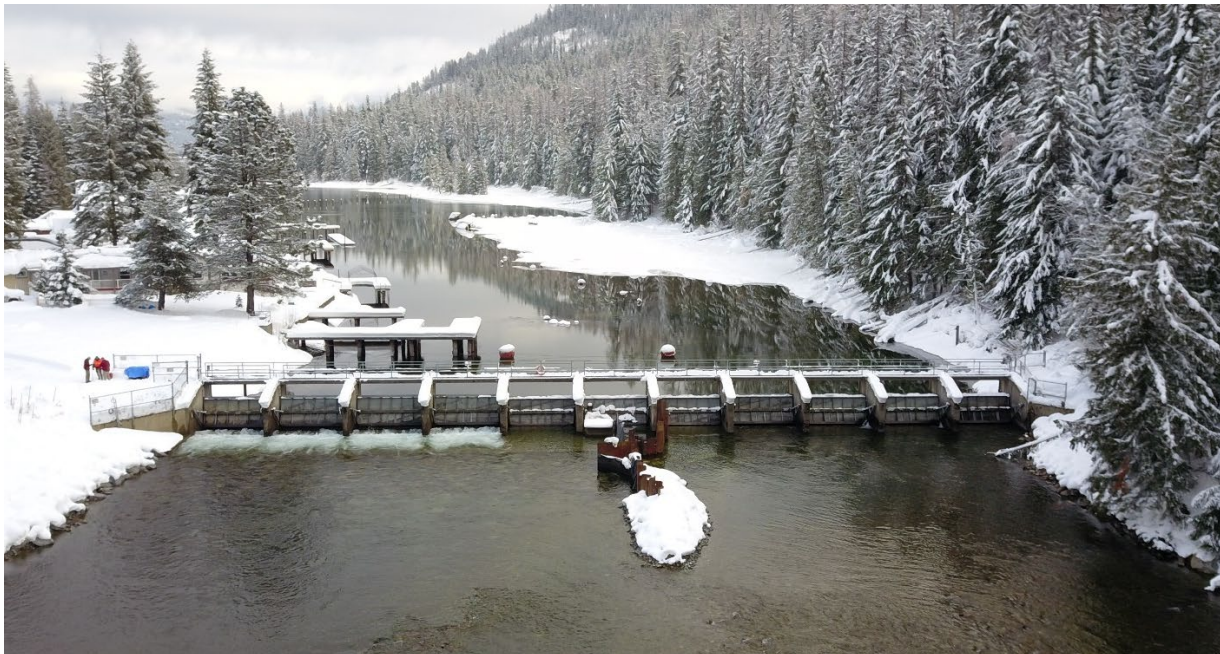
Figure 1: Existing Dam Outlet Structure
