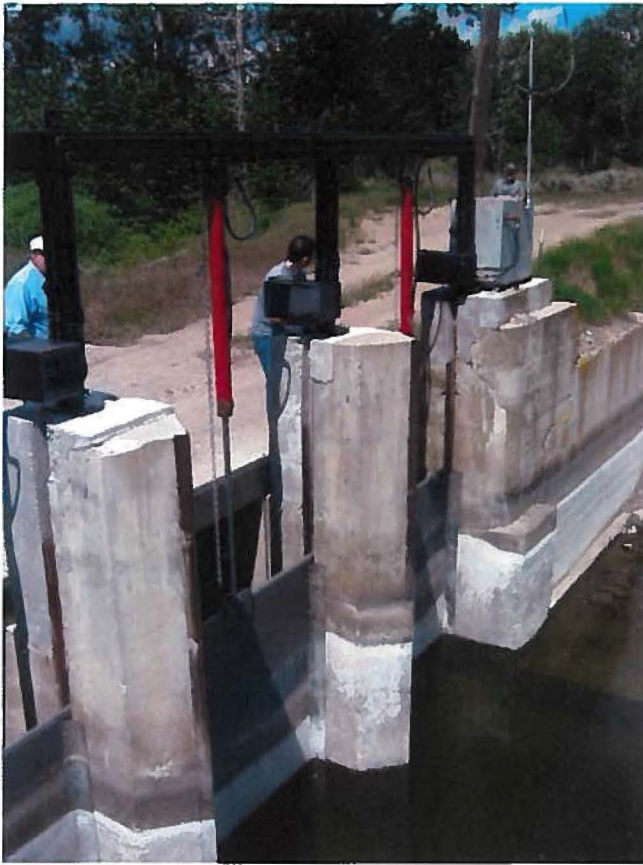
6. Richfield Canal hydraulic spillway slide gates.
