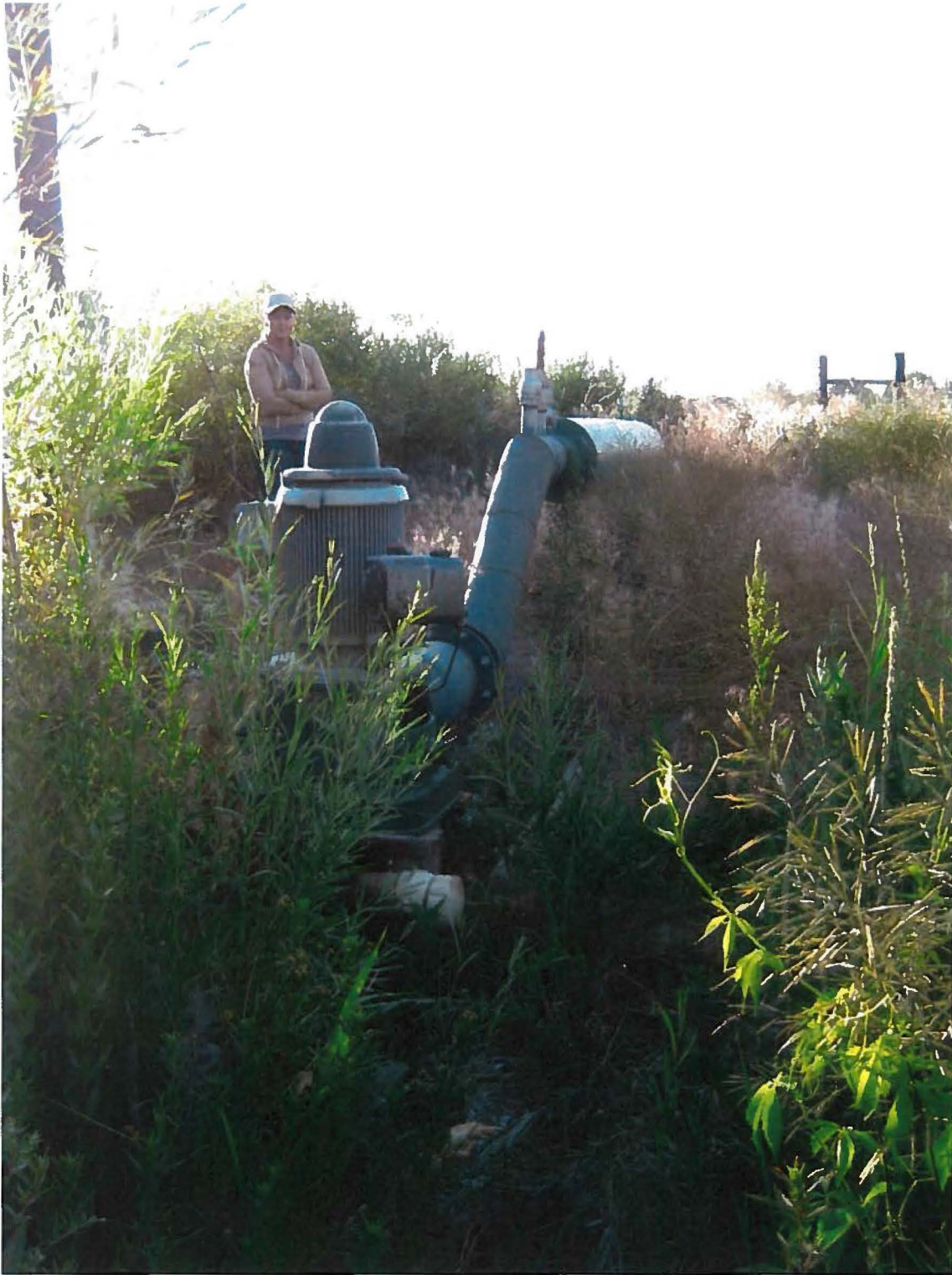
3. Kuntz 98 P2W: view of 30 HP motor/pump, mainline and dragon filter.
