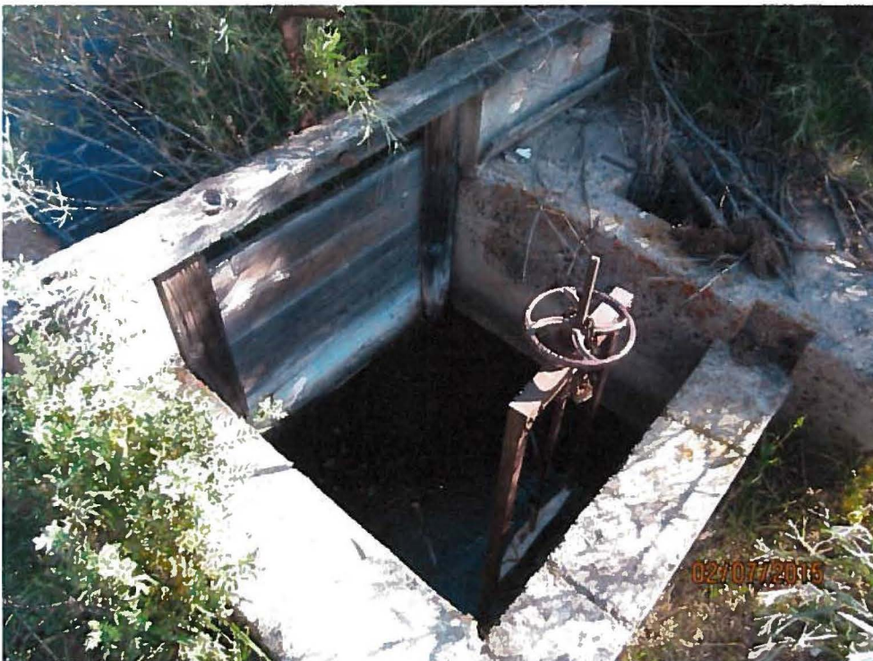
2. Turner 61: orifice-head gate control box, buried mainline connected to head gate.
