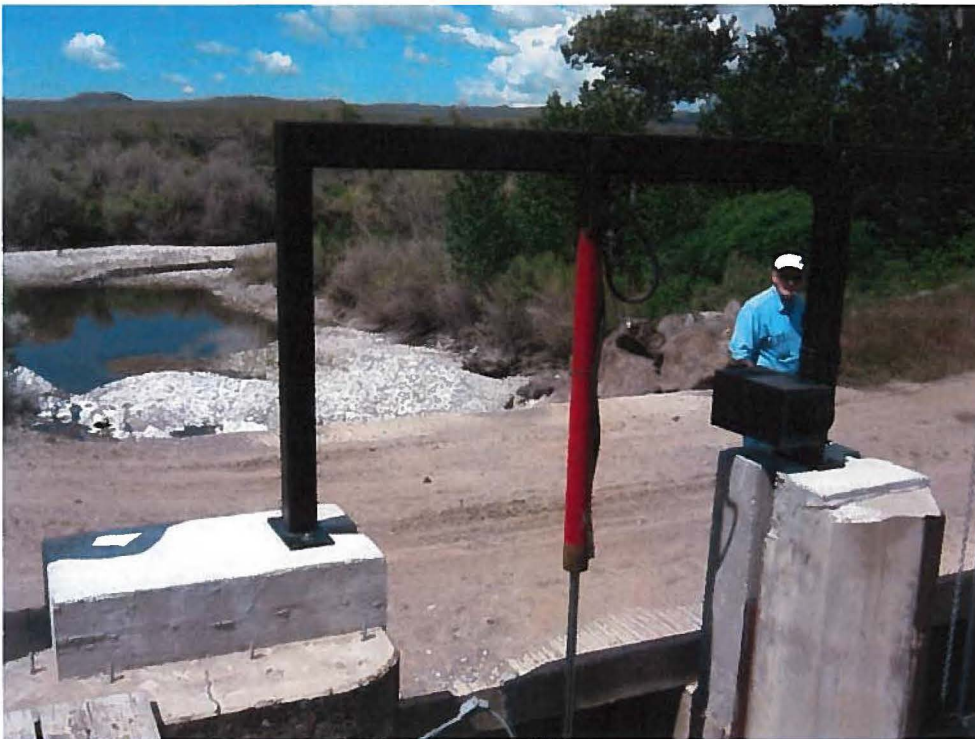
5. Richfield Canal: Spill gates in foreground, water spills to Big Wood River In background.
