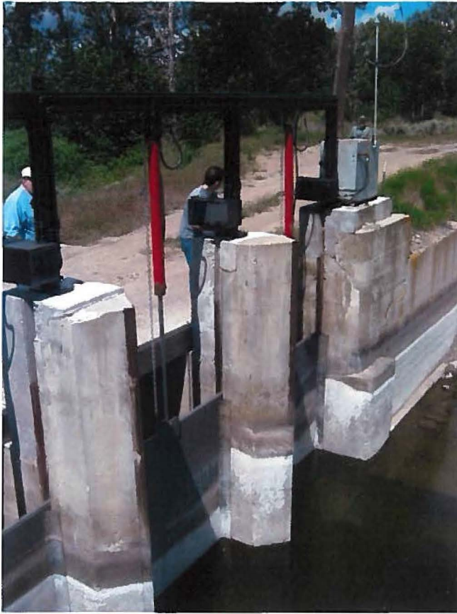
6. Richfield Canal hydraulic spillway slide gates.
