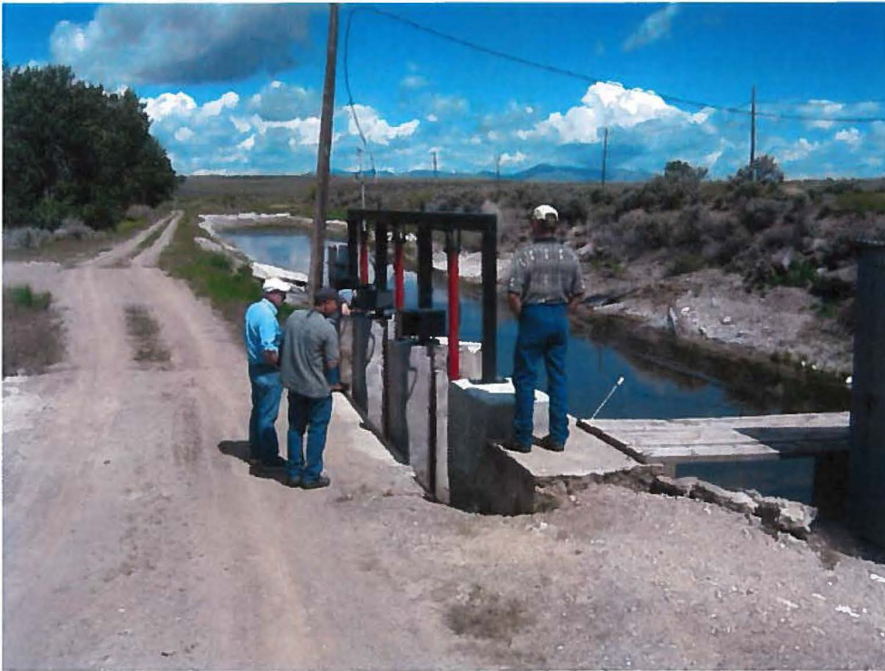
4. Richfield Canal: Spillway gates located on canal downstream of main canal gates and river diversion dam about 365 yards. Water spills to the Big Wood River (located to the left of the photo). Check structure across canal to the right.
