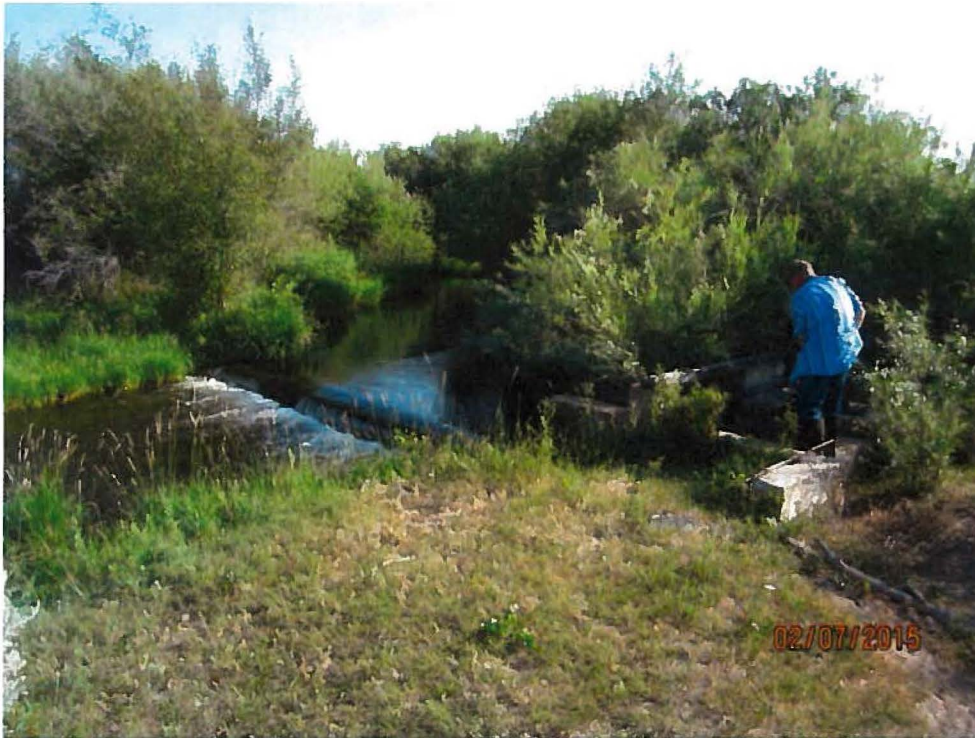
1. Turner 61: diversion dam across side channel of river, to open orifice-control box.
