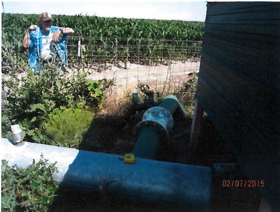
3. Ritter 66 Pump: dragon filter in foreground, 10" mainline and mag meter in background to pivots and hand lines.
