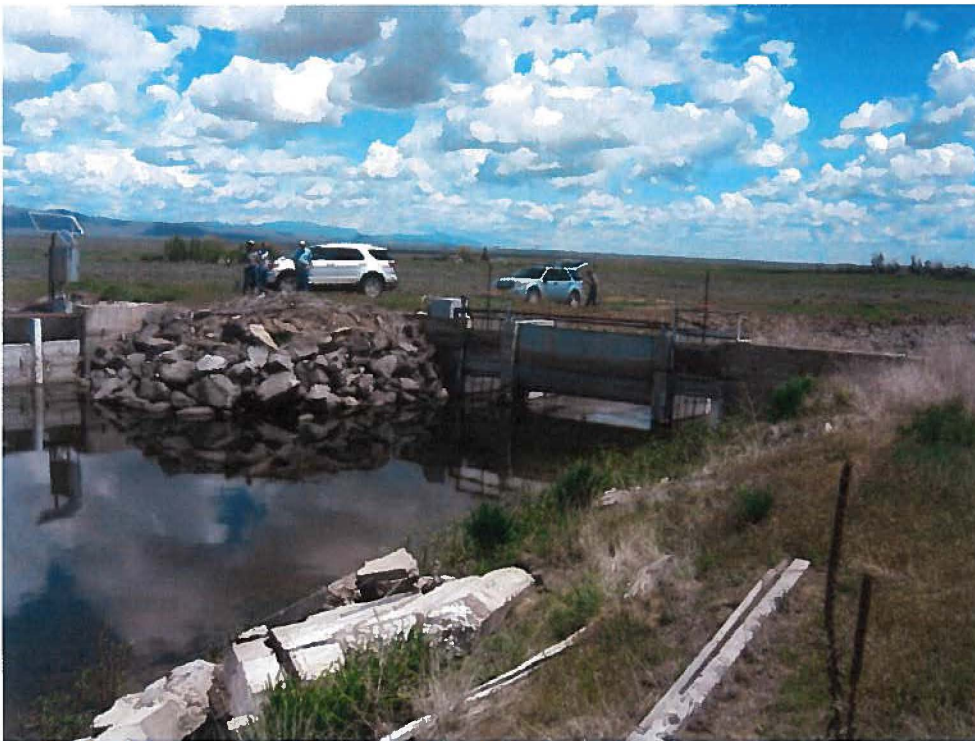
11. Richfield Canal split BWCC East and West Main Canals (head gate control structure on right), and Jim Byrns Slough (head gate control structure on left side of photo).
