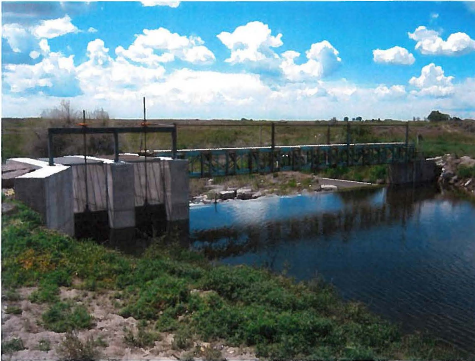
1. Diversion dam across Little Wood River about 120 ft west of Dietrich Main Canal. Two head gates are on east end (left of photo) for river control; one gate on west end for BLM ditch.
