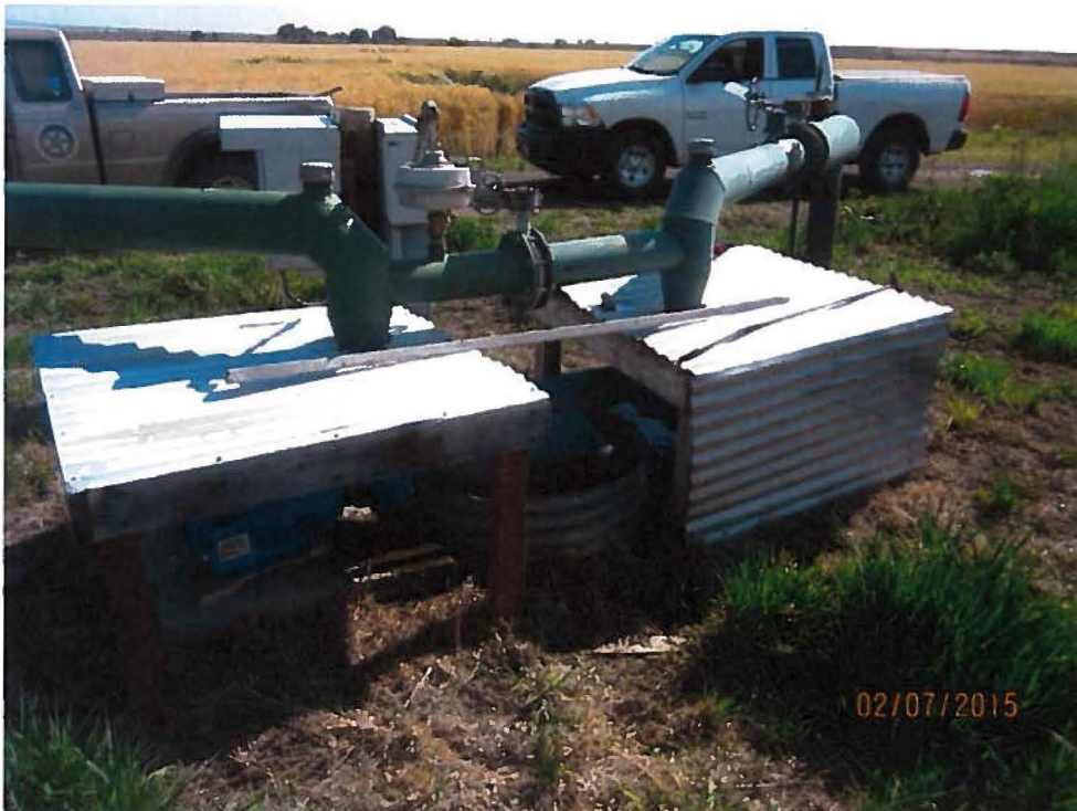
2. Hughes 63P - 64P pumps, CMP intake from river to two (2) centrifugal pumps. Pivot and grain crop in background.
