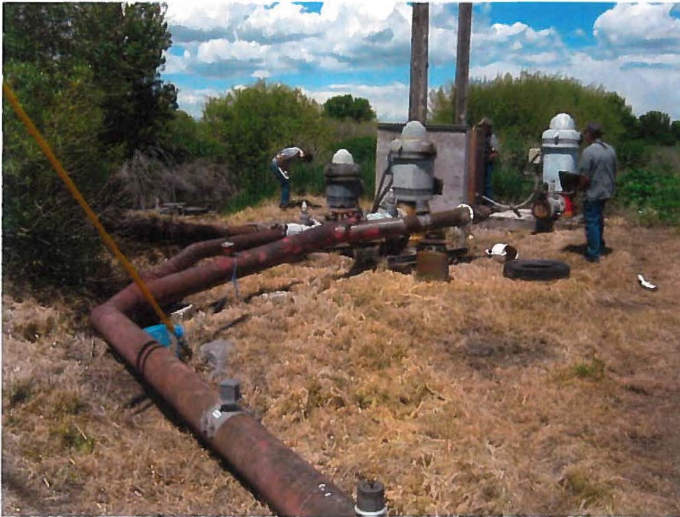
4. Taber 66-P: pump (left – 2 pumps visible from vault) and Taber ground water well (right) manifold into one common mainline to irrigation system discharge points. Note McCrometer meter in foreground on common mainline (measures both river and well water) and McCrometer meter in background on pipe from well.
