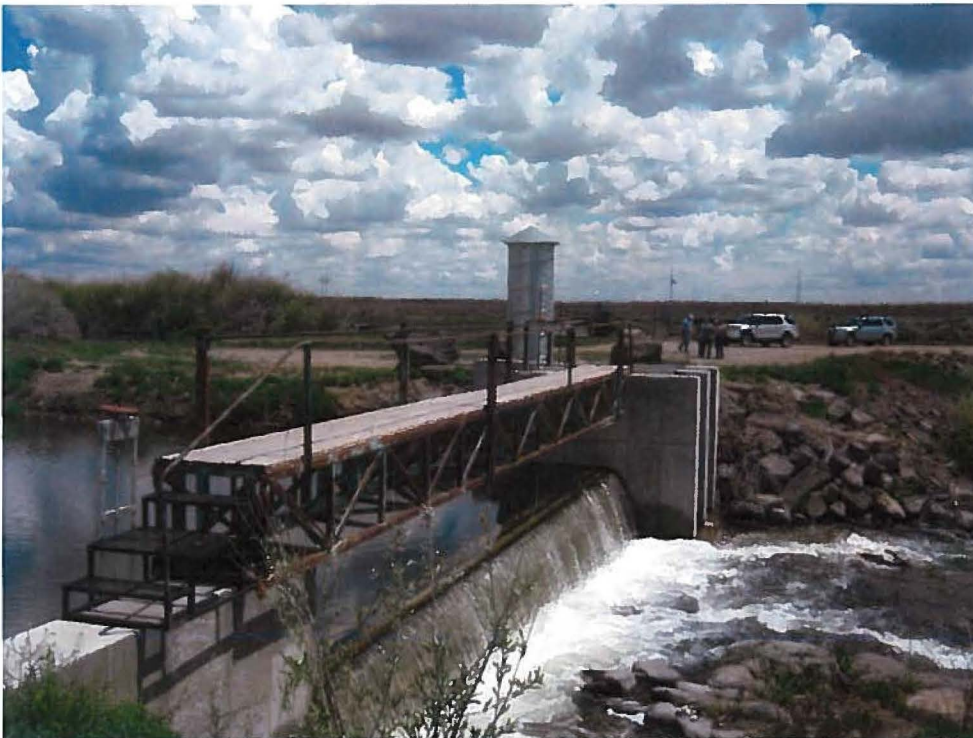
2. Diversion/Control structure across Little Wood River just west of the Dietrich Main Canal (view of structure from west river bank by BLM Ditch. Stilling well shed in background.
