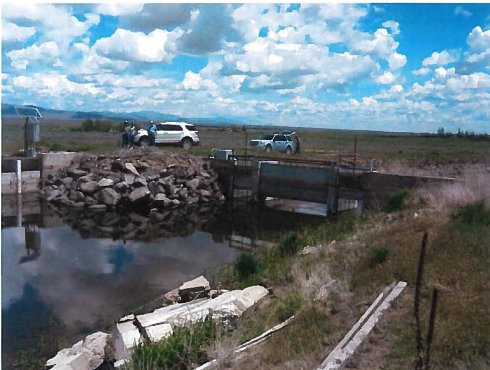
11. Richfield Canal split BWCC East and West Main Canals (head gate control structure on right), and Jim Byrns Slough (head gate control structure on left side of photo).
