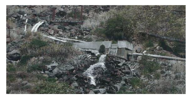
The mouth of the Martin-Curren Tunnel is shown in the upper left corner of this photograph with multiple white pipes coming from it. There is a concrete box at the mouth of the tunnel which the parties have referred to as the "Farmer's Box." The large concrete box in the center of this photograph is called the "Rangen Box."
