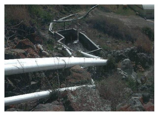
(<u>Exh</u>.1453) The concrete structure in this photograph is the Rangen Box shown from above. One of the white pipes from the Farmer's Box feeds water straight into the Rangen Box. The other white pipe diverts water onto the talus slope where it is then channeled downhill.
