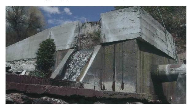
(Exh. 1456) Water can be diverted from the Rangen Box to the Small Raceways using the steel pipe that is coming out of the right side of the concrete structure. Alternatively, water can be allowed to go through the opening and then channeled downhill to a pond that supplies water to the Bridge Dam leading to the Large Raceways. (Tr., Vol VII, p. 1662, L. 25 – p. 1663, L. 6).
