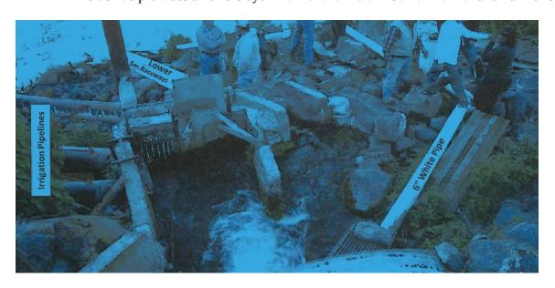
(Exh. 3278). The pipes labeled "Irrigation Pipelines" were used historically for farmer irrigation (e.g., Musser). The 6" White Pipe takes water to Rangen's Hatch House (where eggs and fry are raised), Rangen's Green House (where research is done) and to Rangen's Laboratory. The other two white pipes labeled "Small Raceways" and "Lower" take water further down the talus slope as shown in the next photograph:
