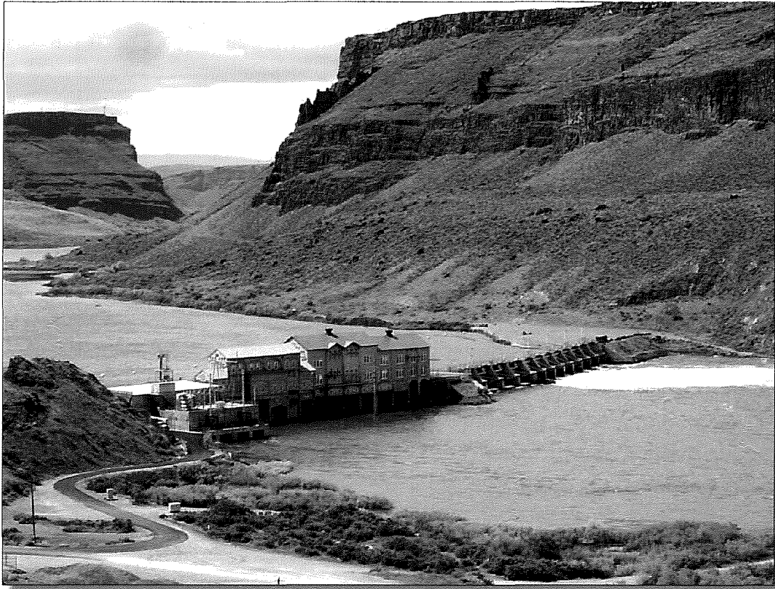
Photo: Swan Falls Dam ( photo by IDWR Dam Safety Program )
