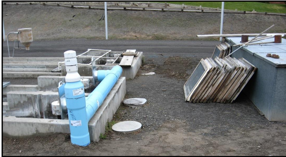
Photo 6. New 8-inch hatchery overflow pipeline at small raceways
