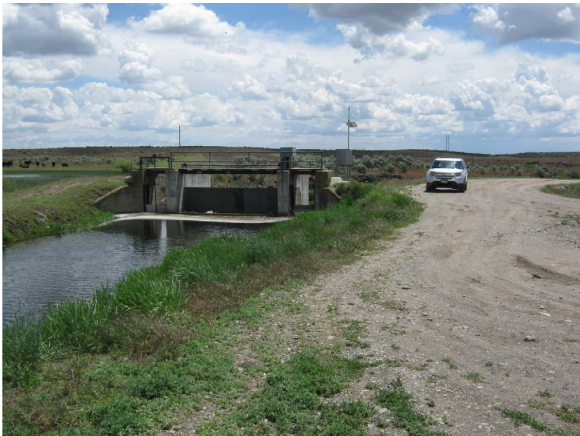
4. Dietrich Main Canal diversion and control structure with head gate controls (view is from confluence point of river and Jim Byrns Slough, river dam and control structure is off photo to right).
