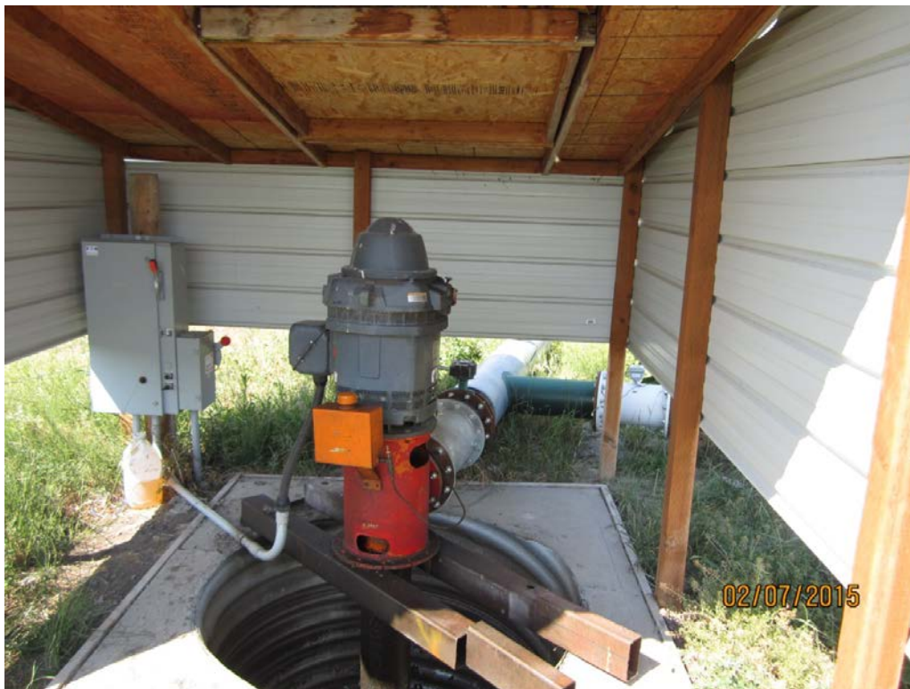
2. Ritter Pump 66: CMP well to vertical turbine 50 HP pump, connected to dragon filter (background, left) and mainline (right, with 10 inch Mag meter).
