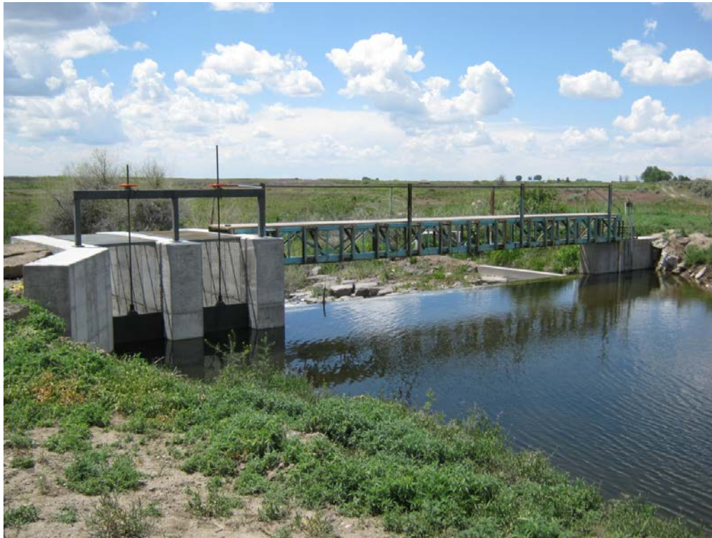
1. Diversion dam across Little Wood River about 120 ft west of Dietrich Main Canal. Two head gates are on east end (left of photo) for river control; one gate on west end for BLM ditch.
