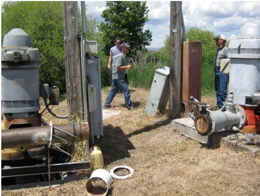
2. Taber Pump 66-P (left): 1 of 2 vertical turbine pumps from open concrete vault connected to river intake pump. Turbine motor pumps water to mainline that connects to mainline from ground water well on right.
