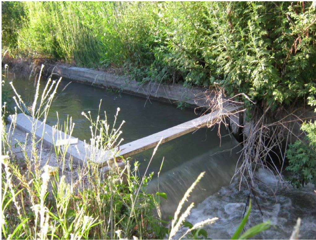
4. Slough Ditch 93: view of 5 ft rectangular weir from downstream.
