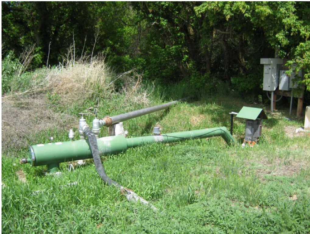
7. Meyers 75P: pond (not visible) in background to pump, mainline wit meter, filter and pressurized irrigation system including hand lines.
