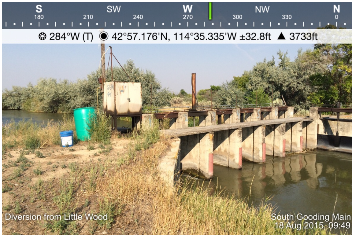
1. South Gooding Main: head gates used to divert water from the Little Wood River. The Little Wood River is not pictured but is off to the right.
