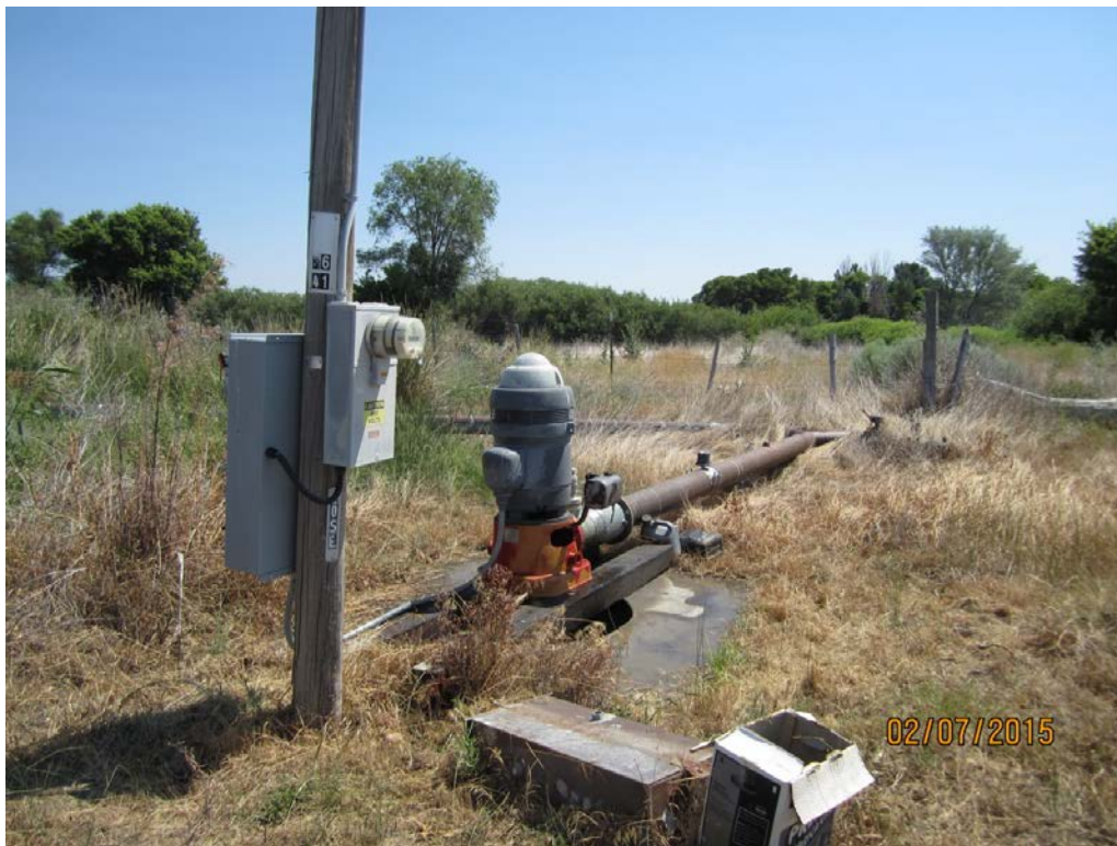
2. White Pump 66-P: 40 HP pump to 8 mainline with McCrometer flow meter, pipe tees to north and south mainlines.
