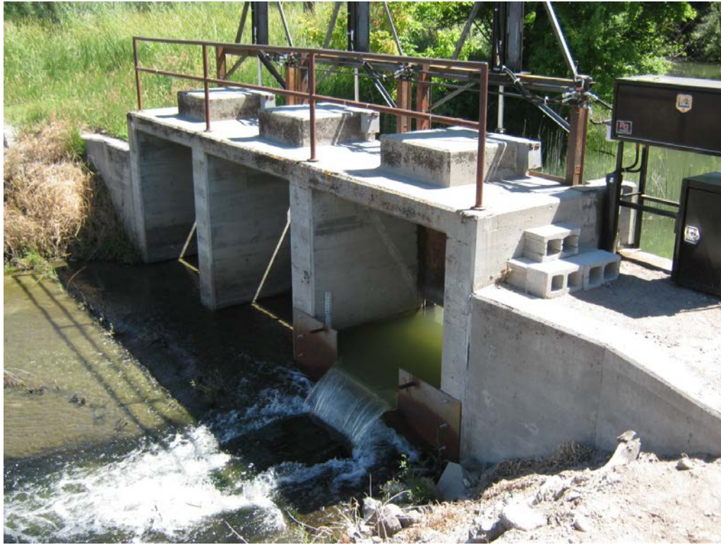
3. 3 ft rectangular contracted weir on south head gate bay.
