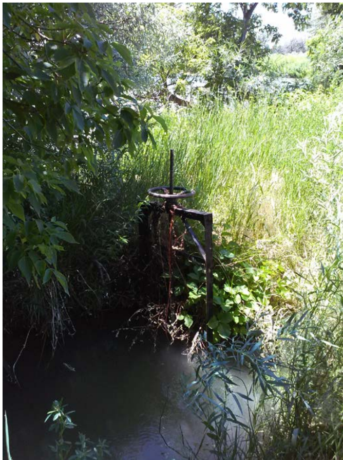
3. Hunter 79N: head gate on orifice-head gate control box.
