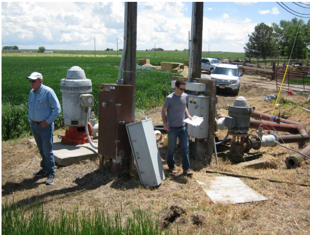
3. Taber 66-P: Pump on right (1 of 2 visible) with connected pipe that manifolds with pipe from ground water well (on left) to a common mainline that is buried to various irrigation sprinkler discharge points including a pivot, wheel lines and hand lines.
