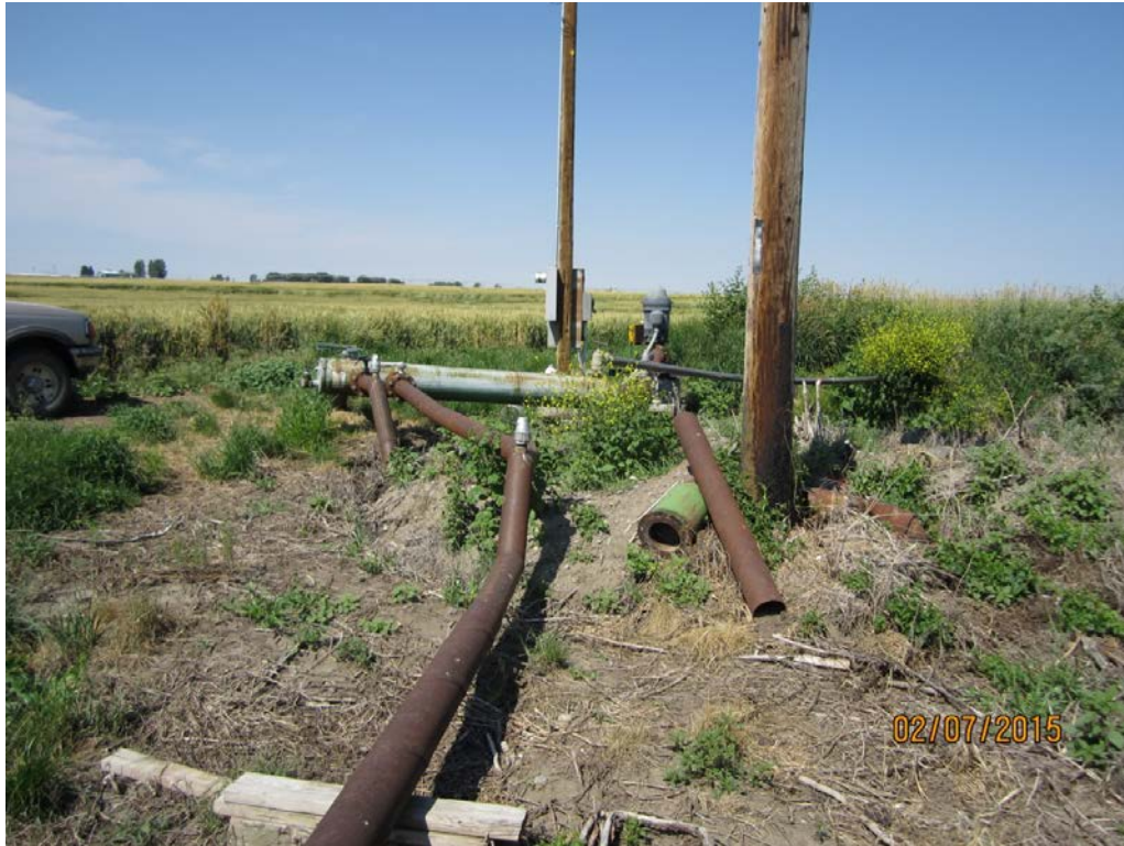
3. Taber 66-P1: Pump in background to mainline/dragon filter; three mainlines off dragon filter to irrigation sprinkler discharge points. Aluminum line off top of filter crosses river to north. Pivot (grain) behind pump.
