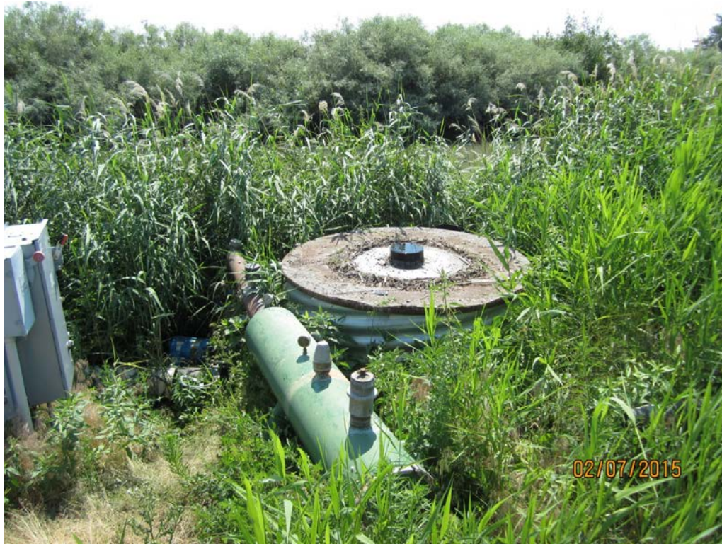
9. Meyers 75: one of two bubbler and re-lift pump systems.
