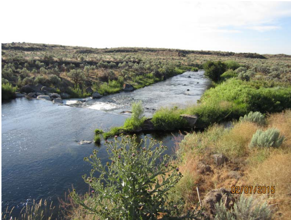
1. Appell 60: diversion dam across river, to open ditch and orifice-control box about 180 ft downstream.
