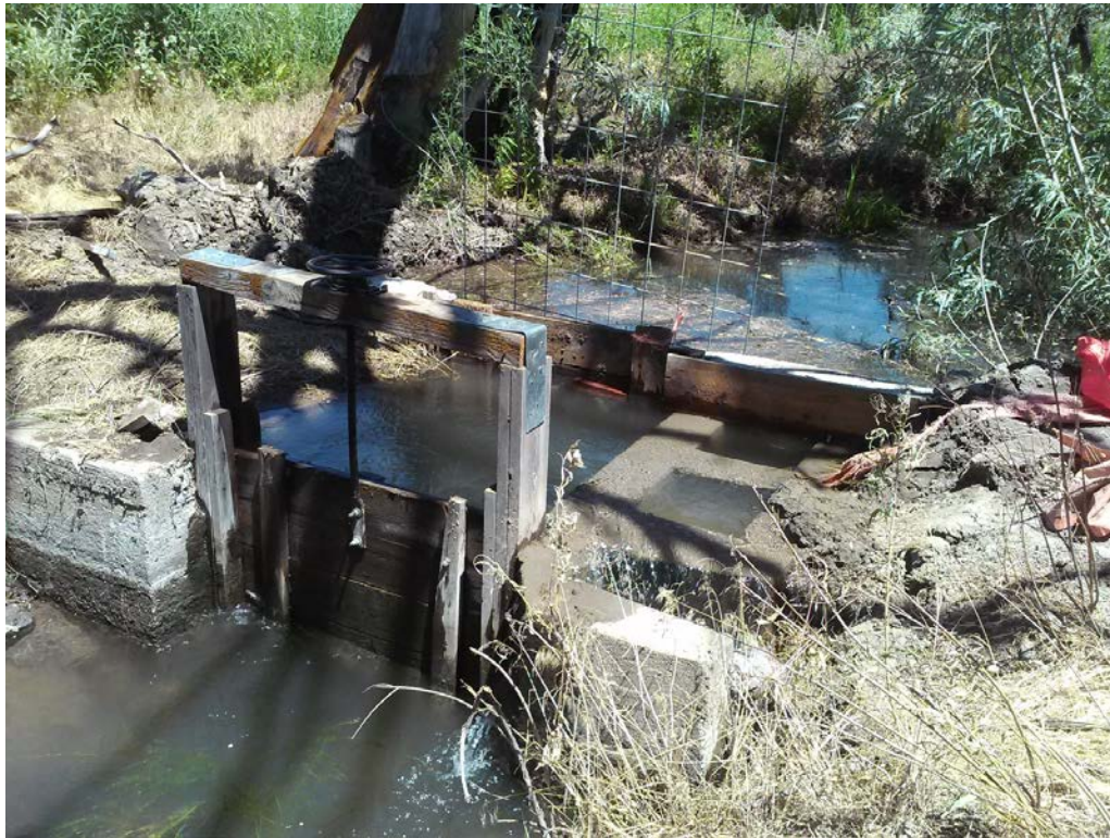
5. McFall Ditch 76S: orifice-gate box. Ditch was off at visit on 6/26/15 but river level high and leaking around and through box.
