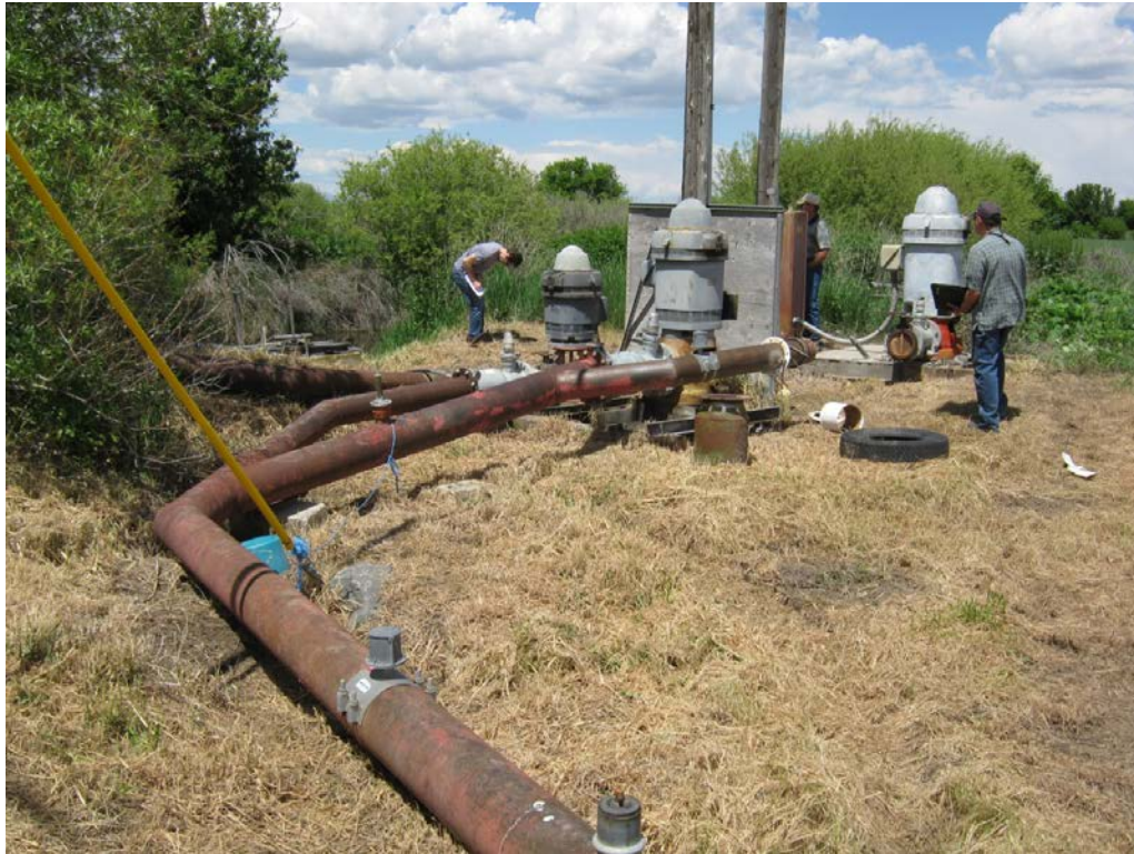
4. Taber 66-P: pump (left – 2 pumps visible from vault) and Taber ground water well (right) manifold into one common mainline to irrigation system discharge points. Note McCrometer meter in foreground on common mainline (measures both river and well water) and McCrometer meter in background on pipe from well.
