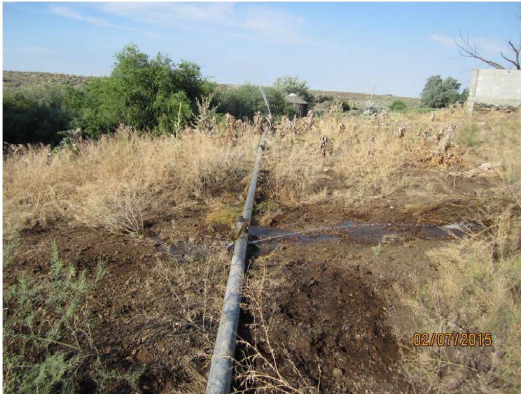
2. Kissler 60: Aluminum mainline with leaks.
