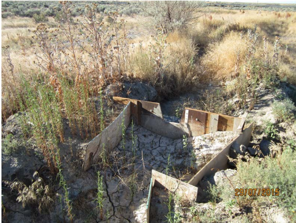
4. Stock 72: Weir in ditch below hydro power canal.
