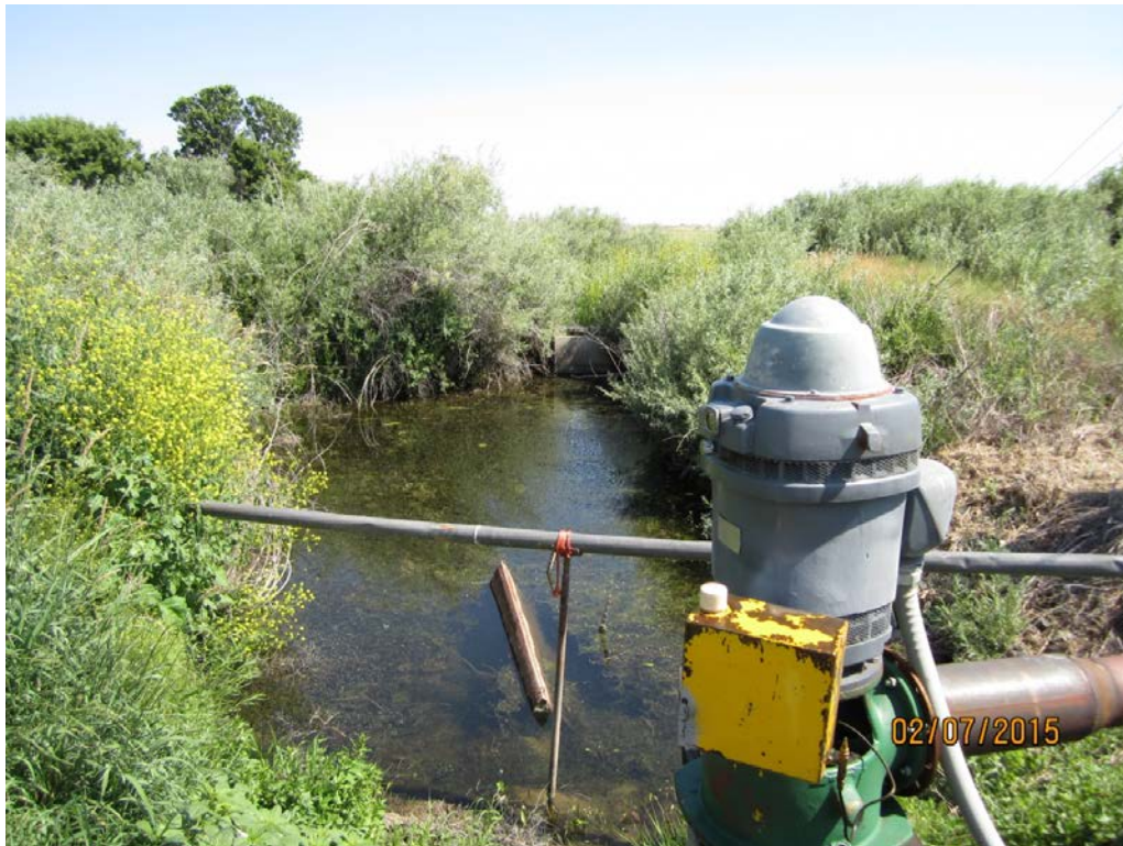
1. Taber Pump 66-P1: concrete diversion box in bank (background) diverts water to pond and pump intake.
