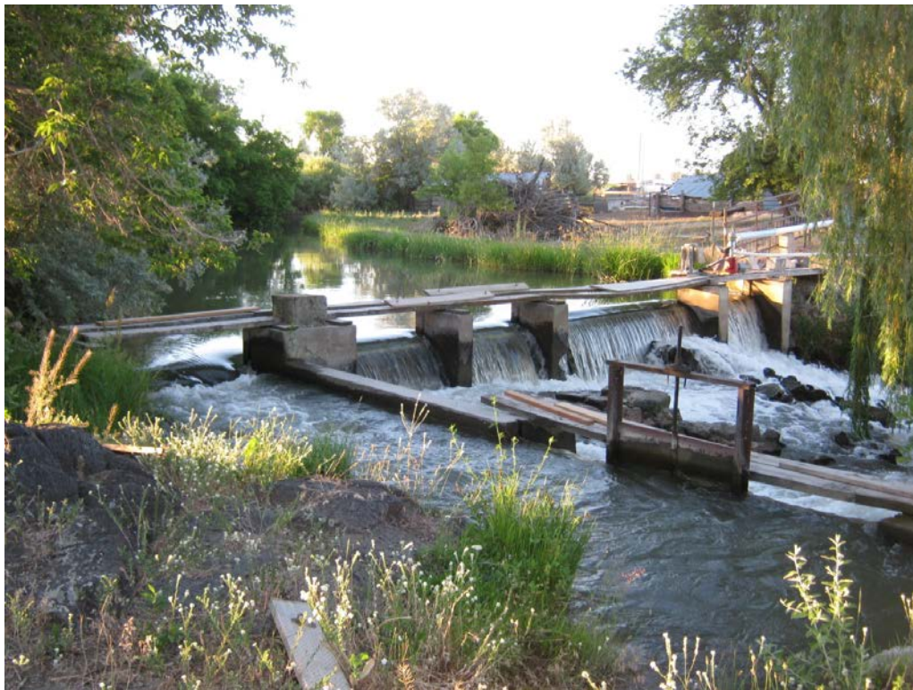
1. Slough Ditch 93: diversion/check dam across river; slide gate on right and stop logs control return flow to river.
