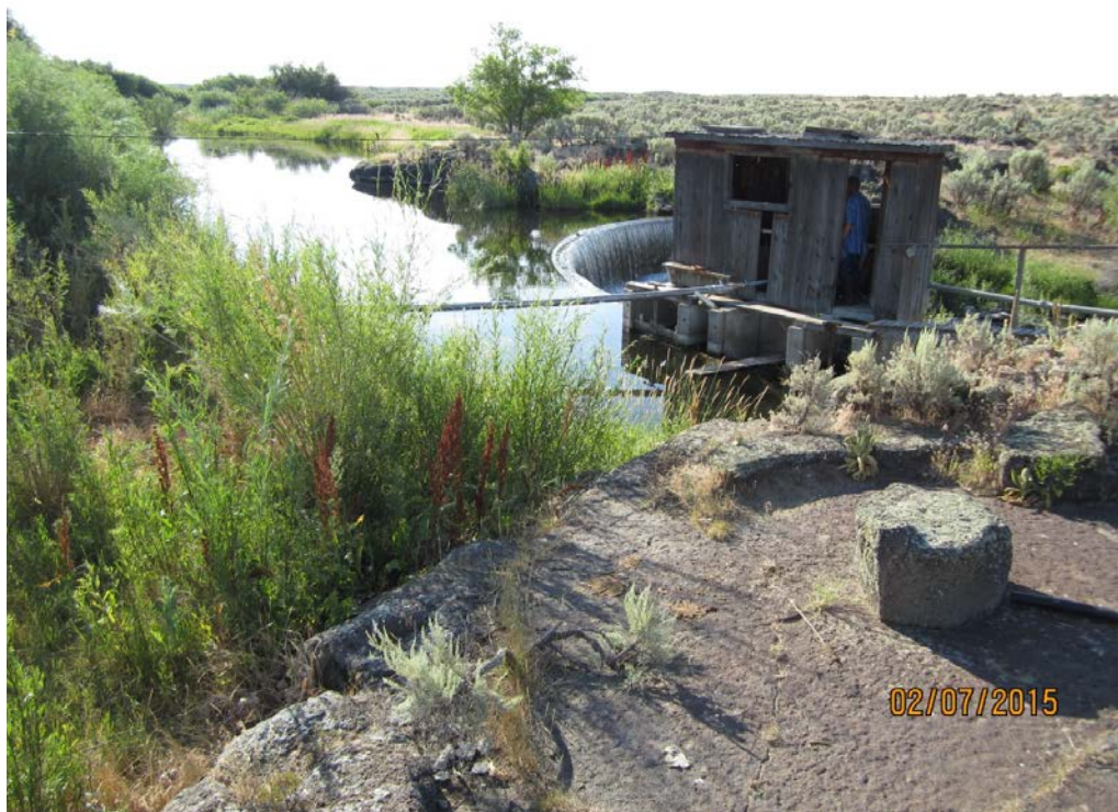
1. Kissler 60: Hydro dam across river to old power shed with 2 HP pump to 4 inch irrigation line.
