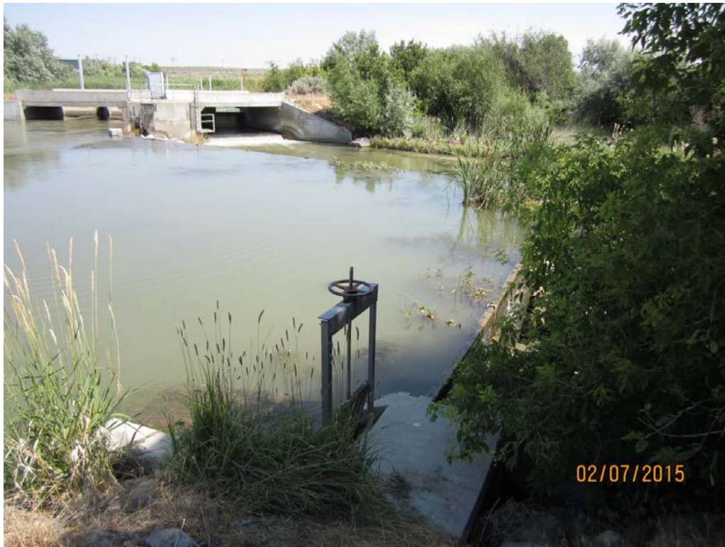
1. Meyers 73: diversion dam and control gate to ditch.
