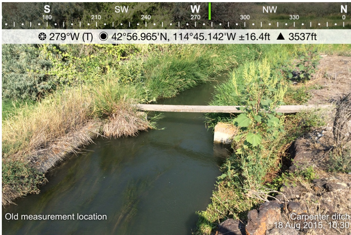
3. Looking down the Carpenter ditch, this was likely a location for a submerged orifice. On the left side in the grass are some stilling wells for measuring the water level above and below the orifice.
