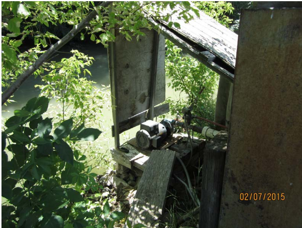
1. Rose 69-P7 pump: 7.5 HP centrifugal pump to 4 inch mainline.
