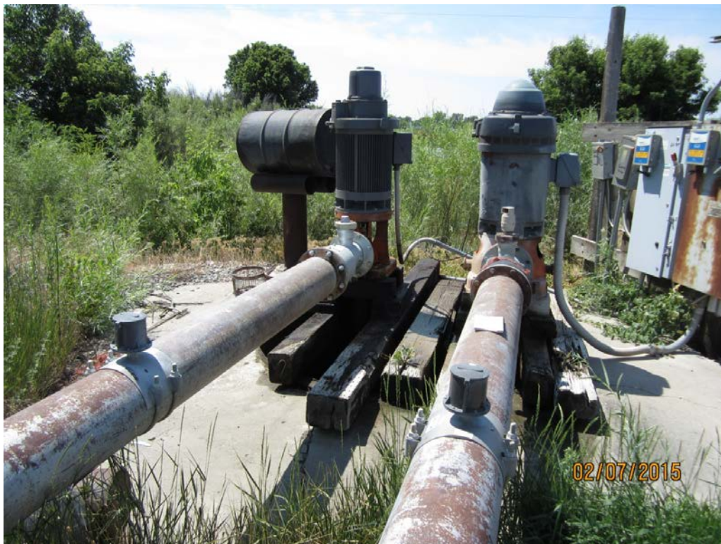
2. White Pumps 68 P1 & P2, 60 HP pump to 10 inch mainline with McCrometer flow meter (south or left of photo) and 100 HP pump to 10 inch mainline and McCrometer meter (north or right of photo).
