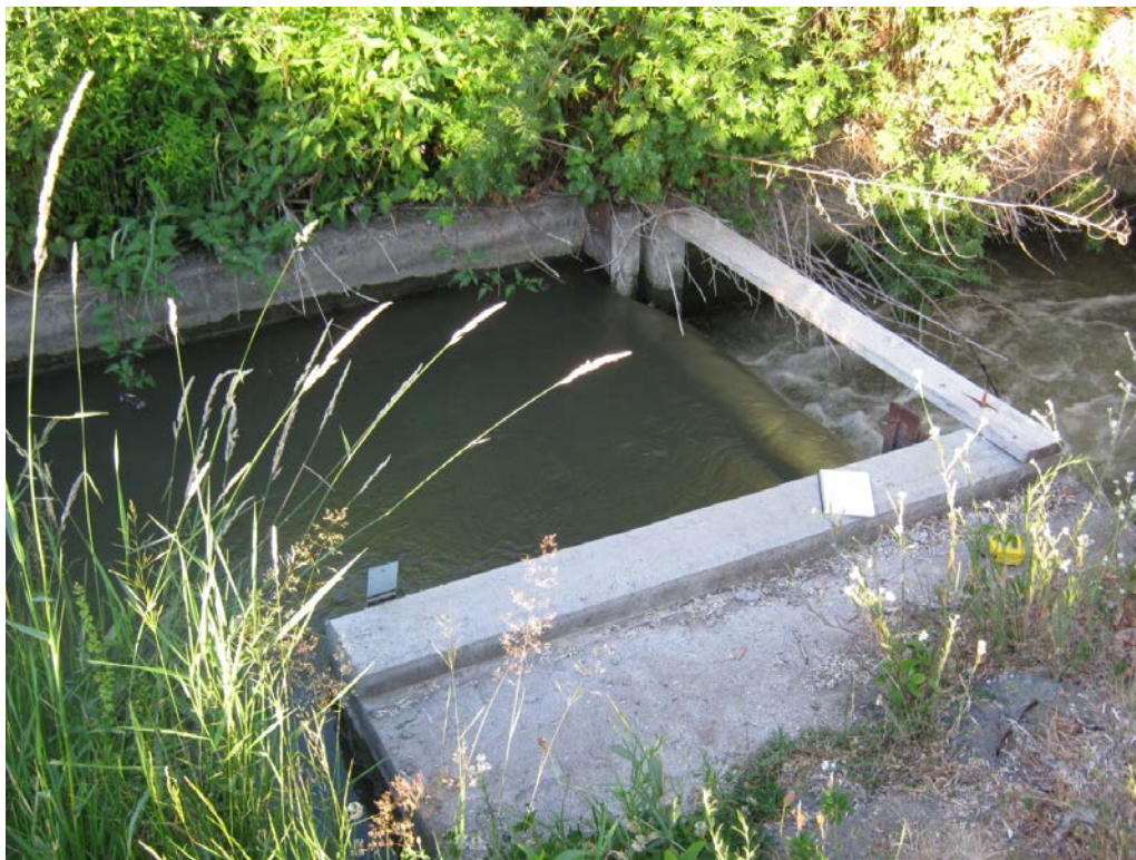
3. Slough Ditch 93: 5 ft rectangular weir in ditch about 30 ft below head gate.
