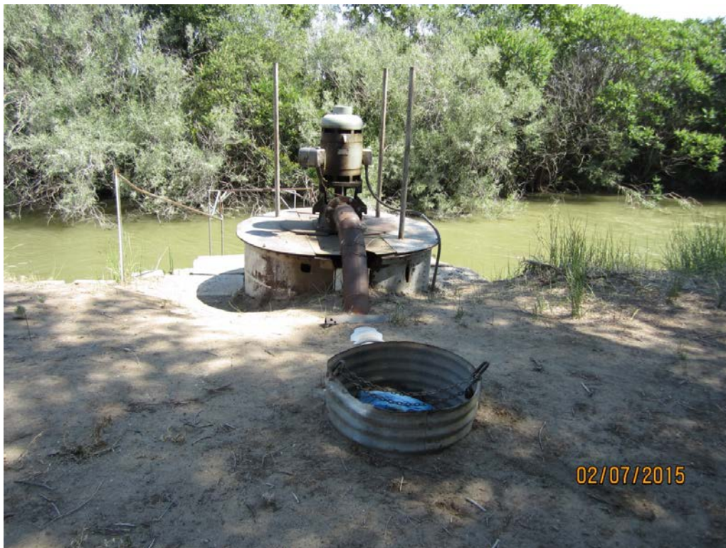
2. Shoshone City Pump 69-P2, steel vault/well with 15 HP pump to 8 steel mainline that transitions to 12 inch PVC pipe. CMP in foreground is exposed section of pipe with inoperable flow meter.
