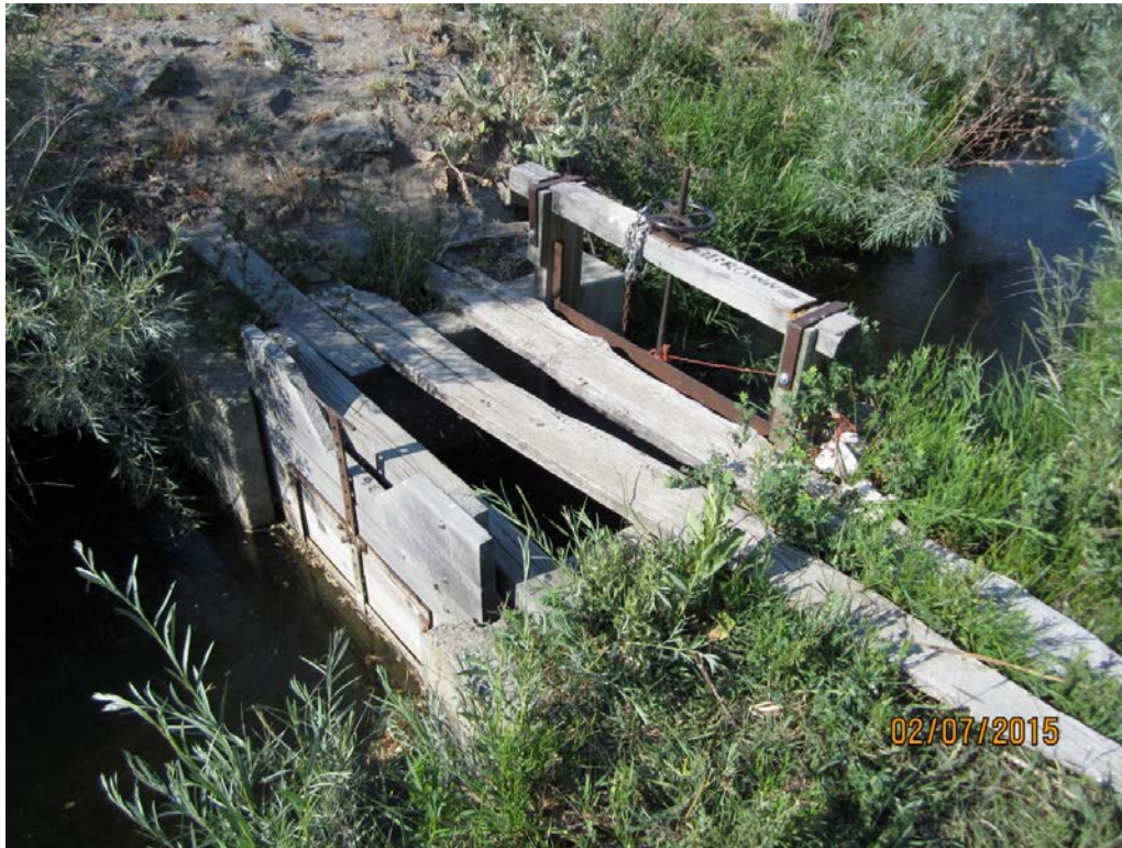
3. Brown 62: Submerged orifice and slide gate control box.
