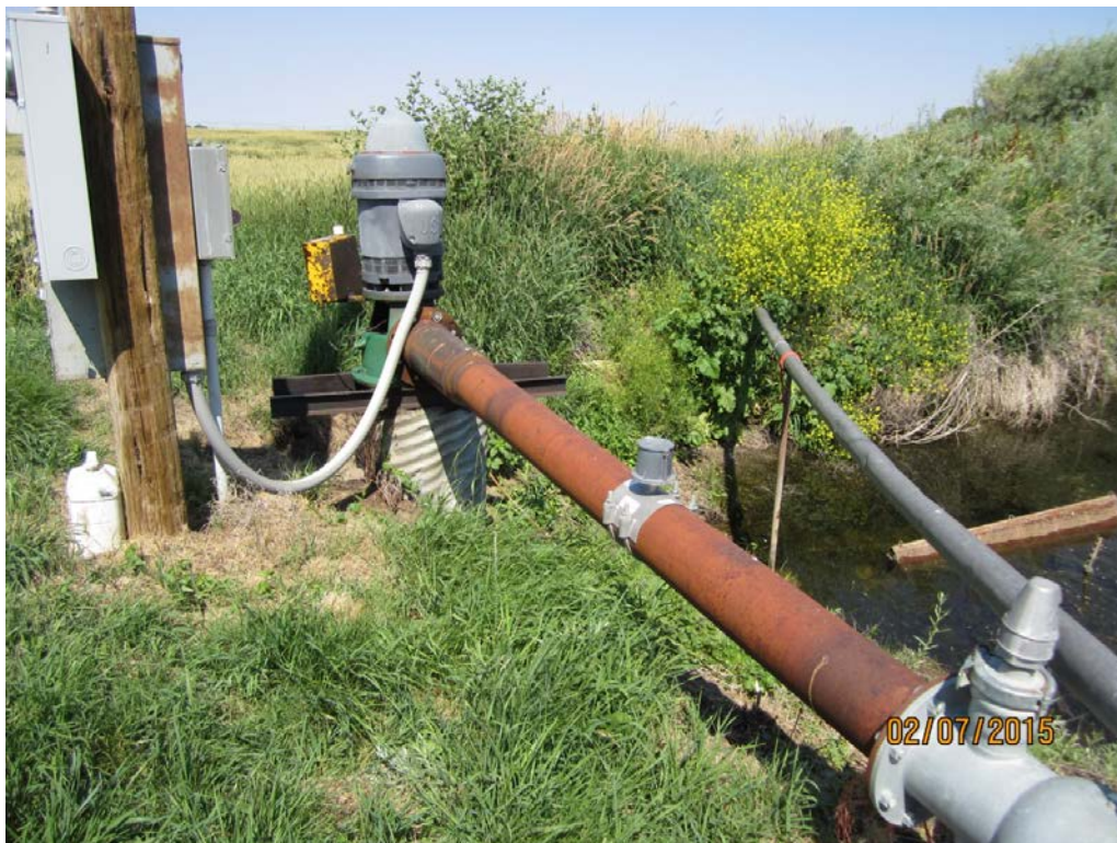
2. Taber Pump 66-P1: 75 HP pump to 8 mainline with McCrometer flow meter.
