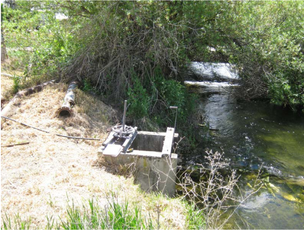
1. Taber Pump 66-P: intake pipe in river to old orifice-gate box connected to pump vault.
