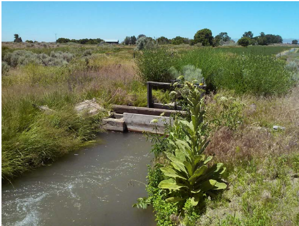
3. McFall Ditch 77N: View of orifice-gate box from check structures.
