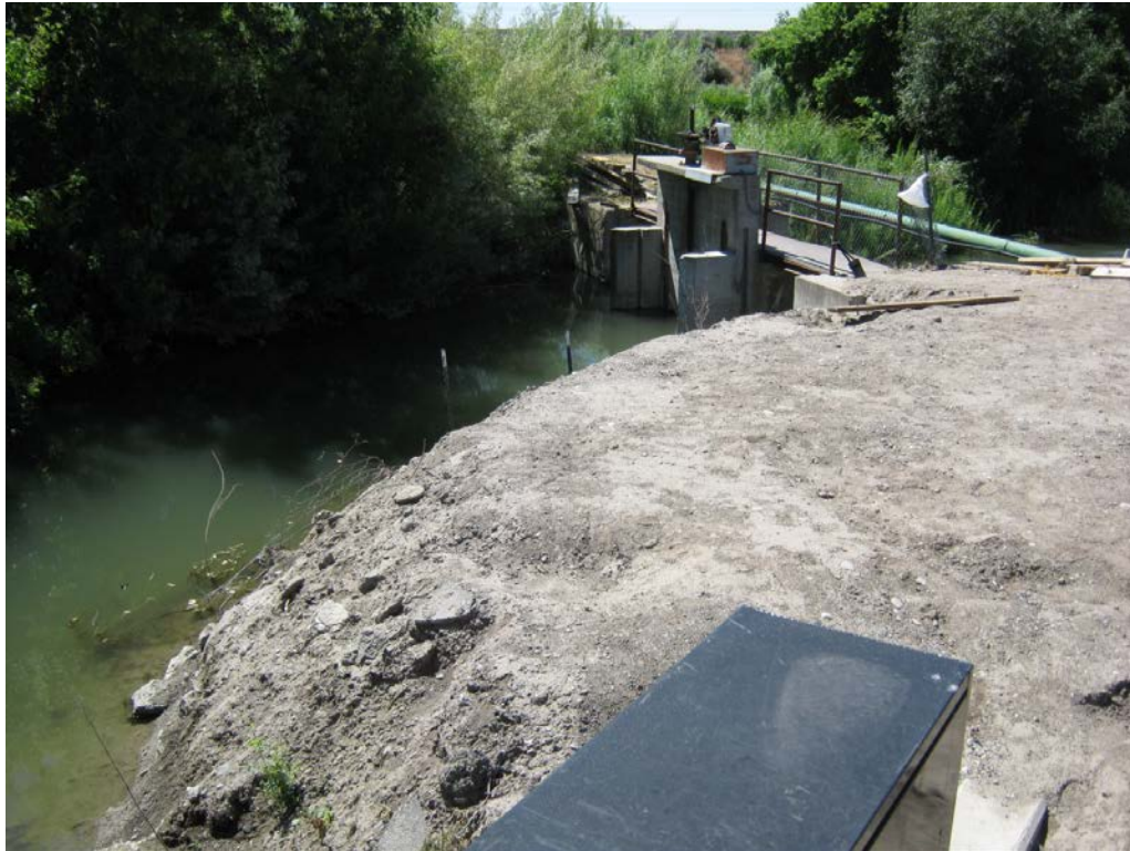
1. Diversion dam/check structure in river controls water to City head gate structure and ditch channel.
