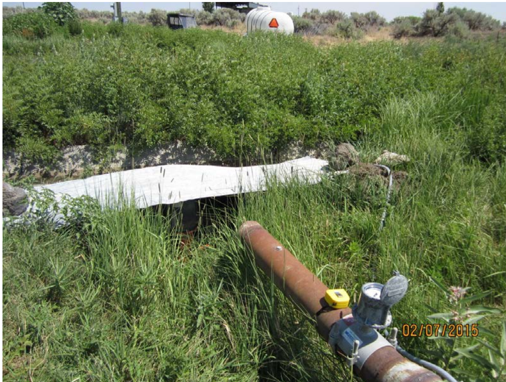
5. Meyers 74: re-lift pump to pivot and hand lines, pond in background (not visible), centrifugal pump in foreground under whit canopy, to mainline with Mcrometer meter.
