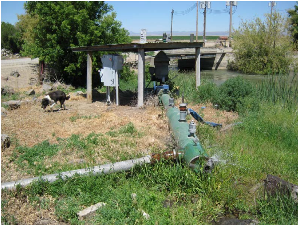
2. Winters 80-P pump: pump and river is in background, dragon filter with 6 inch aluminum mainline off filter going to corner area. Mainline to pivots comes off bottom of filter (buried)
