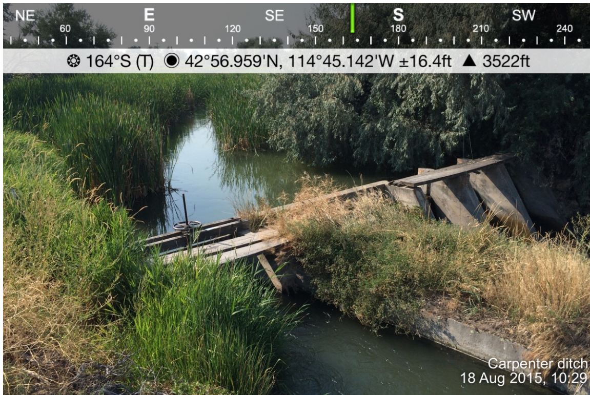
2. The upstream view, Little Wood River flows over the check boards on the right, the Carpenter ditch diversion is on the left.
