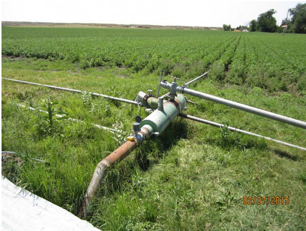
6. Meyers 74: re-lift pump to corner hand lines and pivot (to left of photo)
