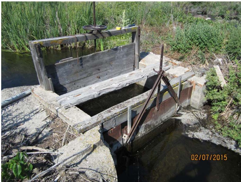
2. Ritter Ditch 65 orifice gate control box.
