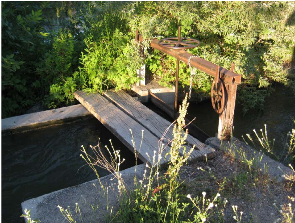
2. Slough Ditch 93: control structure and head gate controls flow to ditch.
