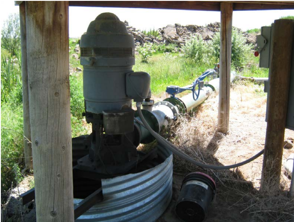
1. Winters 80-P pump: CMP wet well/sump with 50 HP pump to 10 inch mainline with flow meter.
