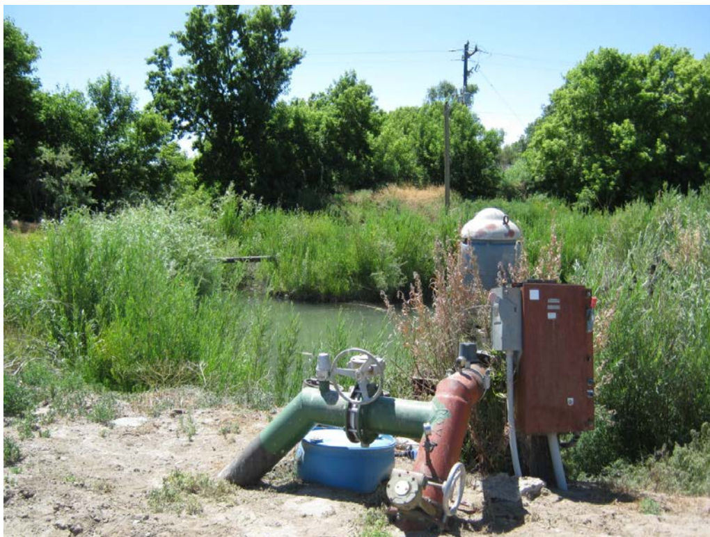
4. Devaney 86 West pump and mainlines from pump. Note diversion pond in background and pipeline from east pump crossing edge of pond in left-center part of photo.
