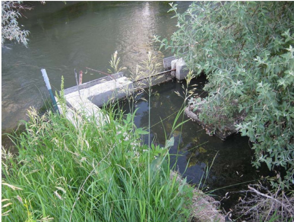
1. Kuntz 98-P2W: diversion box in river to intake pipe and discharge pump (30 HP).
