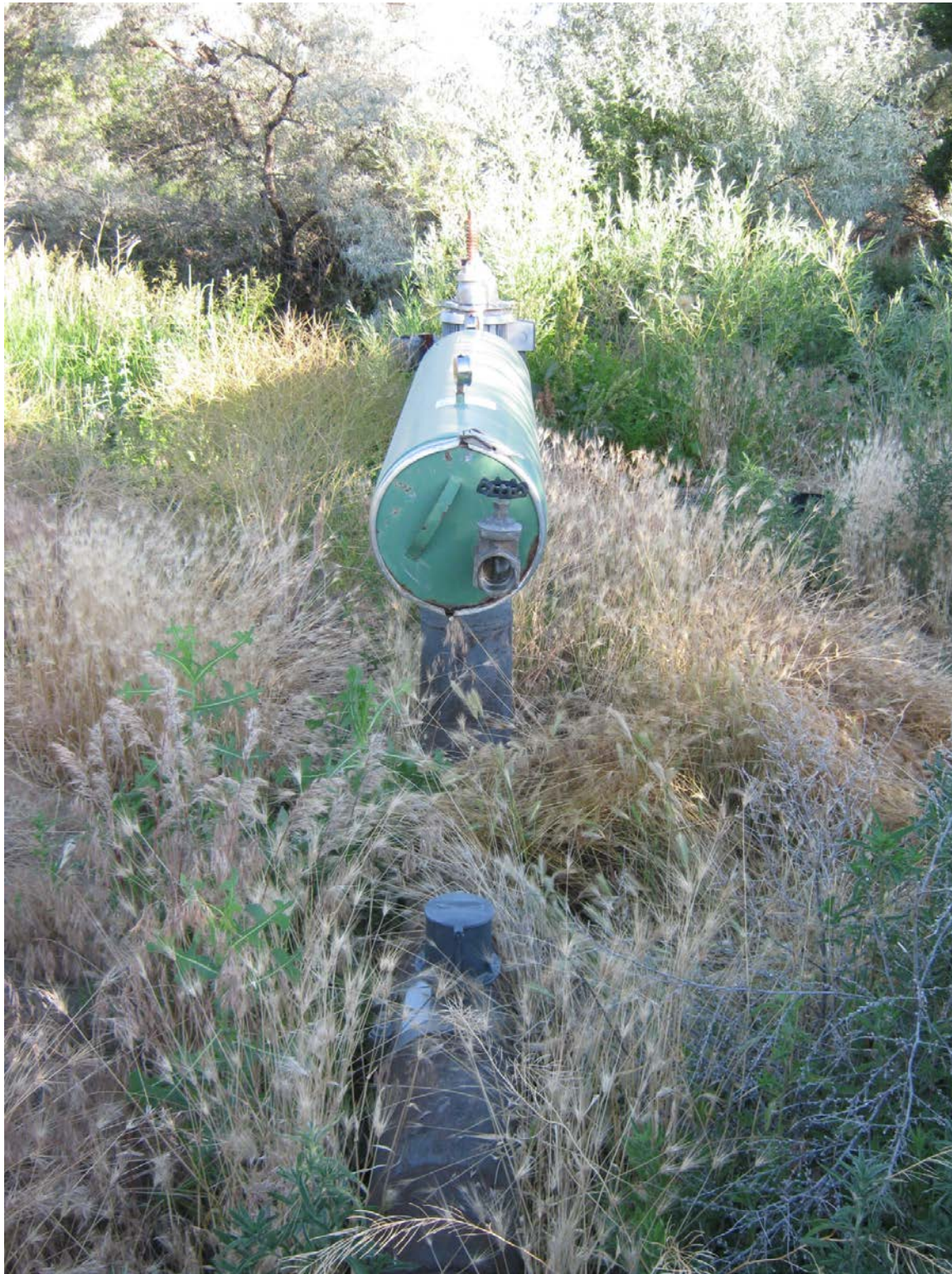
2. Kuntz 98 P2W: view of pump, dragon filter and flow meter on line off filter (foreground)
