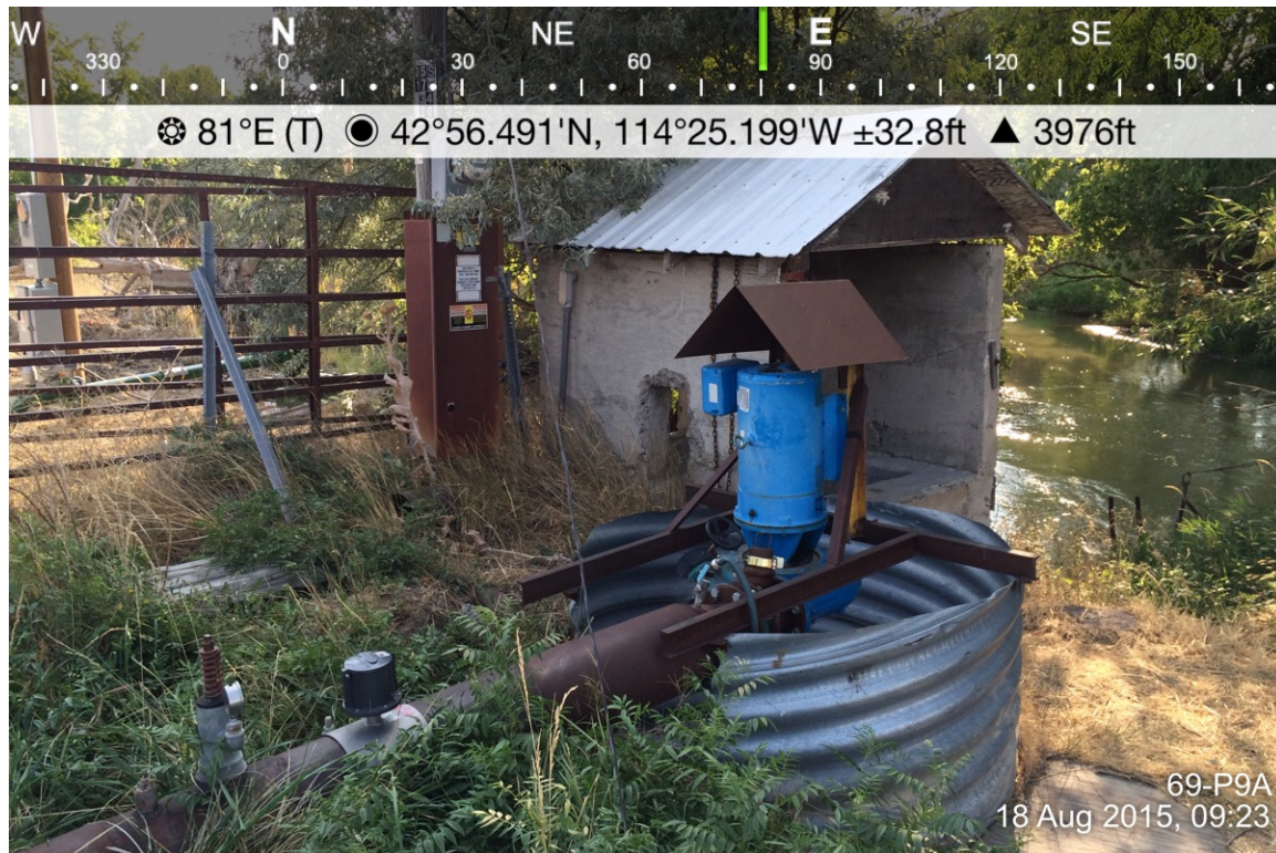
1. Uhrig pump 69-P9A: CMP well to vertical turbine 30 HP pump, and mainline with 10 inch McCrometer meter.
