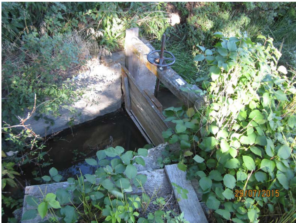
5. Stock 71A: Control gate downstream of ditch heading off river, a return flow gate to left (not shown) can spill water back to the river.
