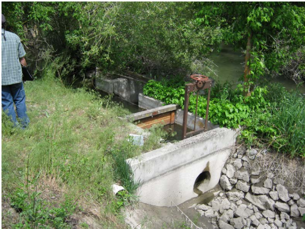
8. Meyers 75: Open ditch/channel from river to diversion check structure with stop logs for spill to river or diversion to orifice-gate box in foreground, then to open ditch and irrigation systems.
