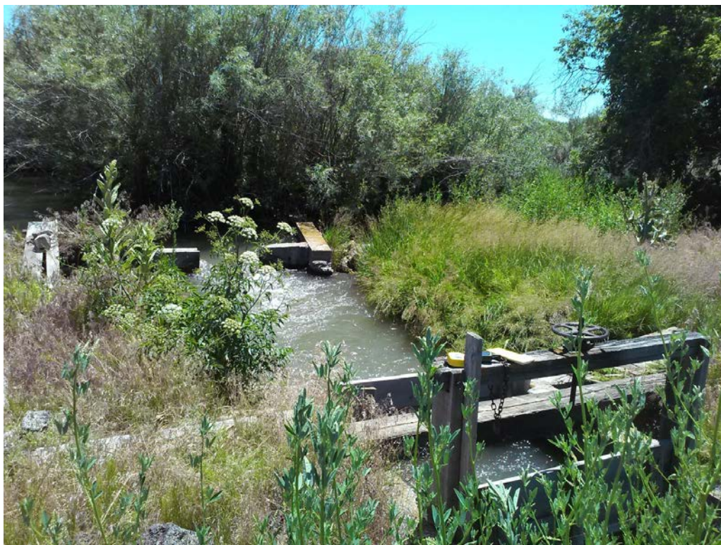
2. McFall Ditch 77N: Check dam in background, orifice-gate box in foreground.
