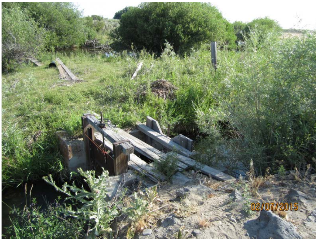
2. Brown 62: orifice-head gate control box, open ditch downstream of box to bubbler and gated pipe.
