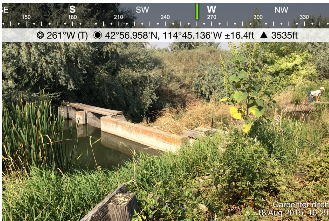
1. The Little Wood River flows over the check boards on the left, the Carpenter ditch diversion is on the right.
