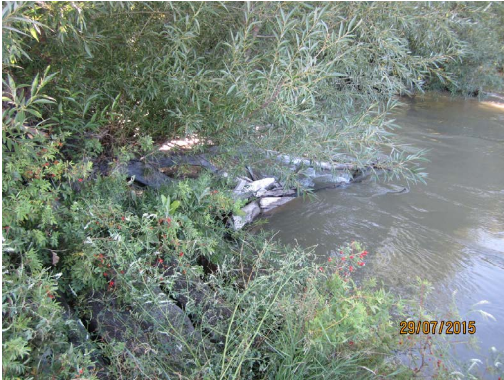
1. Stock 71: Rock and log wing dam in river checks water to ditch and orifice-control gate.
