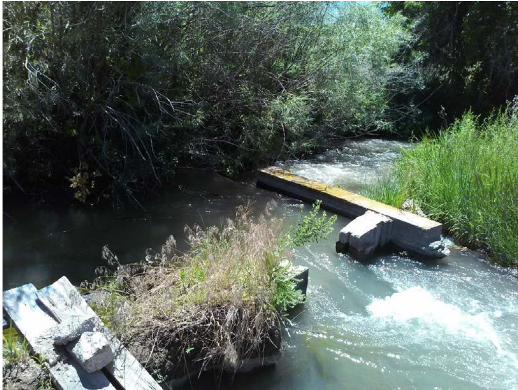
1. McFall Ditch 77N diversion and check dams on side channel of river to head of ditch.
