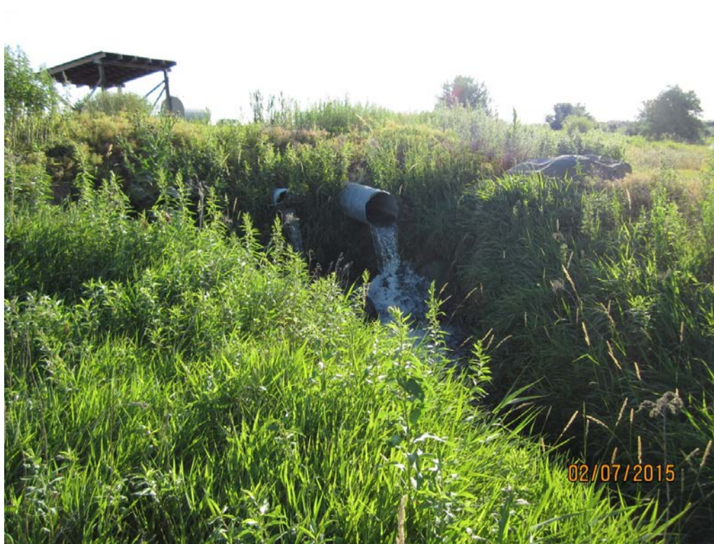
4. Appell 60: ditch return flow/spill back to river, pump in background.
