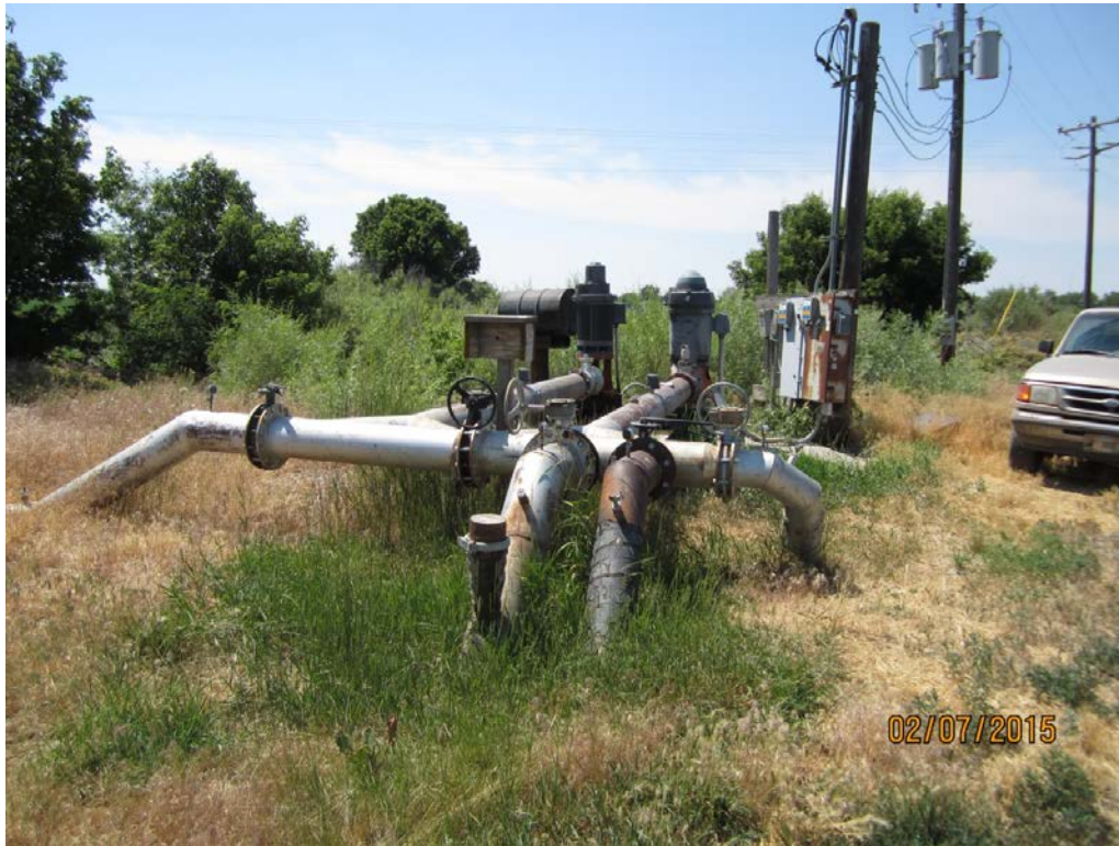
3. White 68 P1 and P2, pumps to mainlines, manifold; 4 lines off of manifold to pressurized sprinkler systems.
