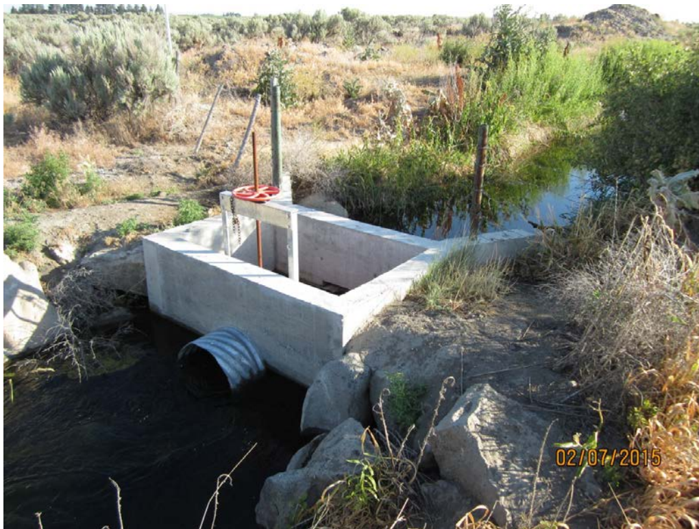
2. Appell 60: orifice-head gate control box.
