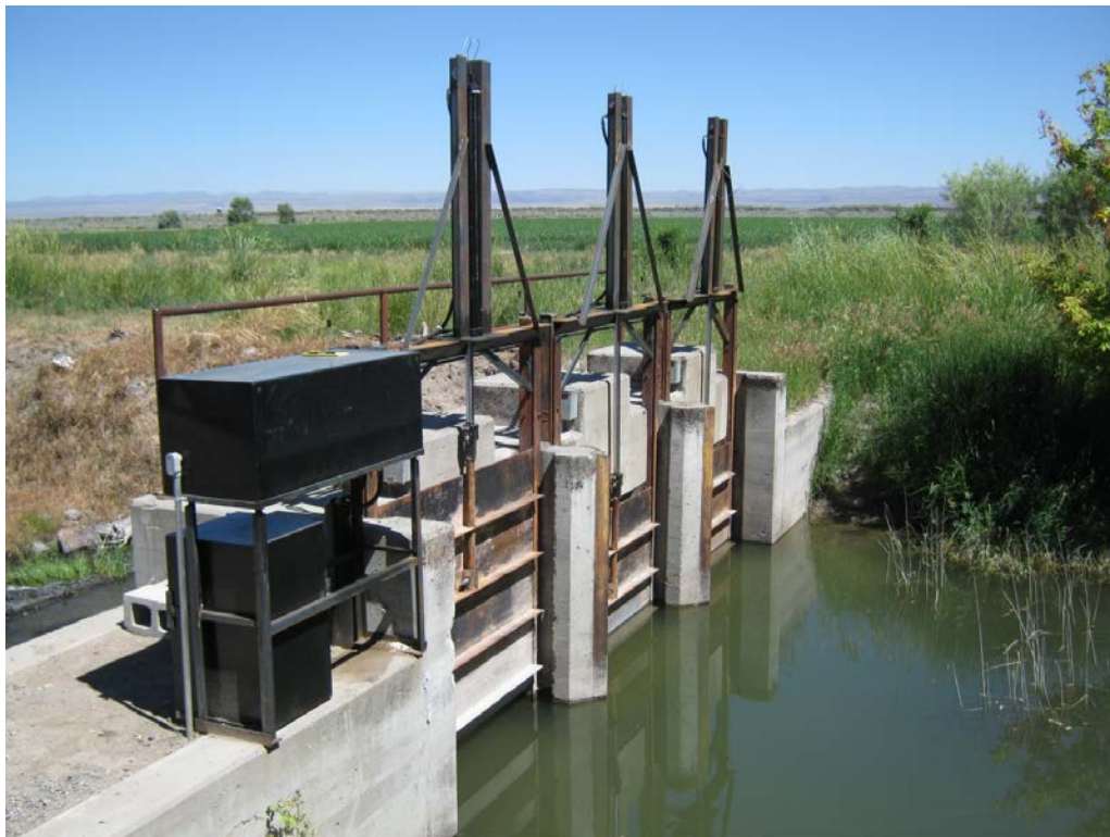
2. Head gate control structure with 3 steel automated slide gates for control.
