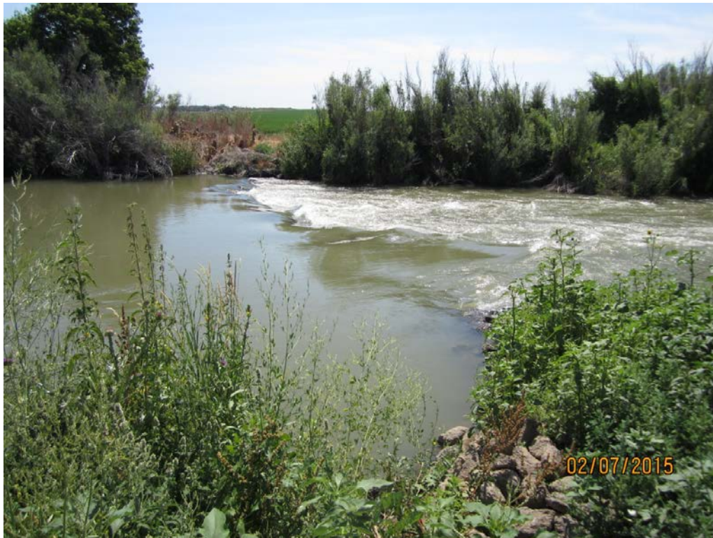
1. Rock weir dam in river raises water to cut in north side of river bank to small pond and pump station.
