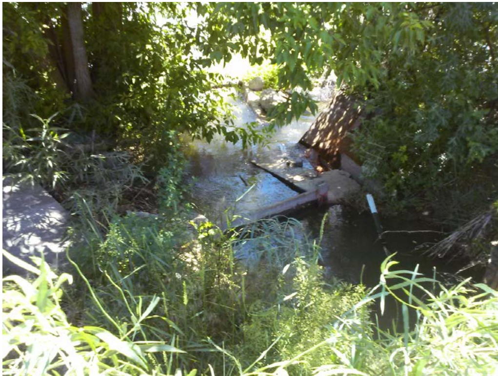
2. Hunter 79N Ditch: orifice-head gate control box at head of ditch off river. Wooden submerged orifice on box entrance.
