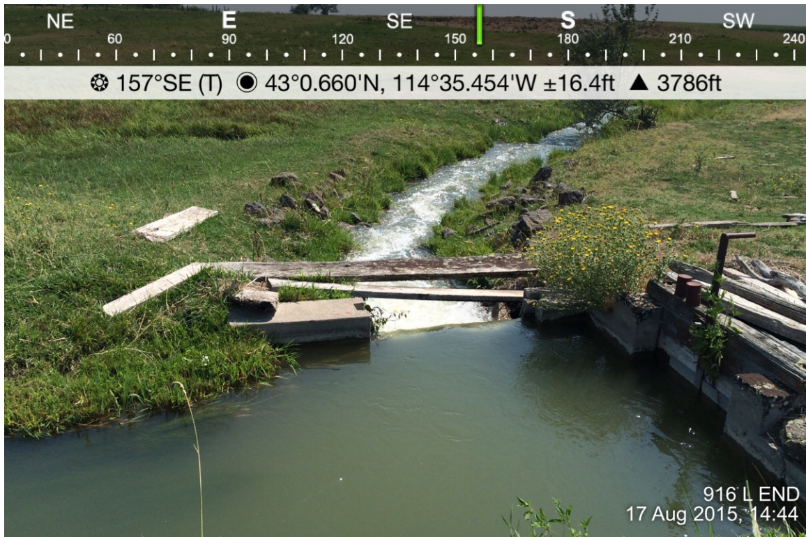
1. 916L End diversion and weir.
