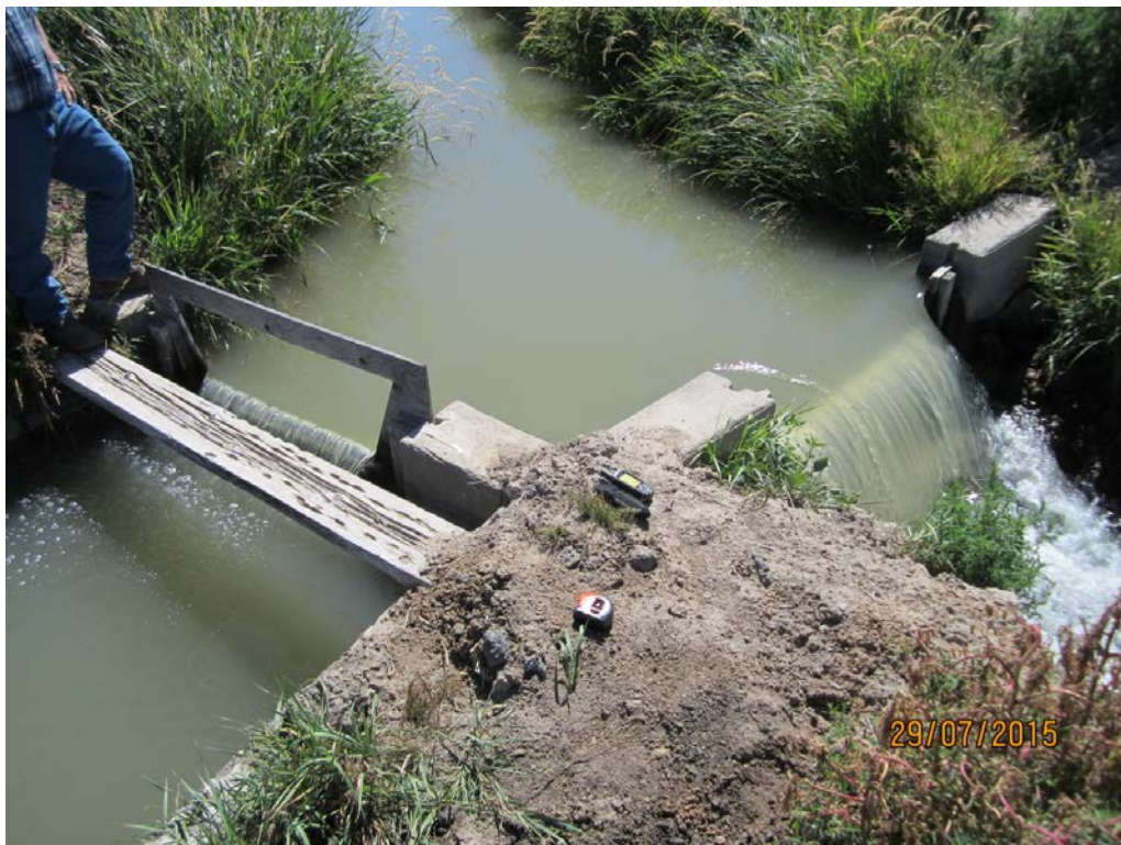
4. Split at end of Robertson Ditch to Sabala Farms (right hand side of photo) and other ditch user (left). Sabala control and measurement is a 4' Cipolletti weir in the concrete check structure.
