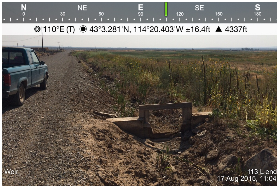
2. 113L: End weir, looking down stream
