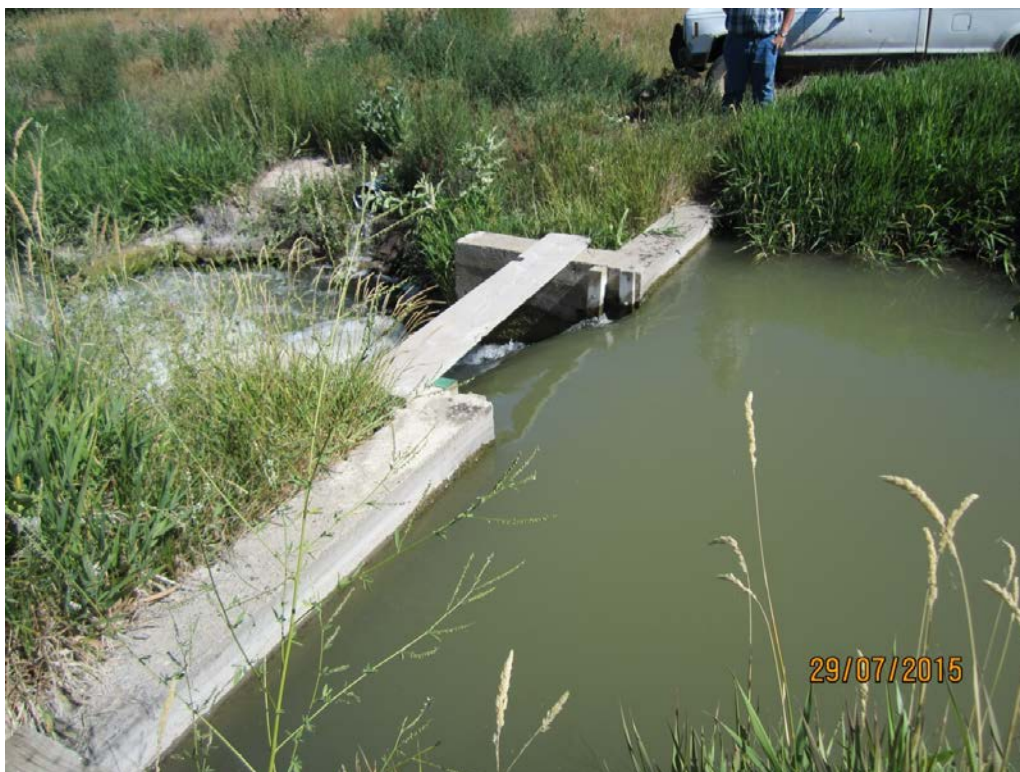
6. View of check structure used as weir from L2 head gate.
