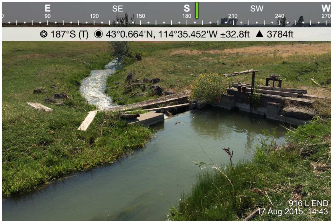
2. 916L End diversion: head gate off to the right is not a working diversion.
