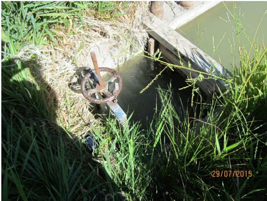
3. Union Ditch – L2 head gate and re-diversion for 4 Brothers right 37-11114B. Orifice gate box with submerged orifice (in box at top) and lateral gate with hand wheel control.
