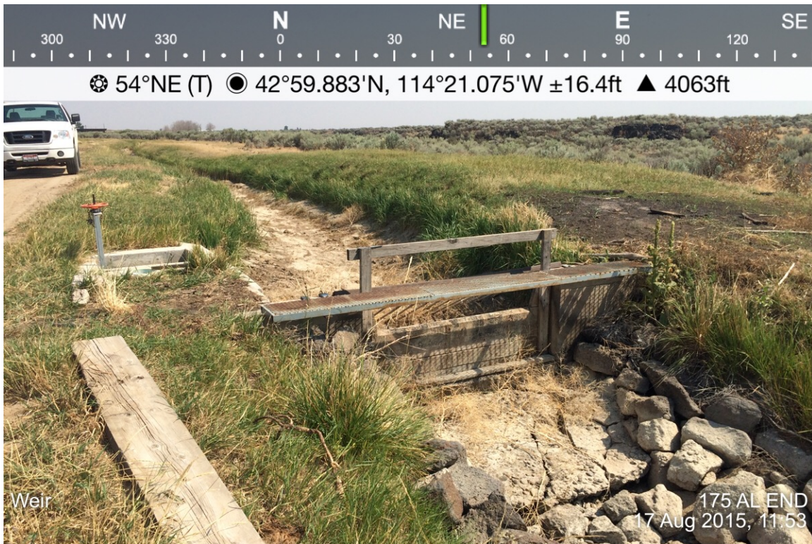
2. Upstream view of 175AL End weir blade.
