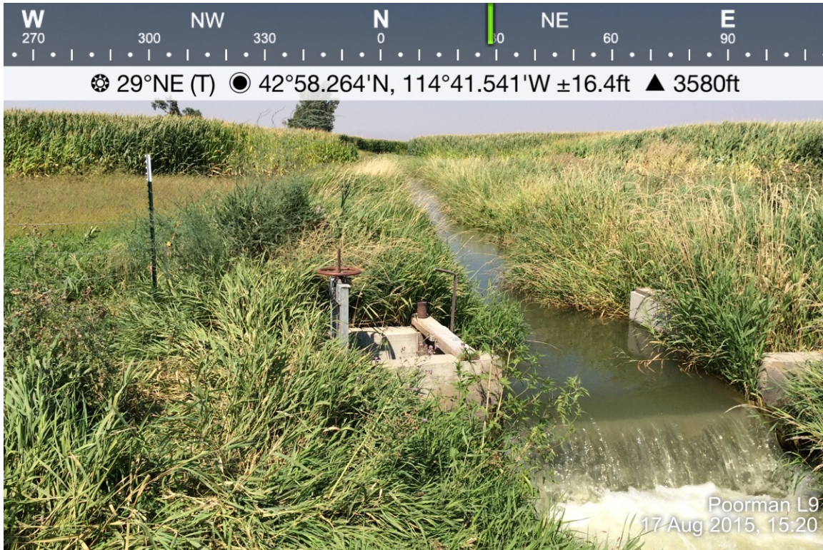
1. Head gate in the center of the picture is the Poorman L9 diversion.
