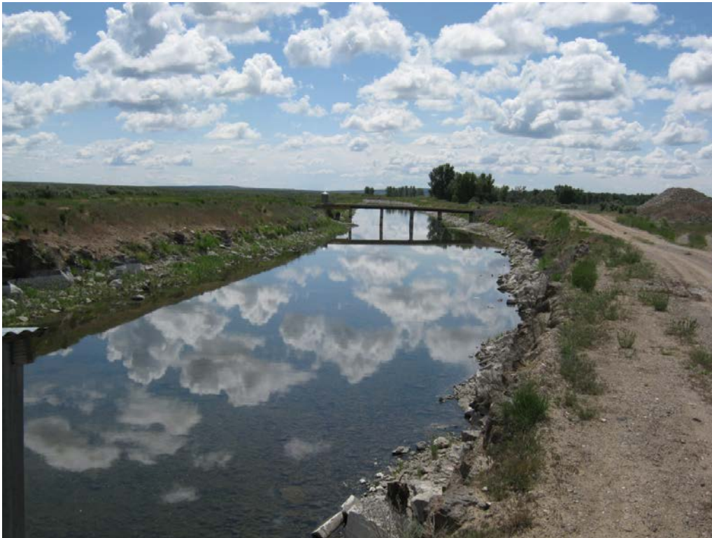
7. View of Richfield Canal looking downstream from spill gates. Rated measurement section in canal at center of photo, about 150 yards downstream from spill gates.
