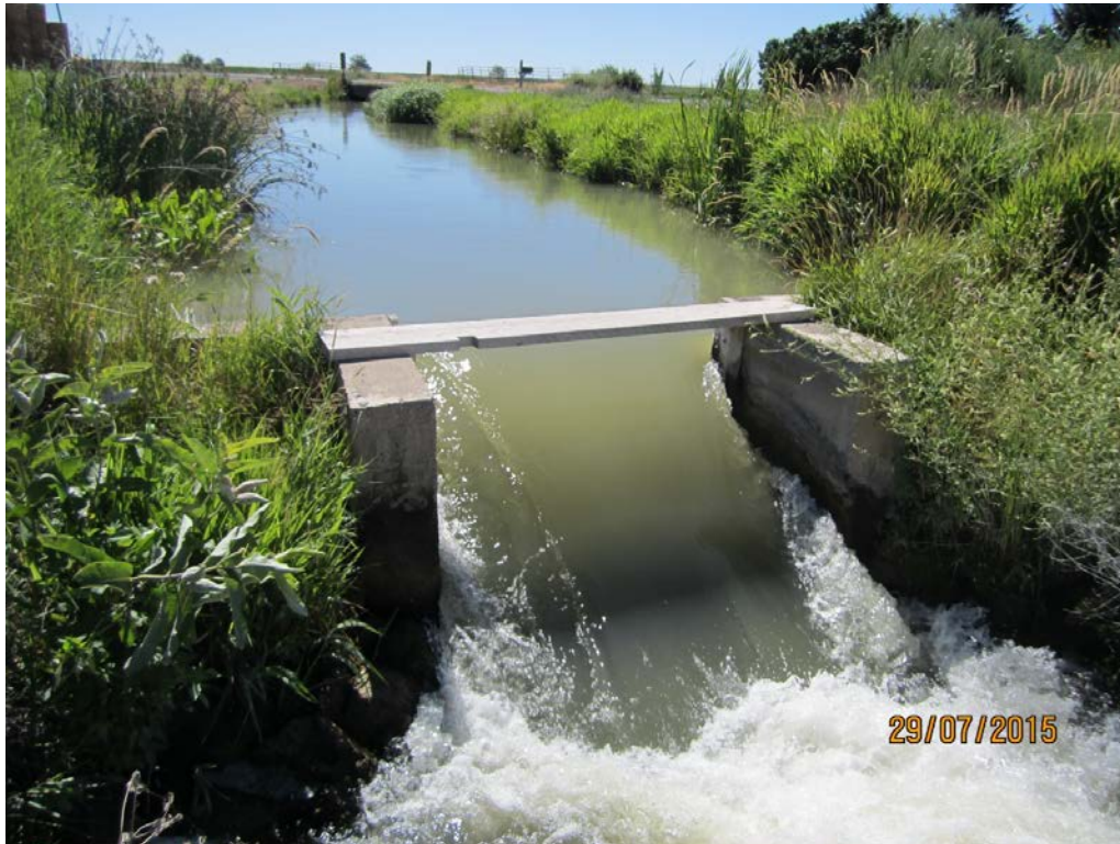
5. Check structure in Union Ditch at L2 head gate (behind check dam to right). Check is used as rectangular weir for measurement of the Union Ditch.
