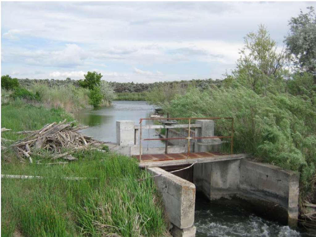
2. Union Ditch control structure and head gate.
