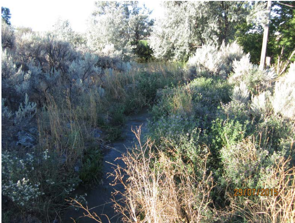
3. Mabbut 70P: Open ditch from 5 HP pump.
