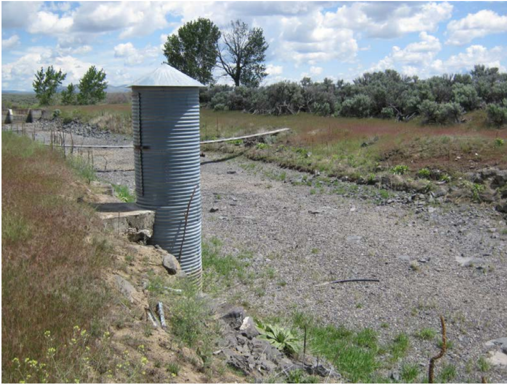
3. Lincoln Bypass Canal rated section with stilling well shed for continuous water level recorder and equipment.
