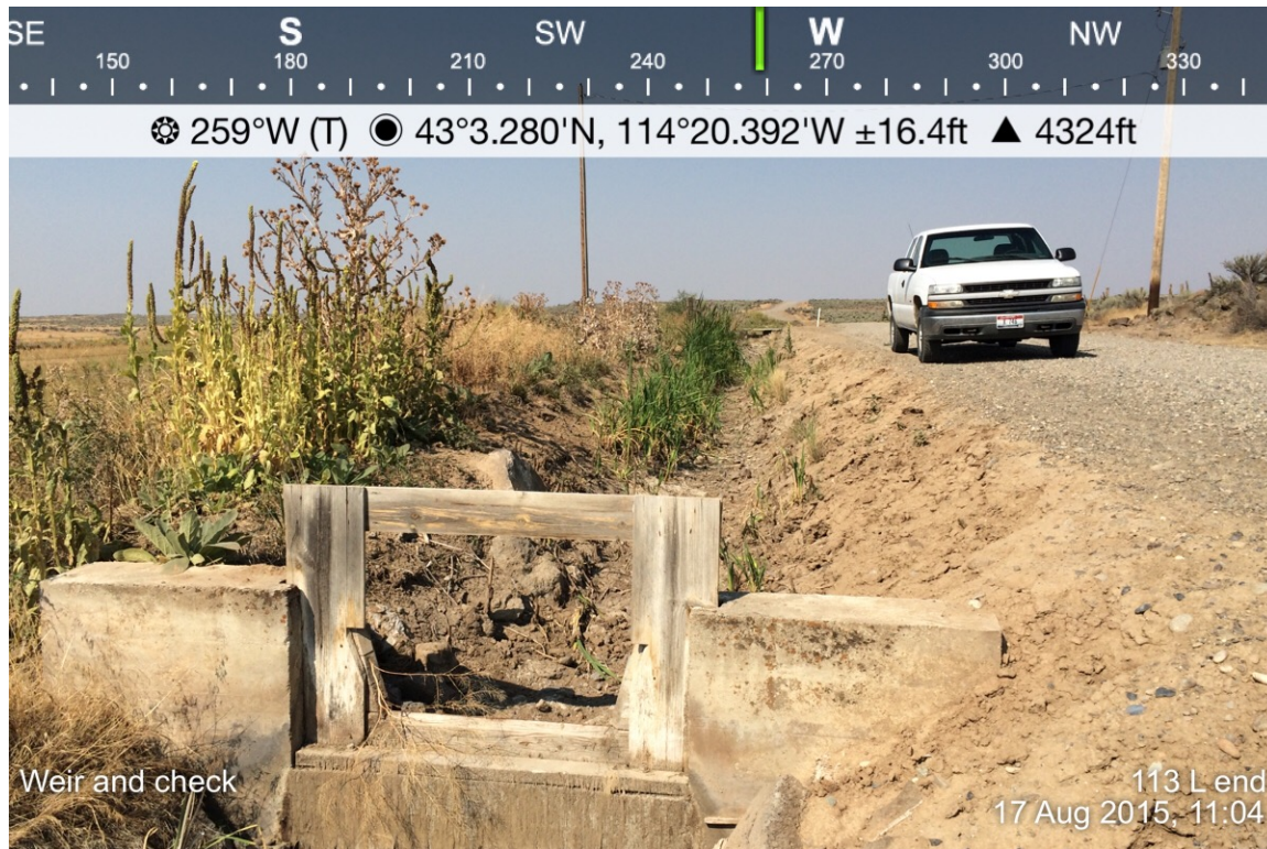
1. 113L End weir blade and check dam further up the ditch.
