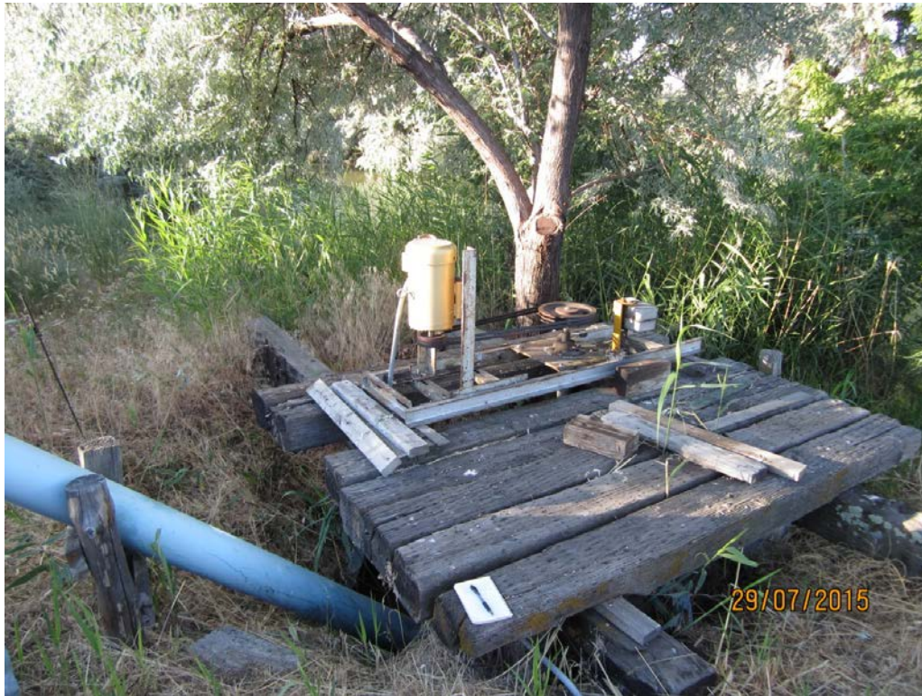
1. Mabbut 70-P: 5HP lift pump from sump to mainline and open ditch.
