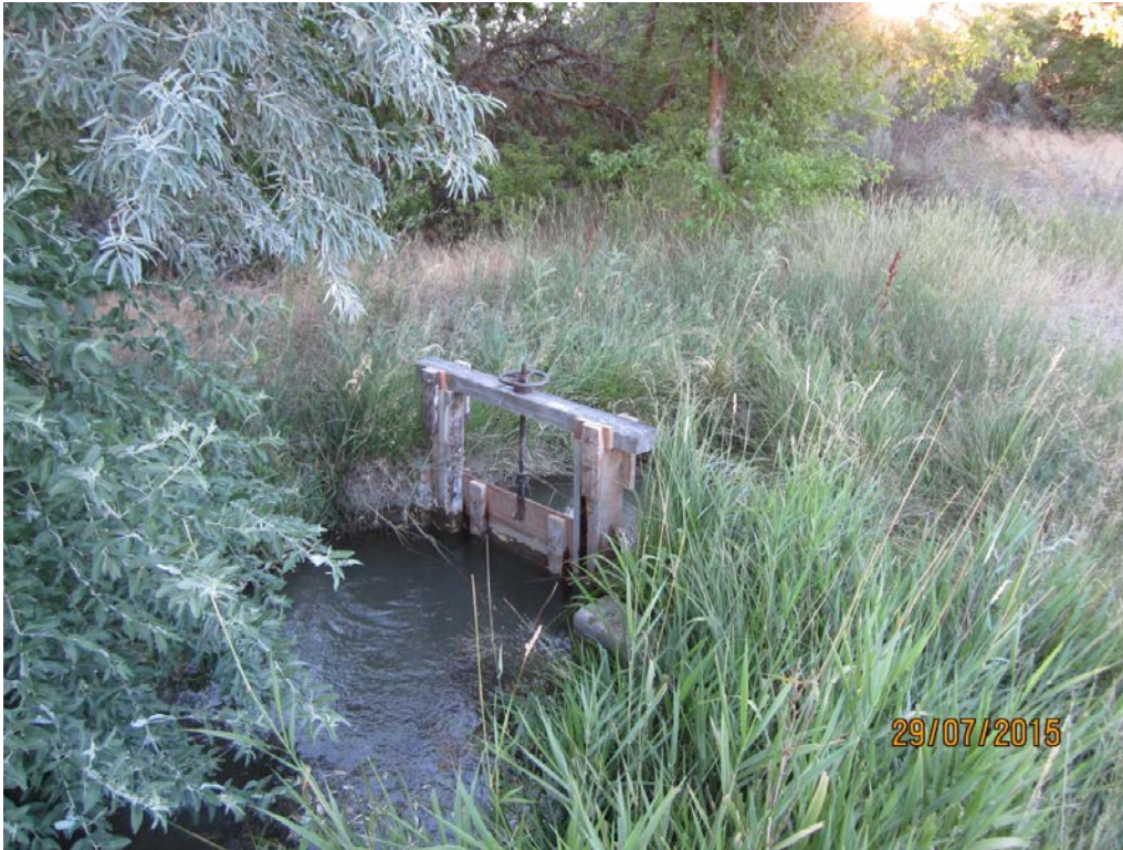
1. Mabbut 70 Ditch: orifice-gate box, rock diversion dam in river background not visible. Open ditch channel to fields on left
