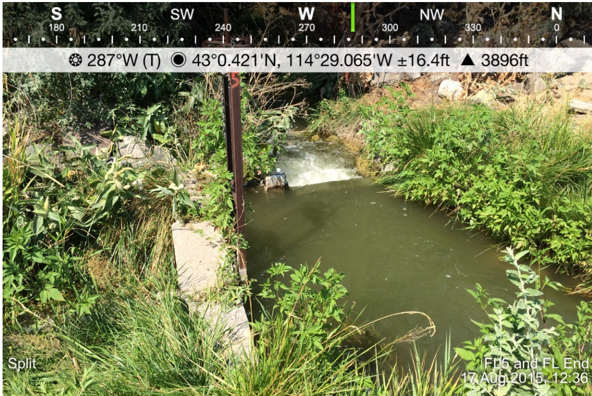
1. The FL5 diversion is a 10" screw top head gate, also shown is the FL End weir.
