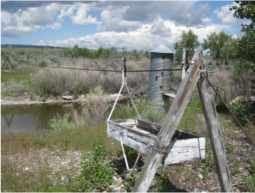
10. Big Wood River Gage Station #5 located in river below Richfield Canal spill gates; cable care in foreground and stilling well behind it.
