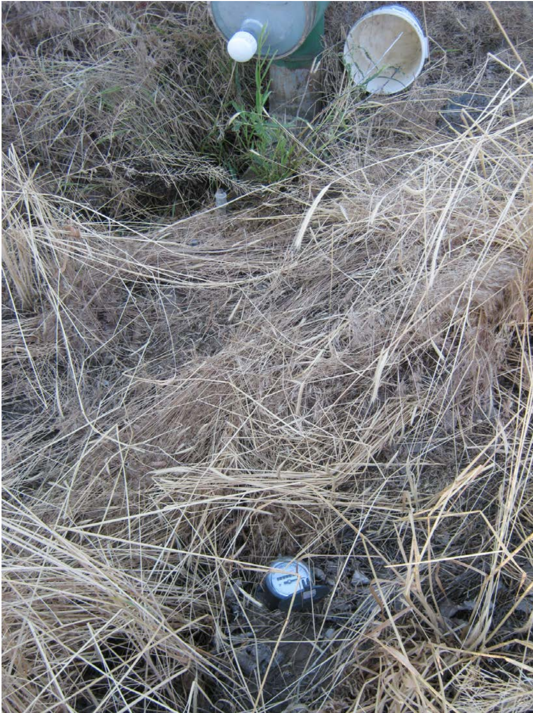
2. Faulkner – Bliss Point pump: McCrometer flow meter on mainline below dragon filter.
