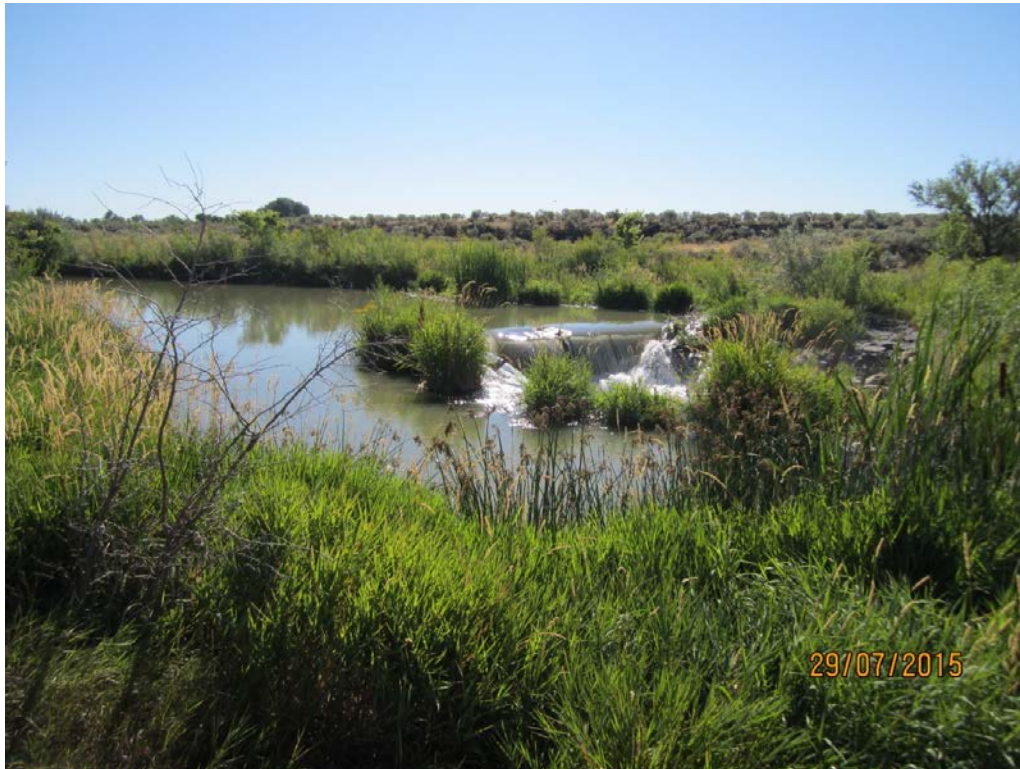
1. Robertson Ditch diversion dam across Big Wood River.
