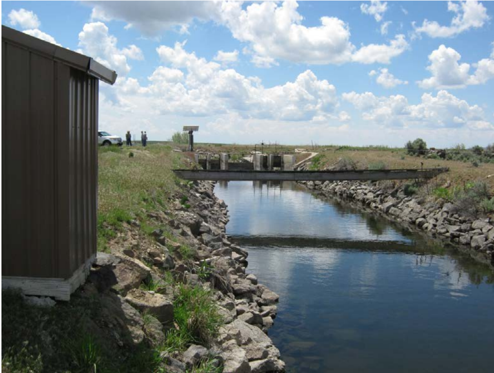
12. Jim Byrns Slough: Downstream view of head gate structure taken from measuring device and stilling well shed.
