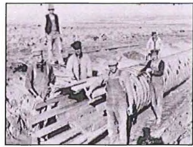
Building wood pipeline, March, 1912. Part of the Milner project. Idaho State Historical Society.
