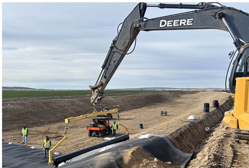
Construction crews install HDPE liner in the Highline Canal. (Photo by Steve Stuebner/IWRB)
