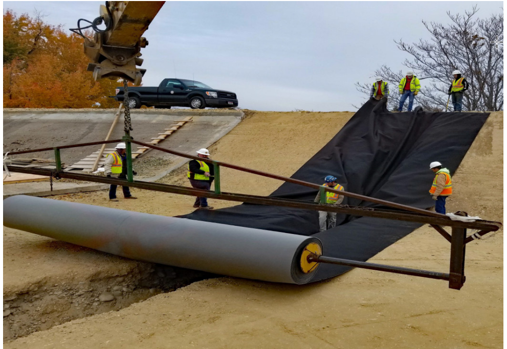
Construction contractors unfurl roll of geomembrane fabric in the New York Canal. Below, locator map shows the 41-mile course of the New York Canal.
