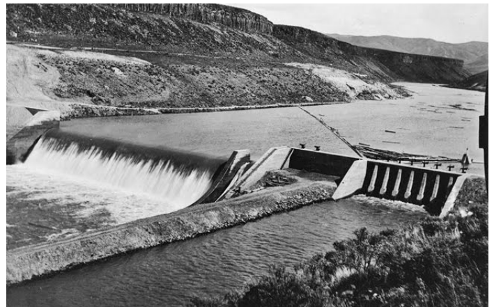
Boise River, Diversion Dam and the New York Canal when it became operational in 1909. (Courtesy National Archives)
