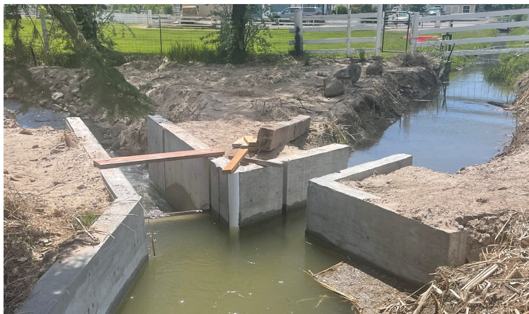
New headgate installed with 45-degree angles to divert flow to ag lands (left) and residential water users (right). Photo courtesy Dennis Hone.
