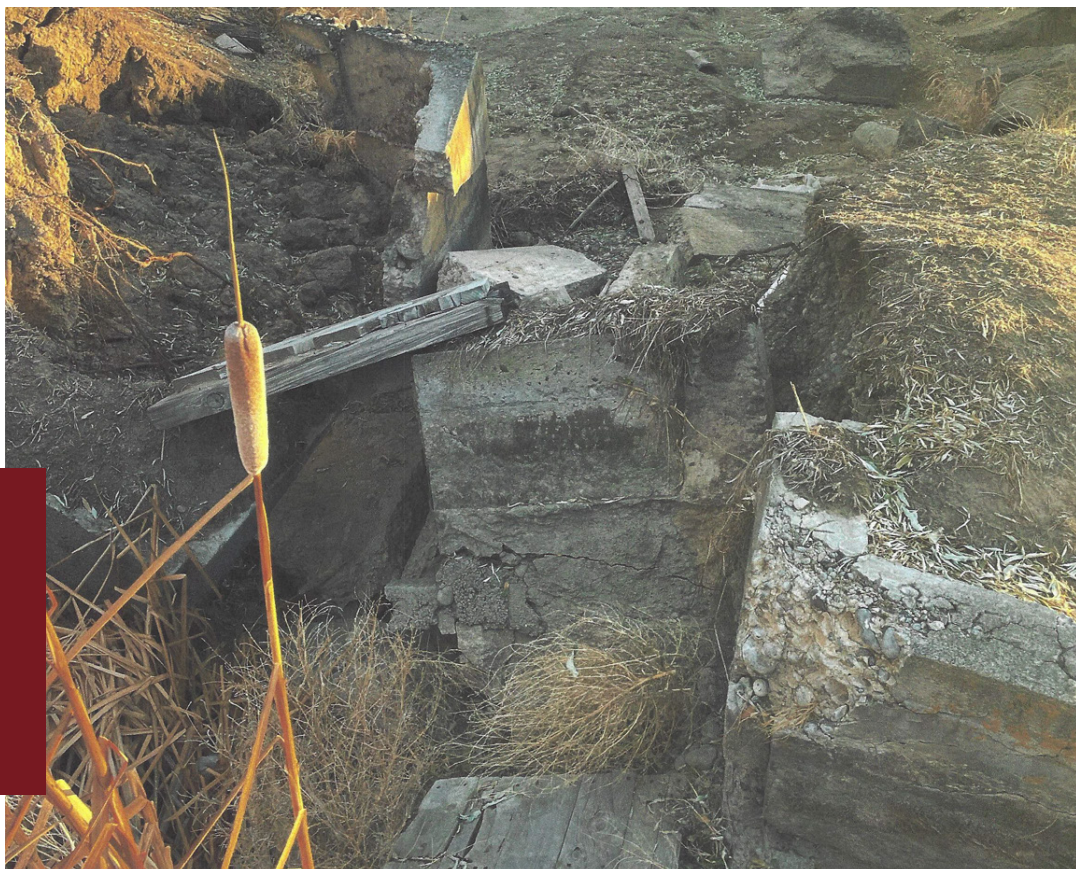
Top, the old headgate. The structure completely failed after the 2022 irrigation season. Below, another view of the new headgate. (courtesy Dennis Hone)
