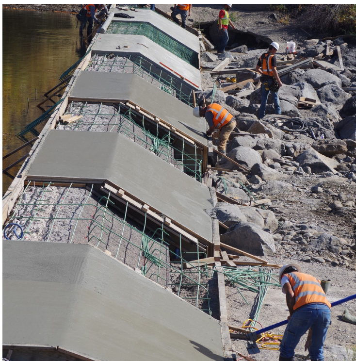
Braun-Jensen construction crew smoothes out concrete on the face of Galloway Diversion Dam. (photo by Steve Stuebner)
