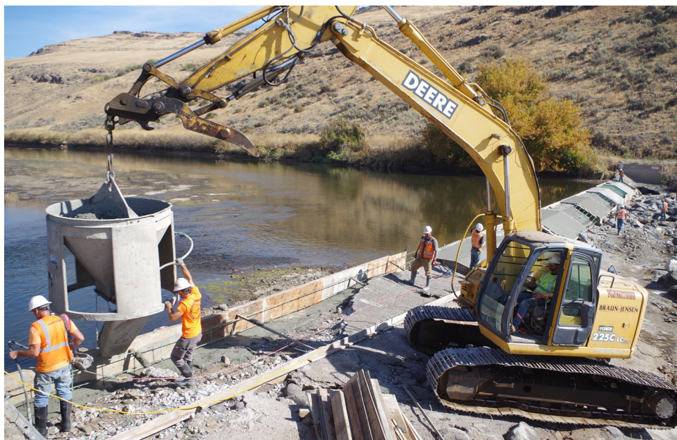
Above, Galloway Diversion Dam pre-construction. (courtesy Meghan Brooksher) Below, Braun-Jensen construction crews pour concrete into forms on the dam's crest in October. (photo by Steve Stuebner)
