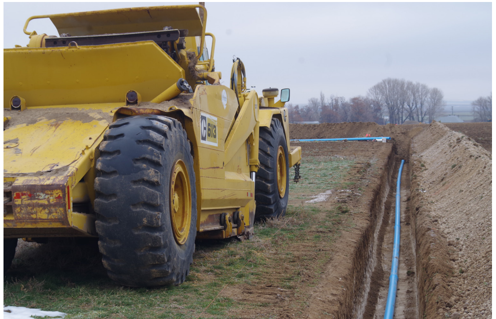
Construction contractors are busy with trenching work to install 16.3 miles of pipelines as part of the new irrigation efficiency system by April 2024.
