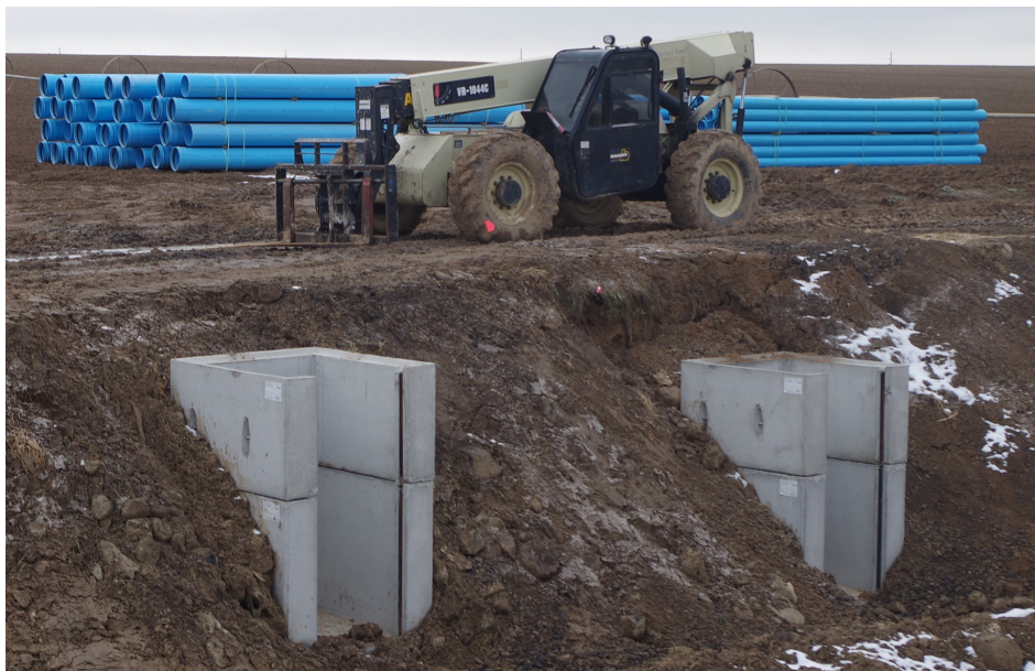
Concrete foundations for irrigation pumps are set in place along an open canal. New irrigation pipe is staged and ready for burial. (photo by Steve Stuebner)
