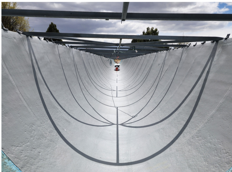
Last Chance Main Flume old liner was replaced with a fresh coating of "Aqualastic" after contractors did extensive repairs and grinding to prepare the surface for the new liner material (photo courtesy Mark Mathews, Last Chance Canal Co.).
