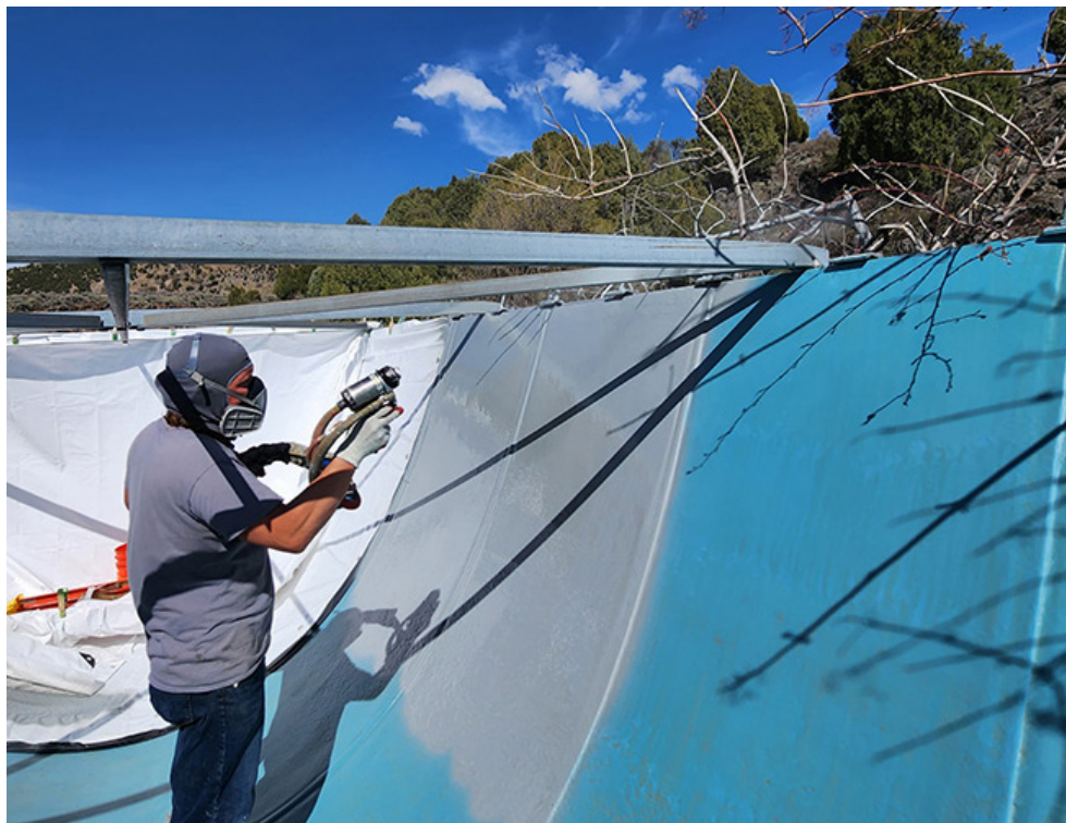
Above: Last Chance Main Flume (courtesy Bear River Heritage Area). Below, construction crew grinds down the surface of the flume and repairs cracks in preparation for new liner coating (courtesy Last Chance Canal).
