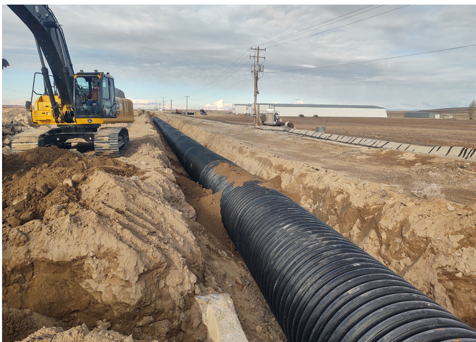
Contractors install 60-inch, double-walled pipe to replace one-quarter mile of old, crumbling concrete open canal. (Courtesy Hat Butte Canal Co.)
