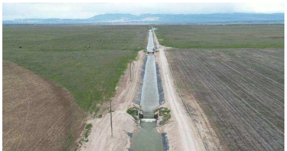
Above: Map of the Grindstone Butte irrigation system. Below, the Grindstone Butte Canal following the installation of the new HDPE liner. (Photo courtesy Bret Andersen)
