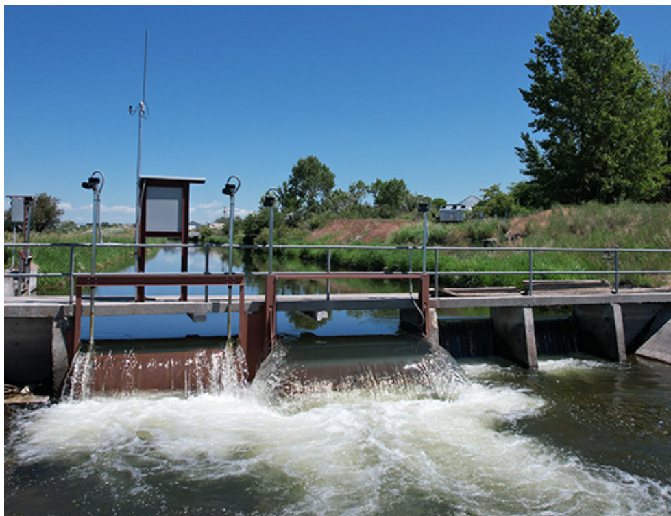
The newly modernized Crosscut Canal check structure was rebuilt during the winter months so it could be operational in the 2025 irrigation season. (Photo courtesy FMID)
