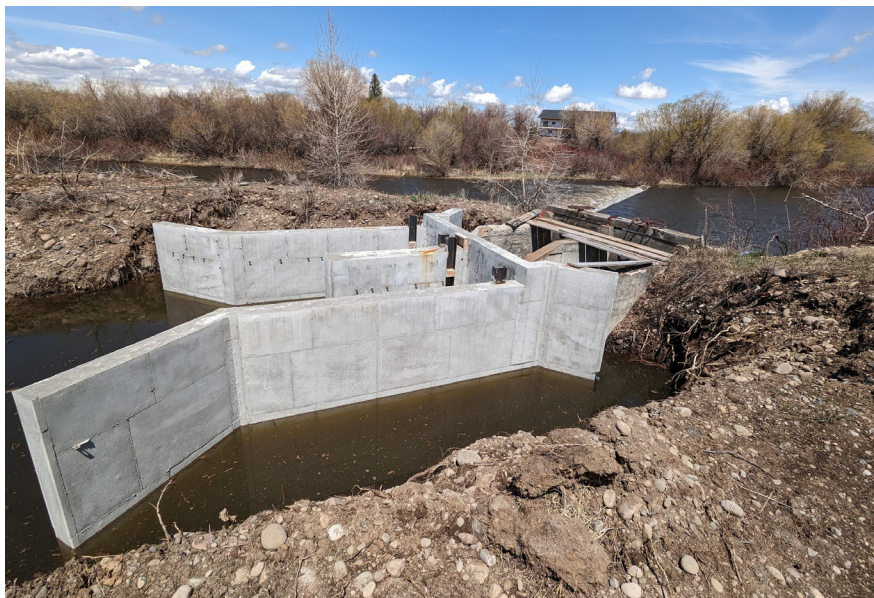
New headgate under construction on the Chester Canal.
