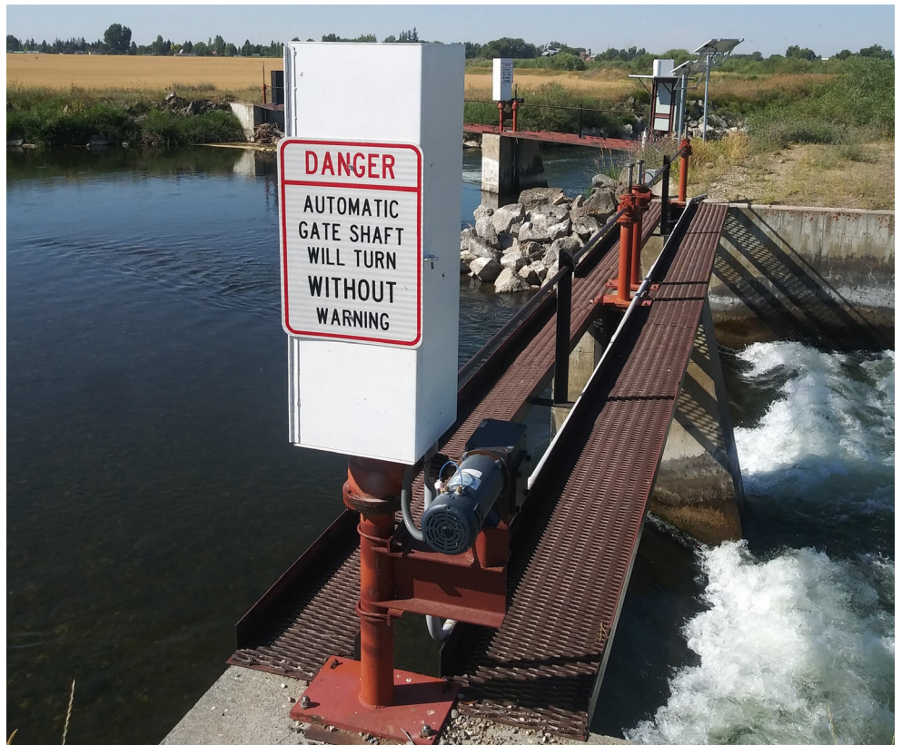
Top, example of automation equipment installed on a modern headgate on the North Fork of the Teton River. Below, the old Chester headgate.
