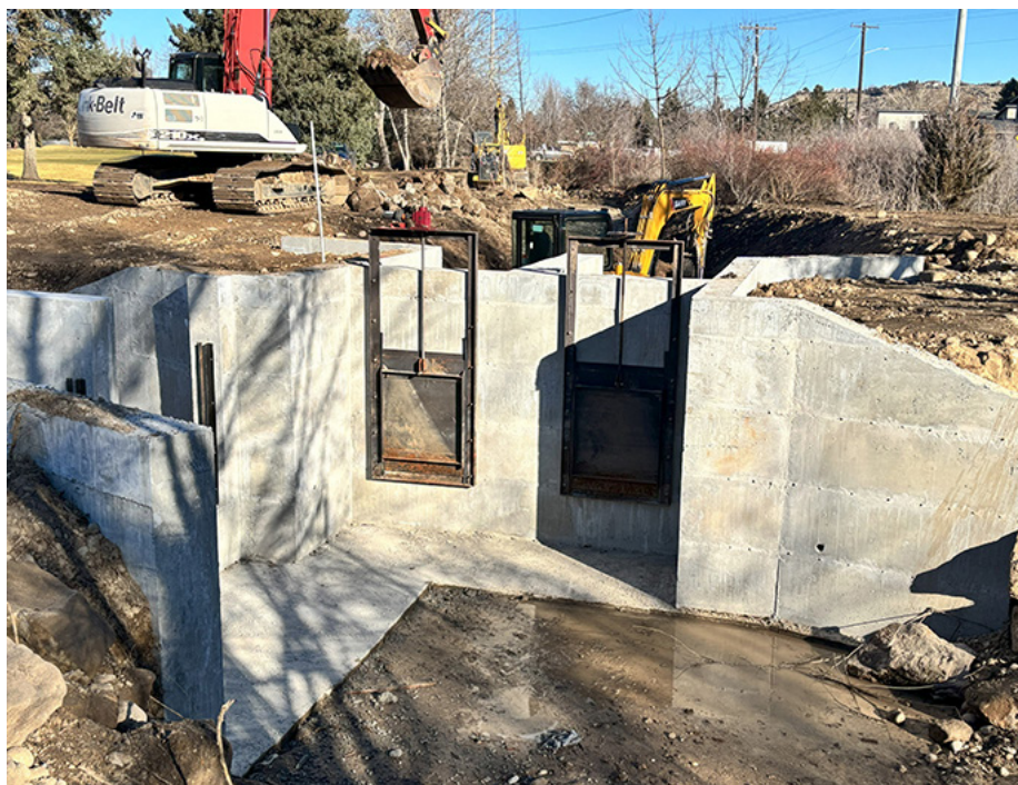
New headgate for the Boise City Canal Company is ready for the 2025 irrigation season. The headgate is located on the eastern edge of Warm Springs Golf Course. Goodwin Dam on the Boise River diverts water to the headgate for BCCC. (photo by Steve Stuebner/IWRB)
