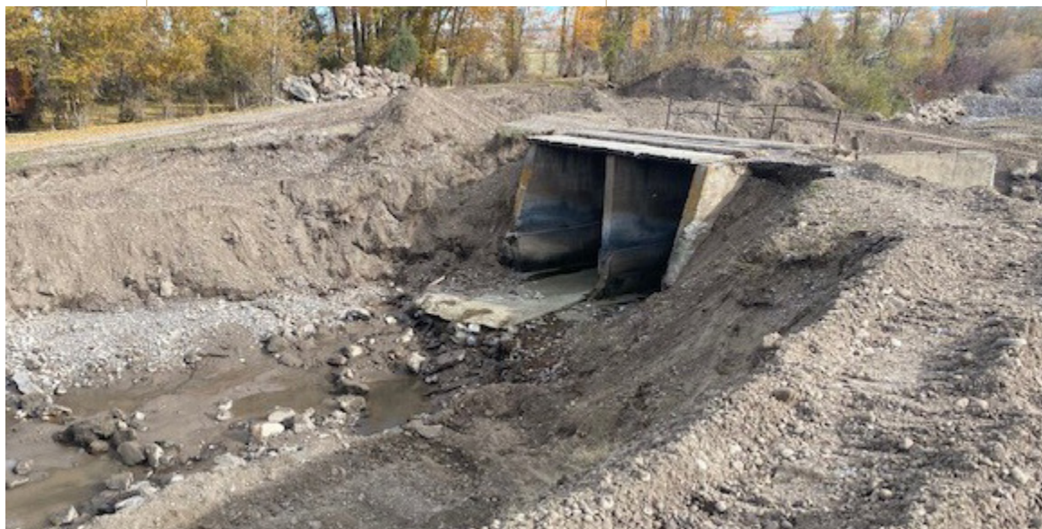
Top, the old headgate. Below, excavation work begins in October 2022 to prepare for removing the old headgate and installing the new one. (courtesy Bannock Feeder Canal Co.)
