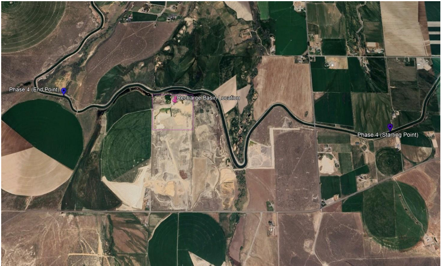
Figure 5: Location of Lateral 1 (4HL) High Line Liner and Sustainability Project.
