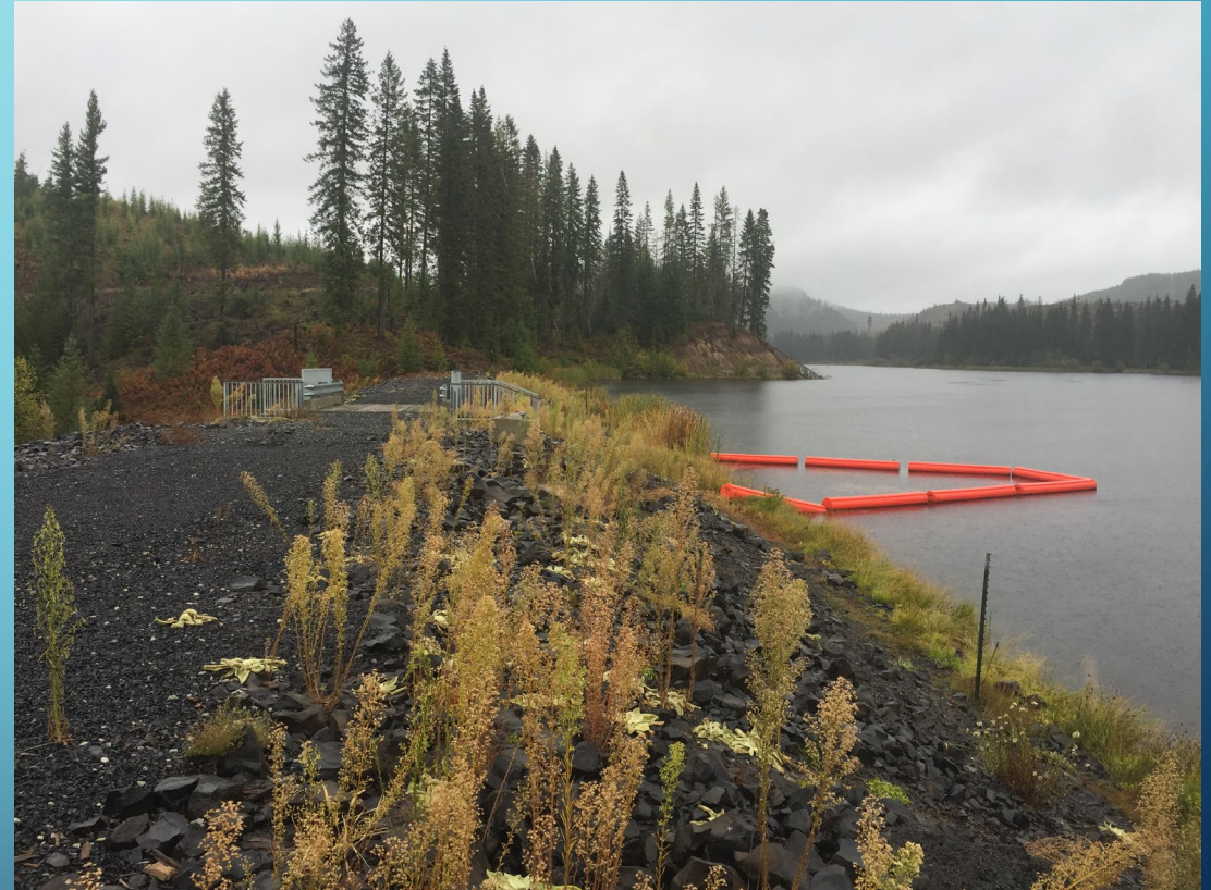
Deer Creek Dam, East of Dworshak Dam
