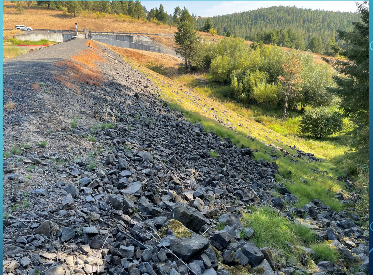
Spring Valley Dam near Troy, ID
