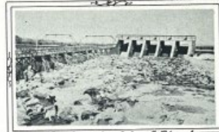
Headworks - Island Plant
