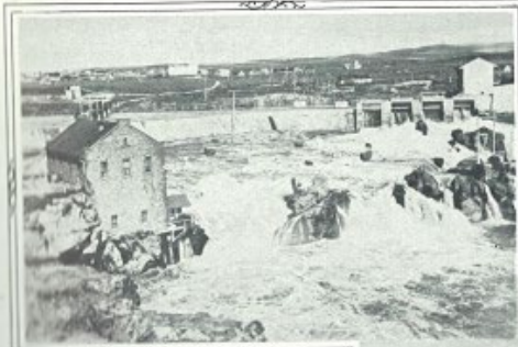
Island Plant & Dam
