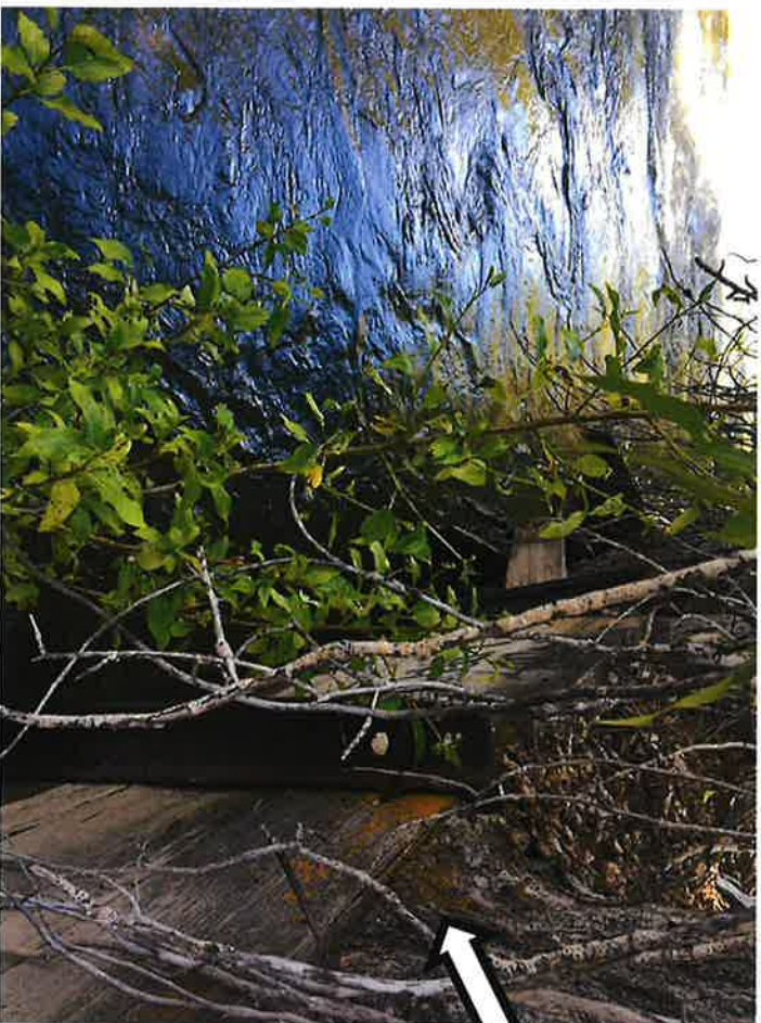
Degraded Wooden Planks
