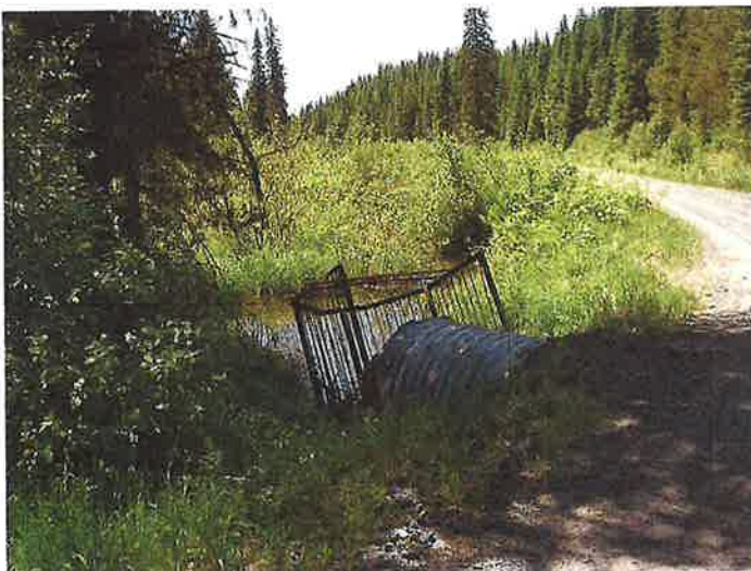
Third Crossing on Canal Creek, inlet. 36" culvert; replace with 73" X 55" pipe arch
