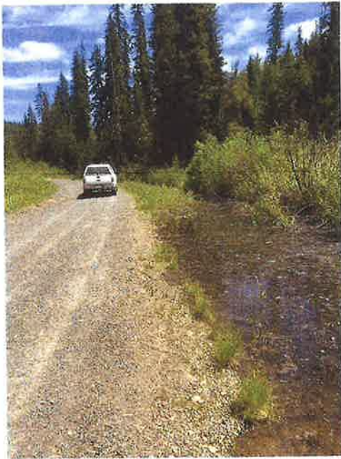
Flooding along Canal Creek due to undersized culverts, after water has receded. At higher flows, the water is over the road.
