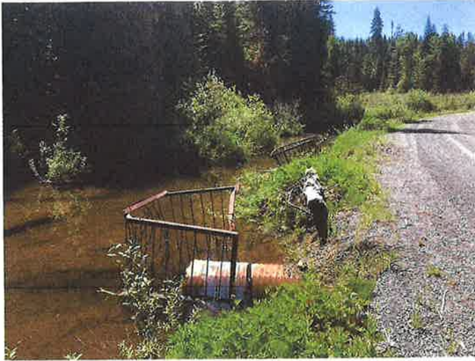
First Crossing on Canal Creek, inlet. 2 36" culverts with beaver/trash racks Replace with 81" X 59" pipe arch
