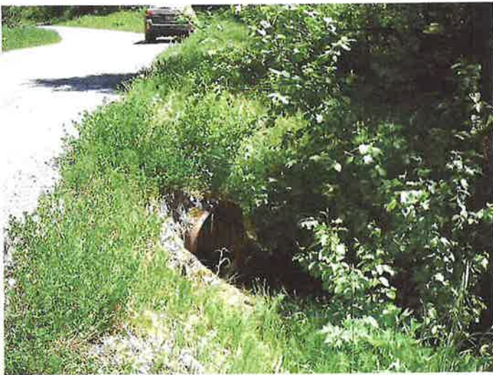
Second Crossing on Canal Creek, inlet. 36" culvert; replace with 73" X 55" pipe arch
