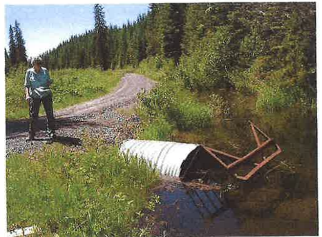
Fourth Crossing on Canal Creek. 60" culvert; replace with 73" X 55" pipe arch
