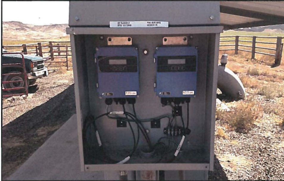
SV Ranch 2 - Two Fuji flow meters for dual penstock
