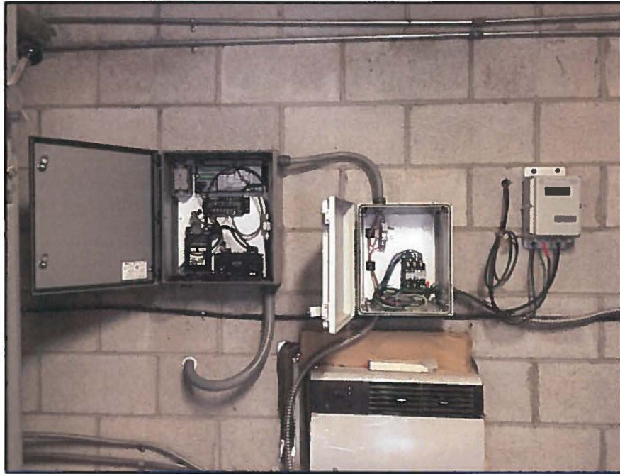
Deruyter flow meter and telemetry equipment
