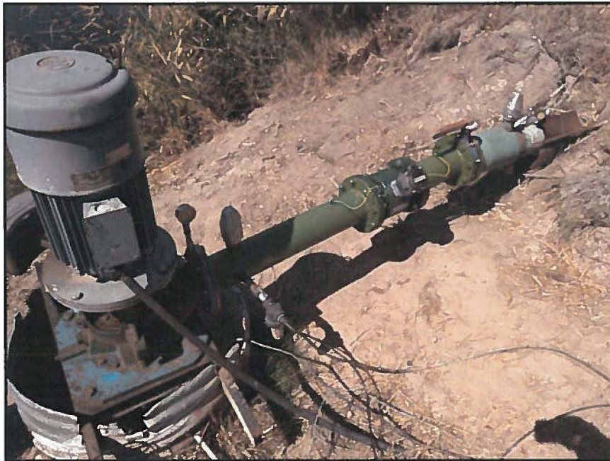
TRI flow meter installation
