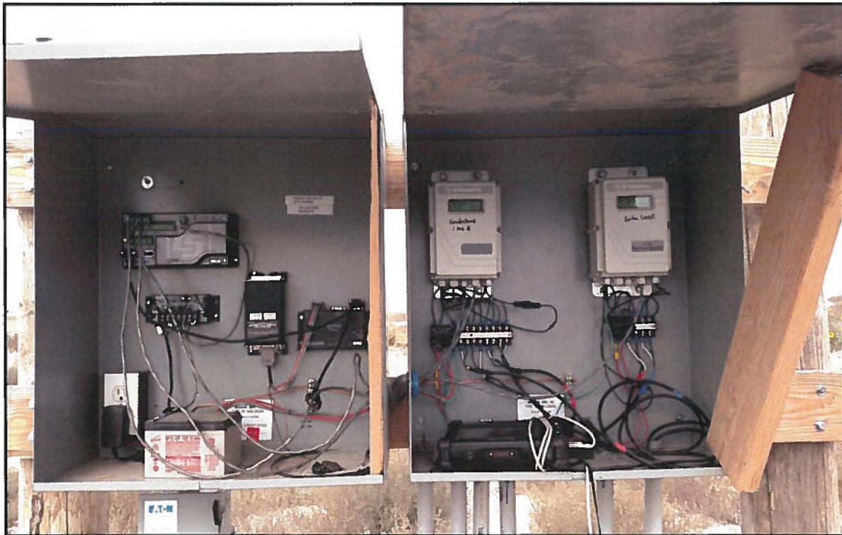
Grindstone Butte and Sailor Creek flow meter and telemetry installation
