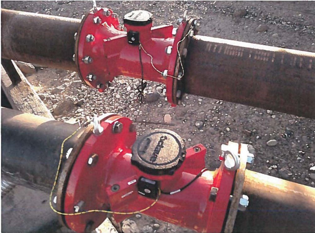
Walker Plow LLP flow meter installation
