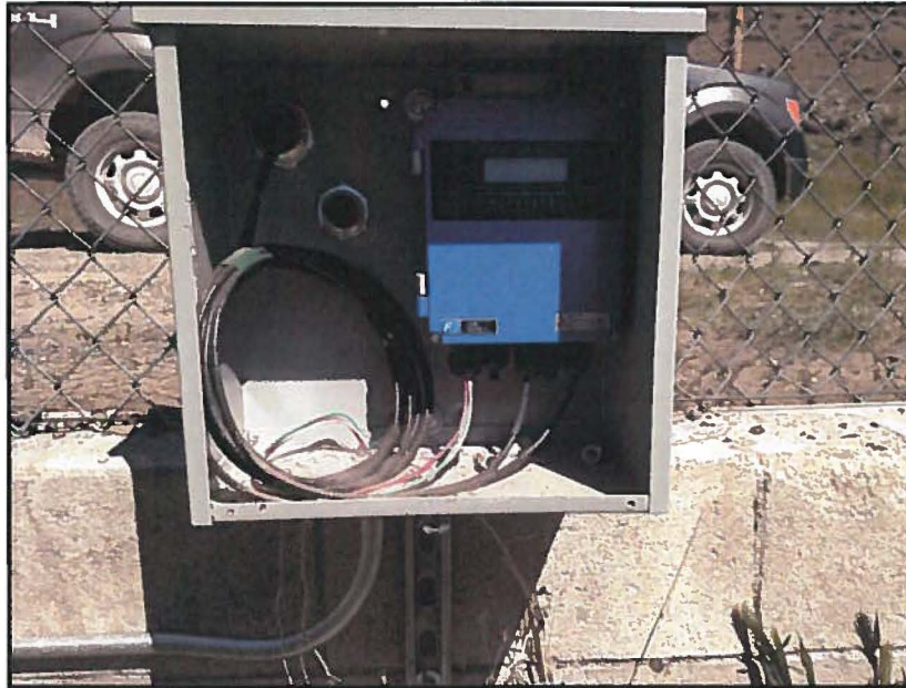
Bledsoe Flow Meter Installation
