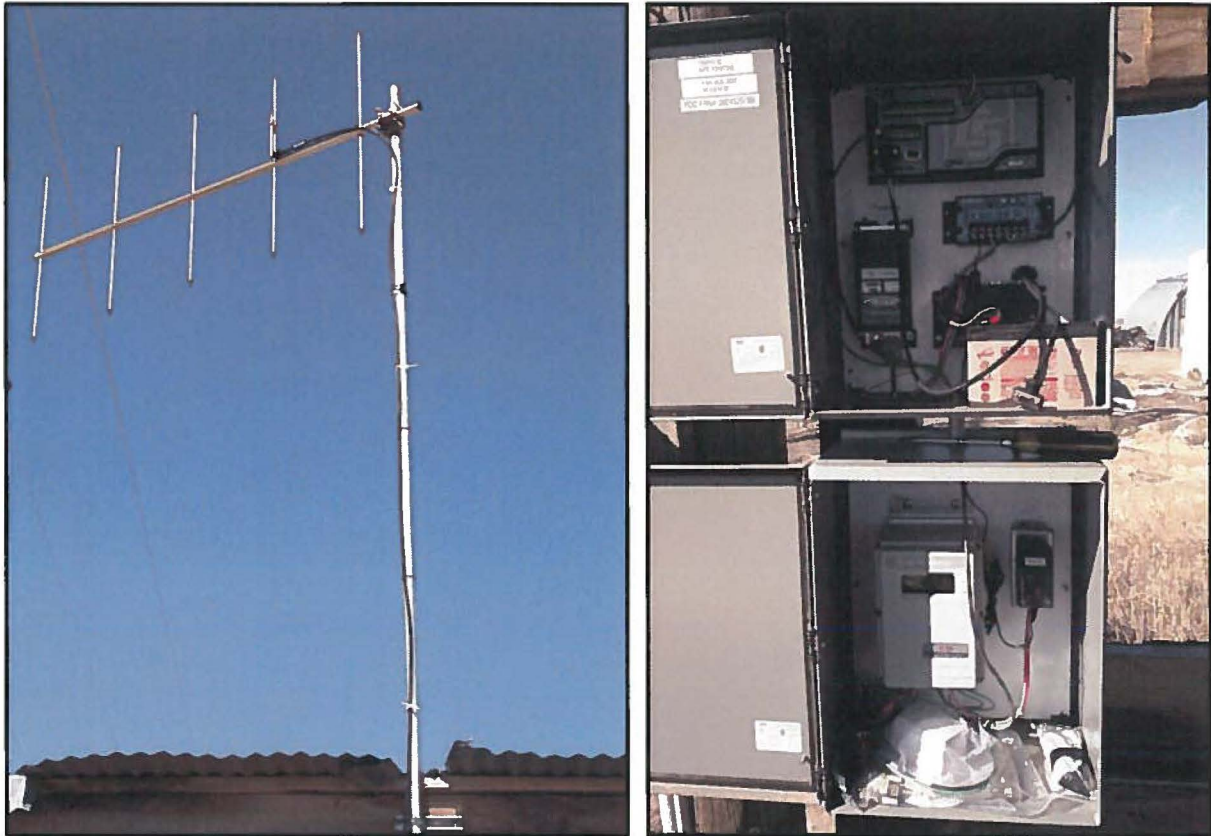
Triple C Yagi 5 element 9 dB antenna (left) and flow meter and telemetry installation (right)
