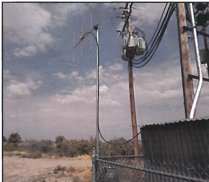
Gingerich Brothers Yagi 3 element 7.5 dB antenna
