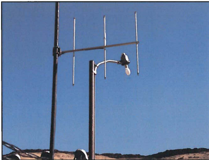
Yagi 3 element 7.5 dB Antenna at King Hill Wiley
