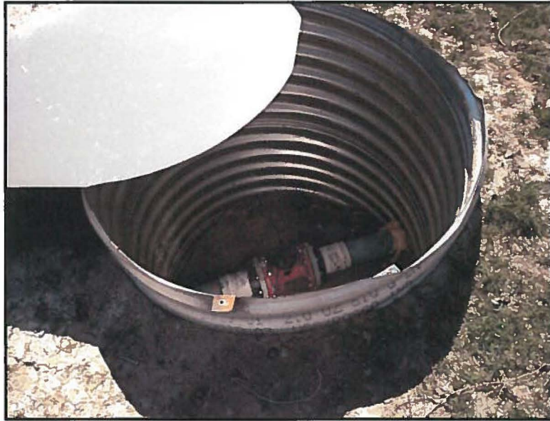
Verlin Gingerich flow meter installation
