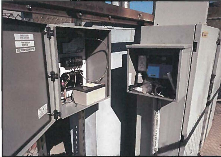
Eagle Cove flow meter and telemetry equipment
