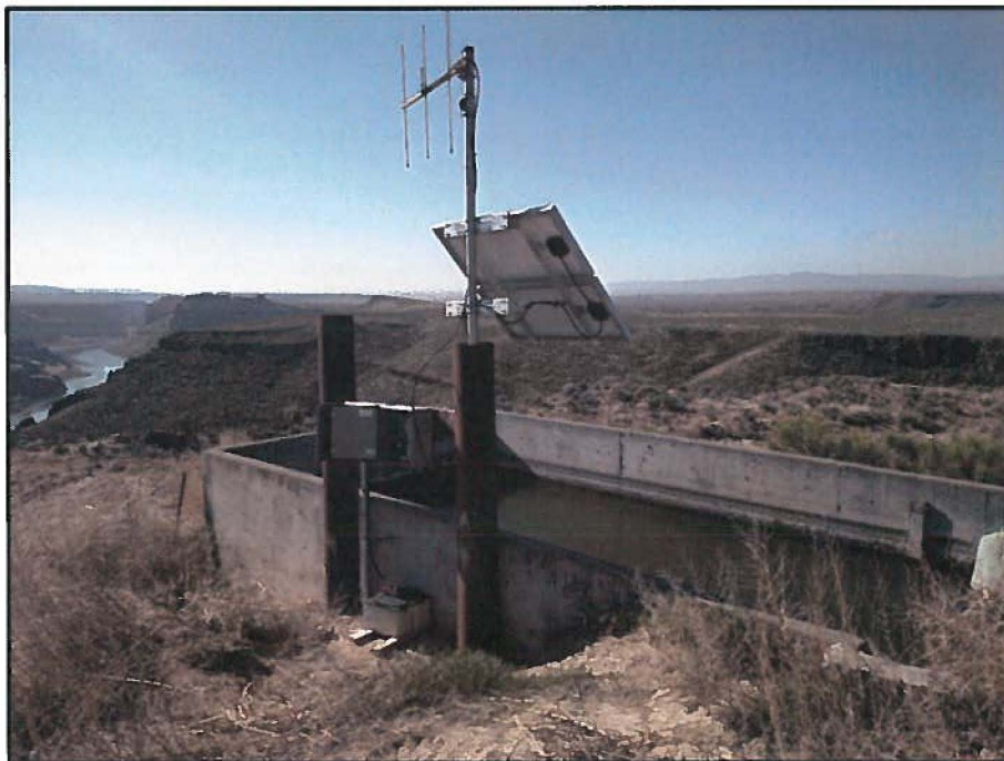
Murphy Flats Yagi 3 element antenna and solar panel
