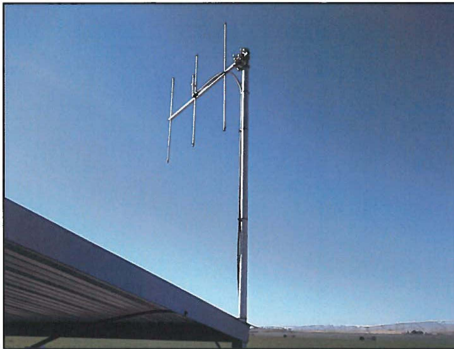
SV Ranch 2 Yagi 3 element 7.5dB Directional Antenna
