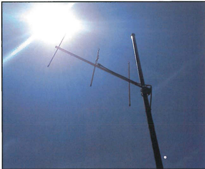
Yagi 3 element 7.5 dB Antenna at King Hill Wiley
