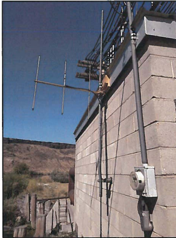
Blanksma Dunes Yagi 3 element 7.5 dB antenna
