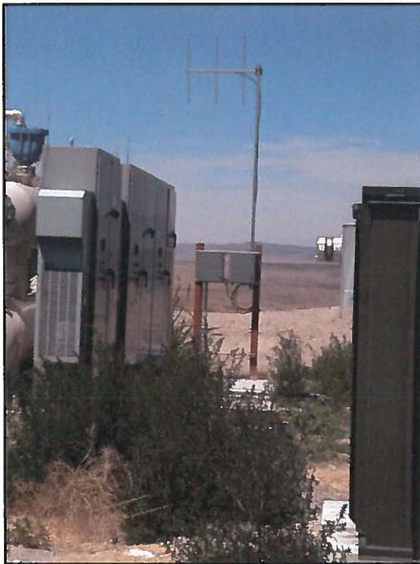
Midnight Sun Yagi 3 element 7.5 dB antenna
