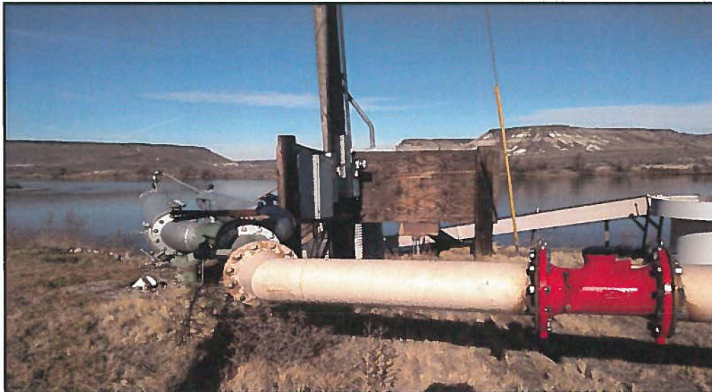
SV Ranch 3 with Octave flow meter on right (red)
