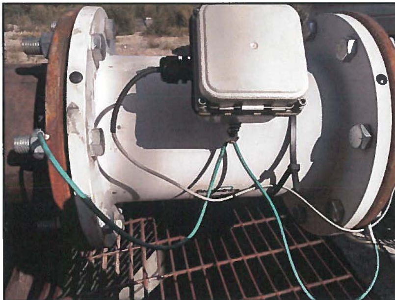
Rivendale Seametrics flow meter
