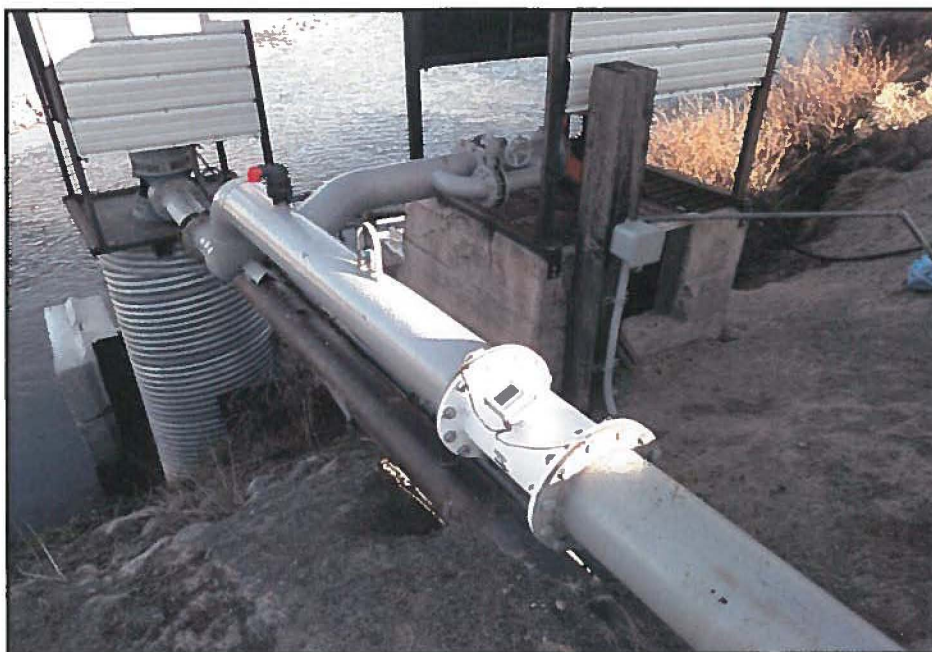
Gardner Brown Flow meter installation
