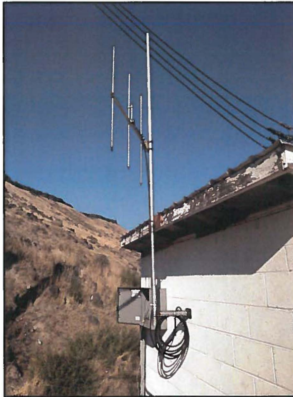
Blanksma Chalk Flats Yagi 3 element 7.5 dB antenna
