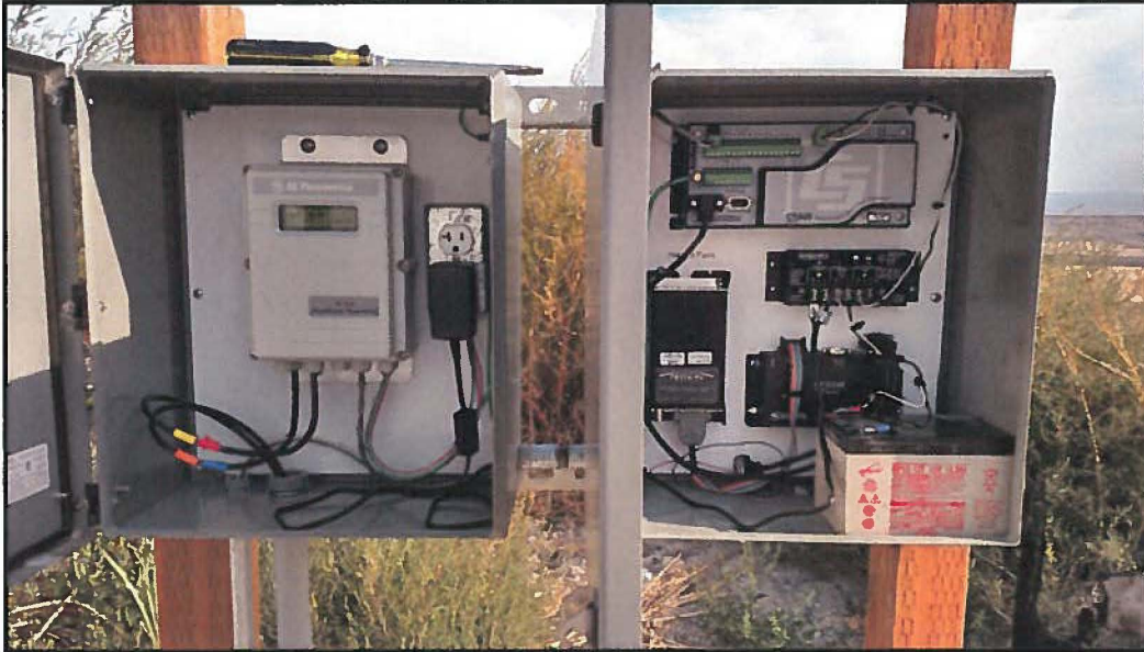
Midnight Sun Dual channel flow meter with telemetry equipment installation
