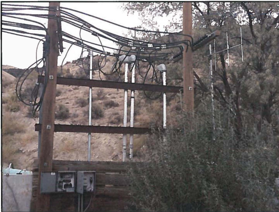
Owyhee Farms Cottonwood Yagi 3 element 7.5 dB antenna
