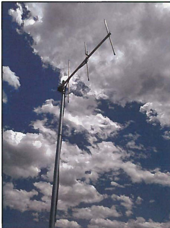
Eagle Creek Yagi 3 element 7.5 dB antenna
