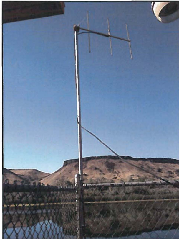
Eagle Cove Yagi 3 element 7.5 dB antenna
