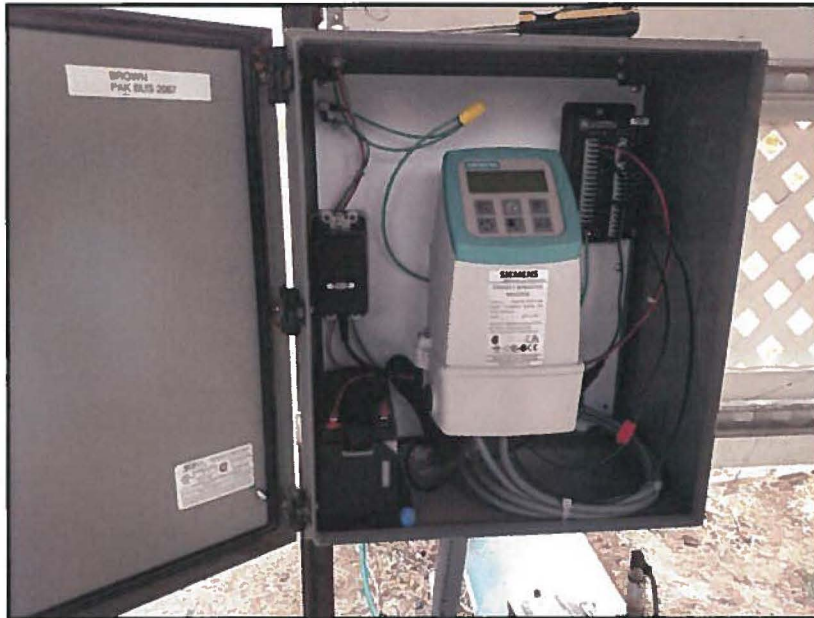
Merill Brown flow meter display and datalogger setup in protective housing
