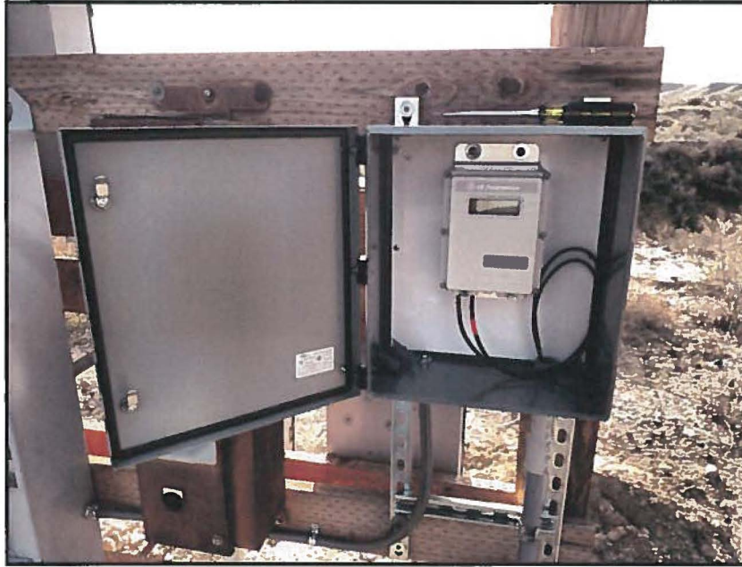
Sherwin Sundberg GE AT868 flow meter installation
