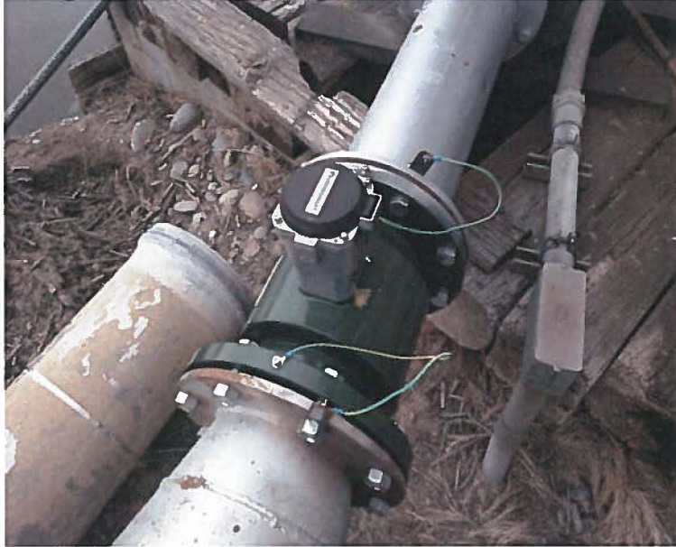
Leeland Shetler IM3000 flow meter installation
