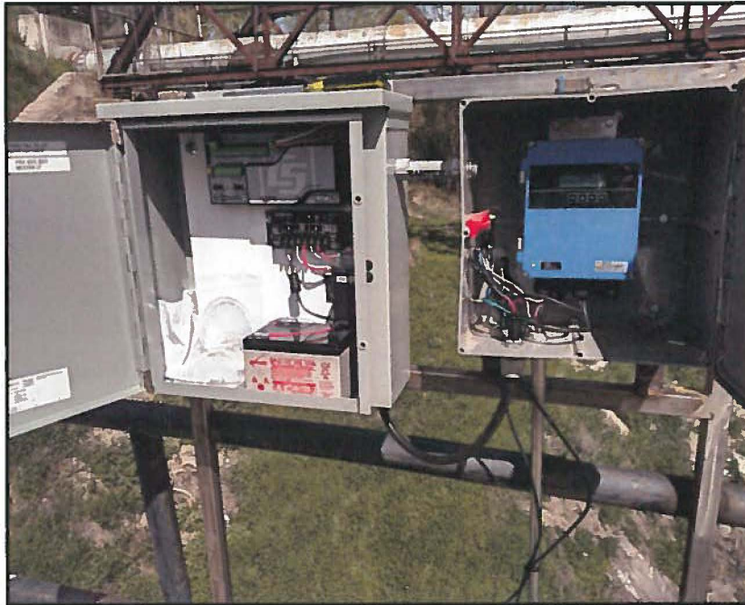
Telemetry setup and Fuji Flow Meter at King Hill King Hill
