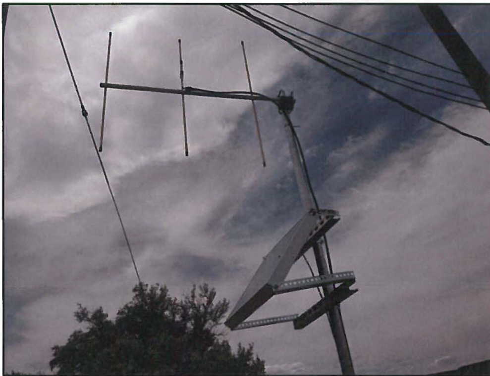
SV Ranch 3 Yagi 3 element 7.5 dB Directional Antenna
