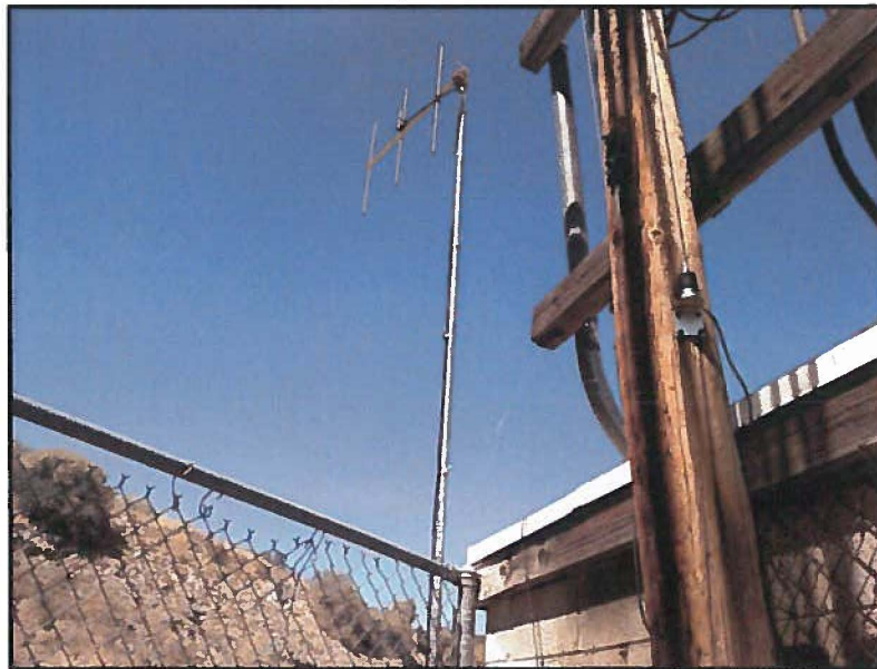
Dale Hooley Yagi 3 element 7.5 dB antenna
