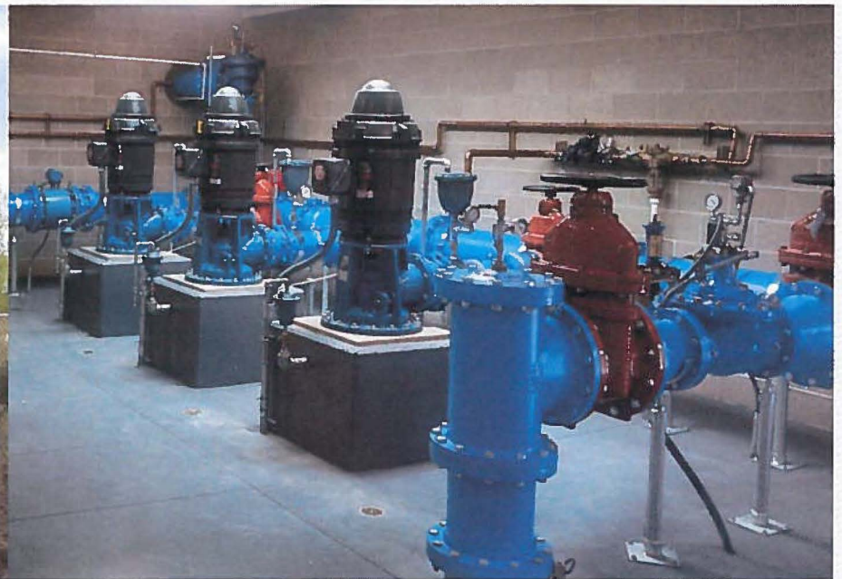
VERTICAL TURBINE PUMPS (3 EA) - 75 HP
