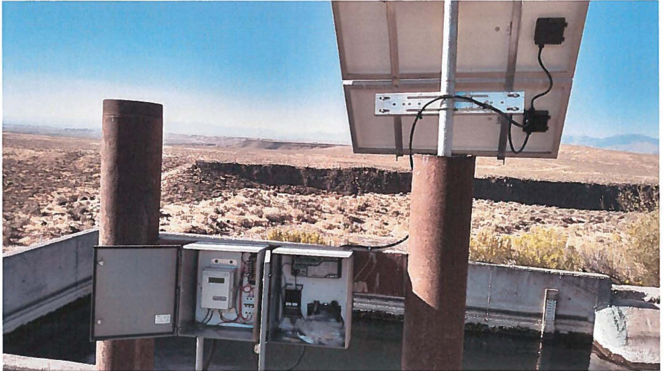
Murphy Flats flow meter and telemetry installation
