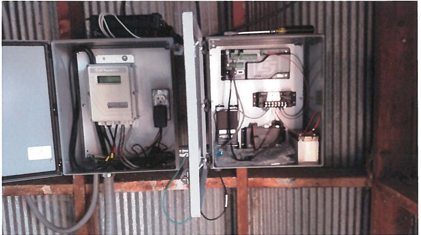
Indian Cove flow meter and telemetry installation
