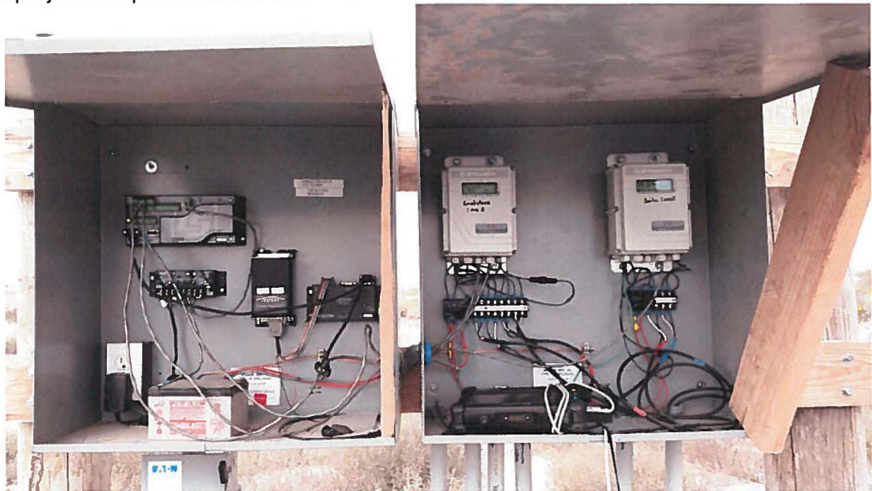
Grind Stone Butte and ATN Holdings flow meter and telemetry installation
