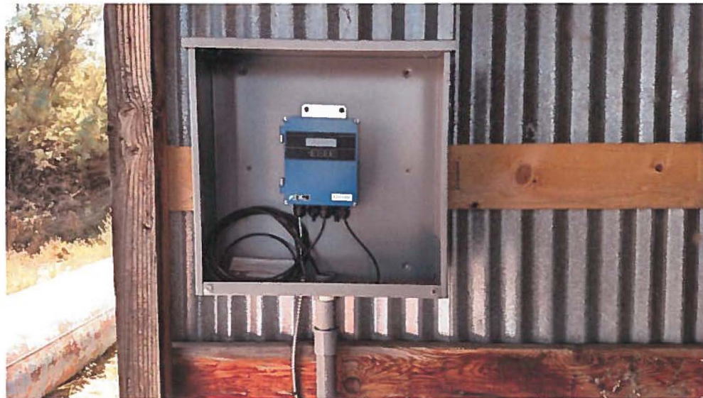
flow meter install
