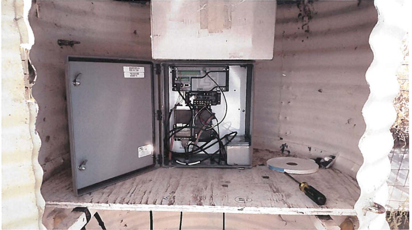
Grand View Irrigation District gauge hut with new telemetry equipment and panel
