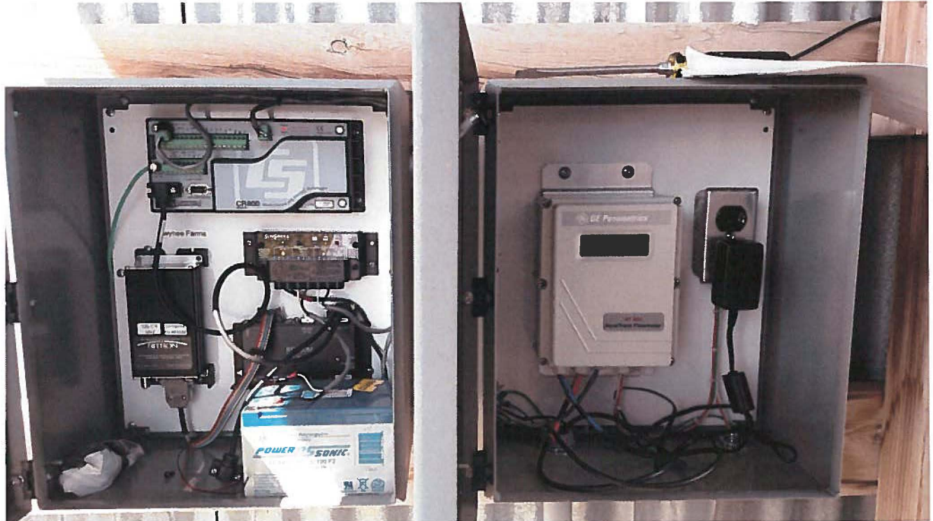
Murphy Land Company Cove Arm flow meter and telemetry installation
