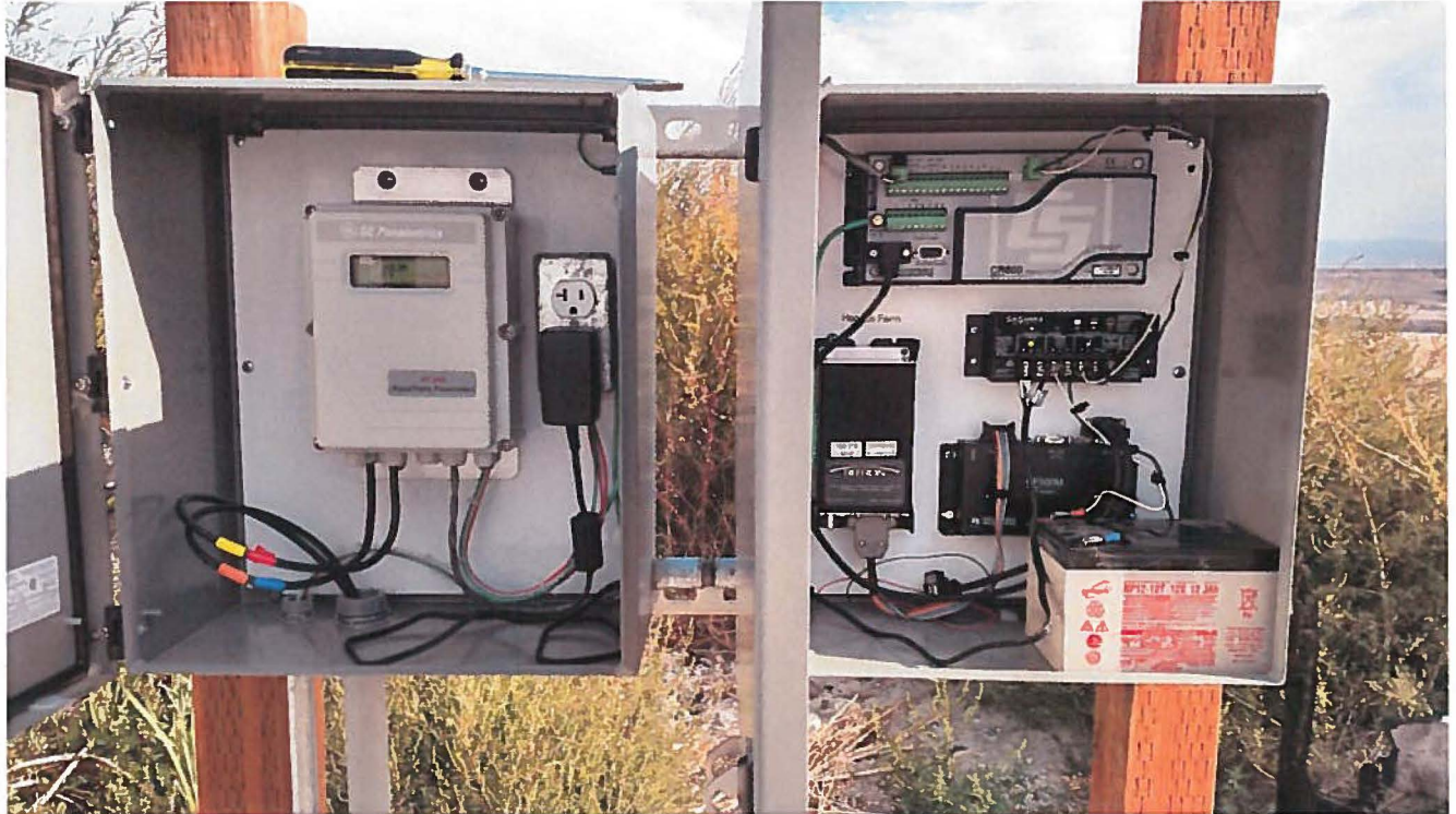
Eagle Creek flow meter with telemetry equipment installation
