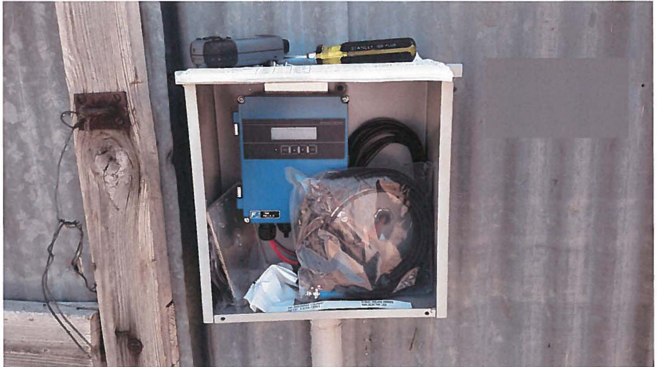
West Indian Cove flow meter installation
