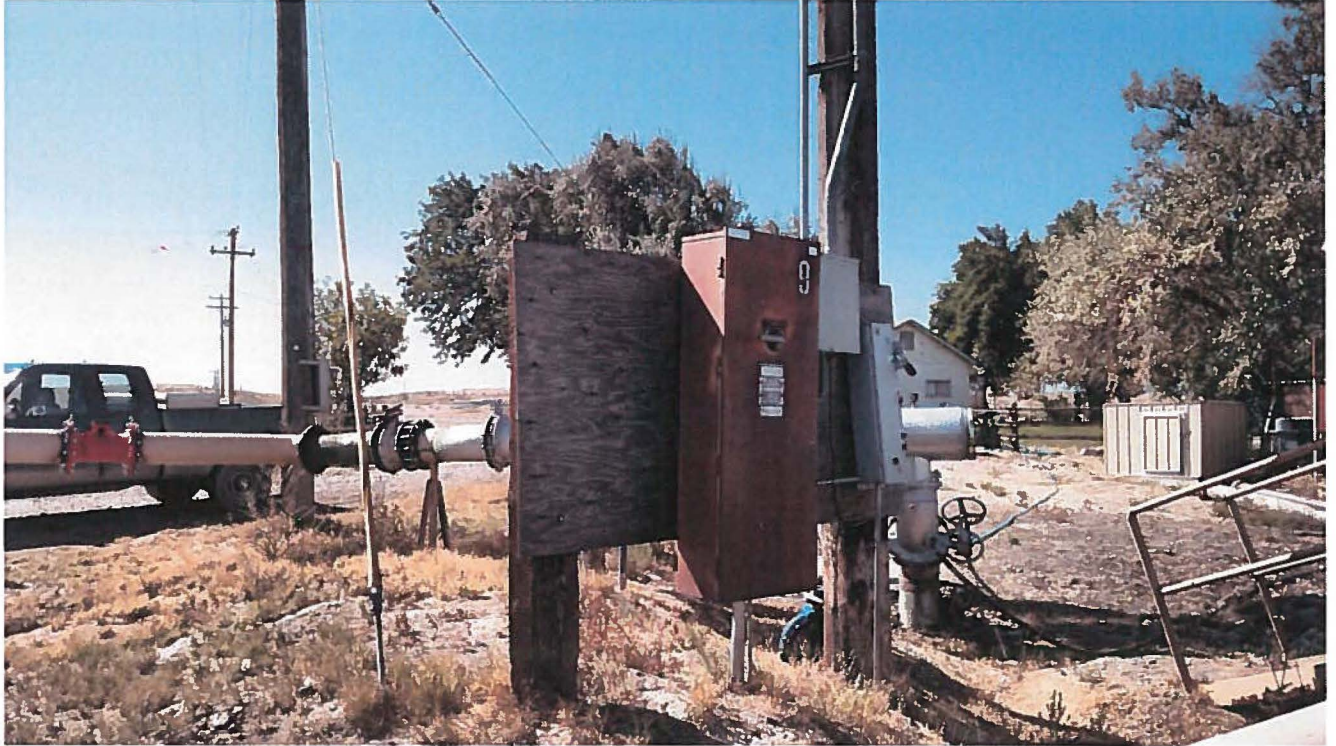
SV Ranch 3 with flow meter installed on the left side of the photo
