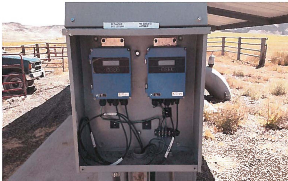
SV Ranch Site 2 two flow meters for dual penstock
