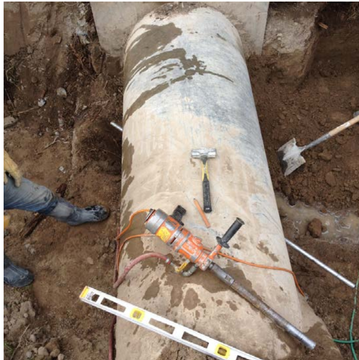
Indian Cove concrete bore 2 with alignment rod through the Low Line pipe
