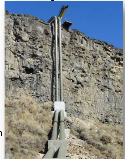
IGWA pipeline to Rangen Completed in 2015 Financed by IWRB
