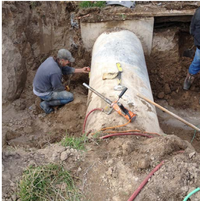
Indian Cove concrete bore 1on the Low Line pipe
