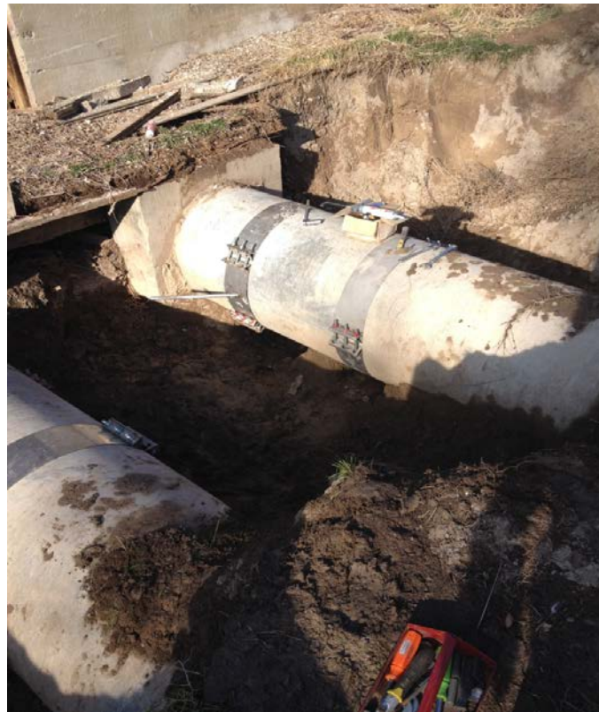
Indian Cove with bands and alignment rod in the High Line pipe
