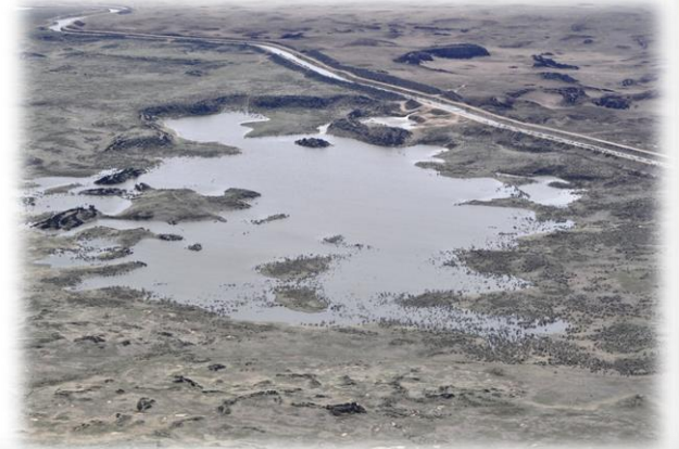
Milepost 31 recharge basin completed in 2013
