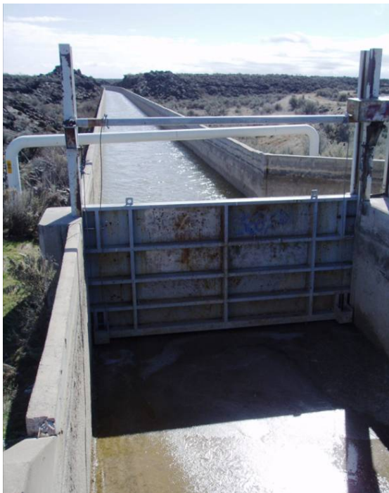
Recharge water flowing down the Milner Gooding cement flume and into the recharge basin. No water flowing past the main gate on down the canal.
