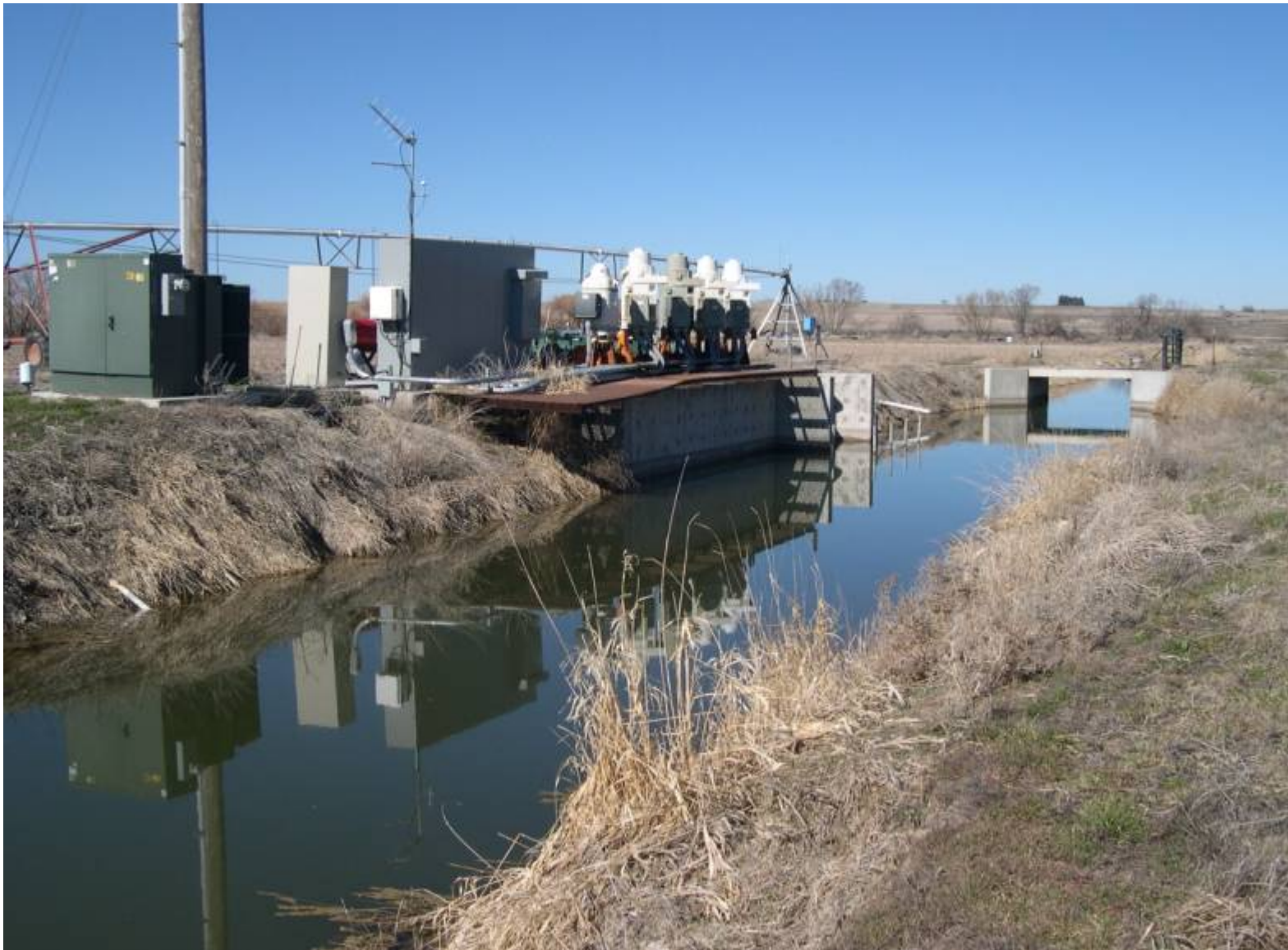
Southwest Irrigation District Milner reservoir pump station pumping Board recharge water at 27 cfs.
