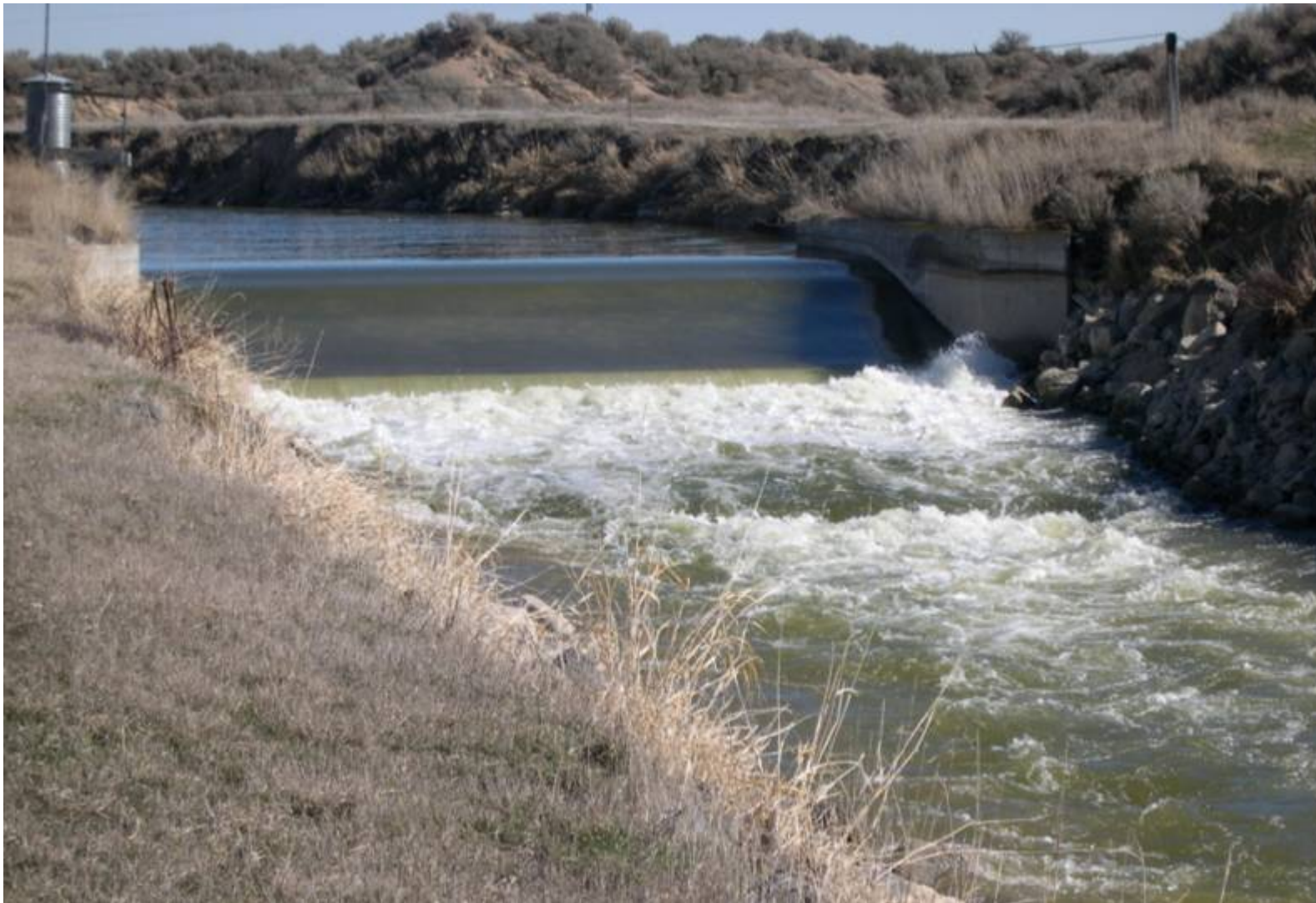
NSCC routing 600 cfs Board recharge water through the X-cut bypass weir and gauge on February 18 th .
