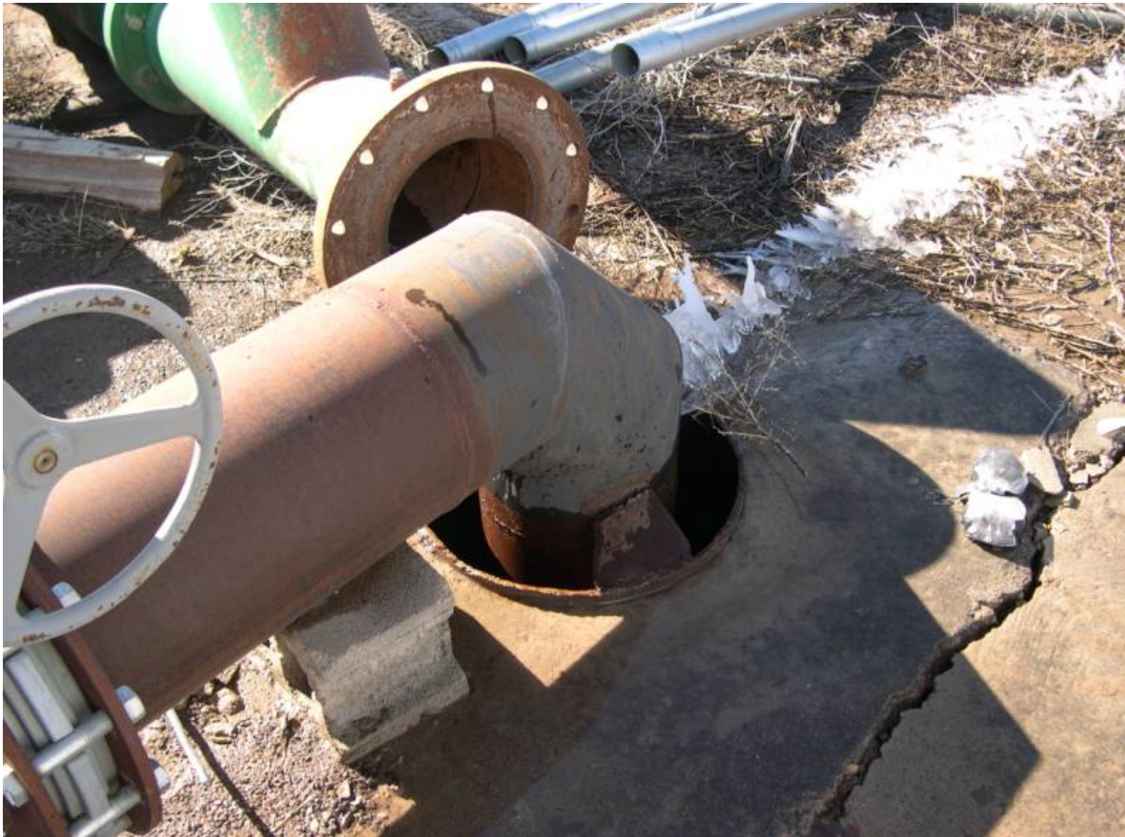
SWID injection well recharging water, measured flow 7,100 gpm (16 cfs).
