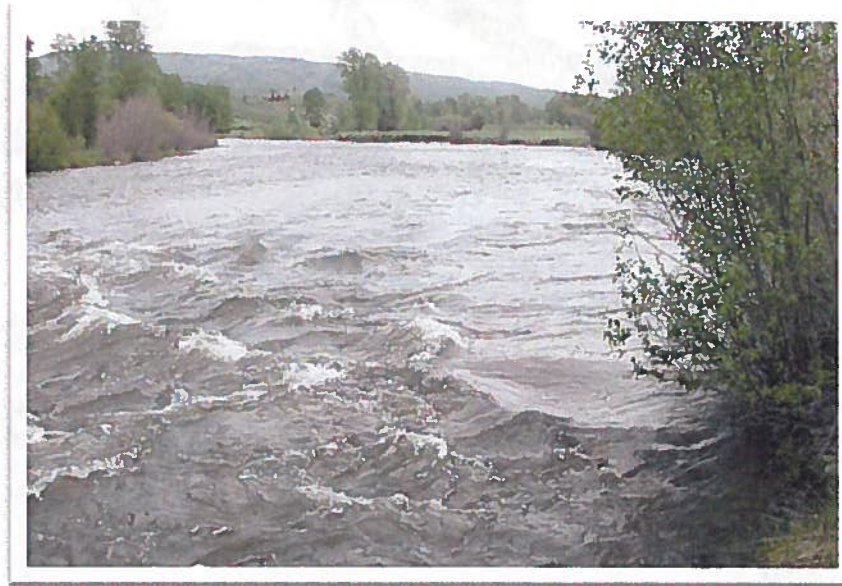
Figure 34. A J-Hook rock vane at bankfull stage, Little Snake River, Colorado. Note the variation in velocity distribution.
