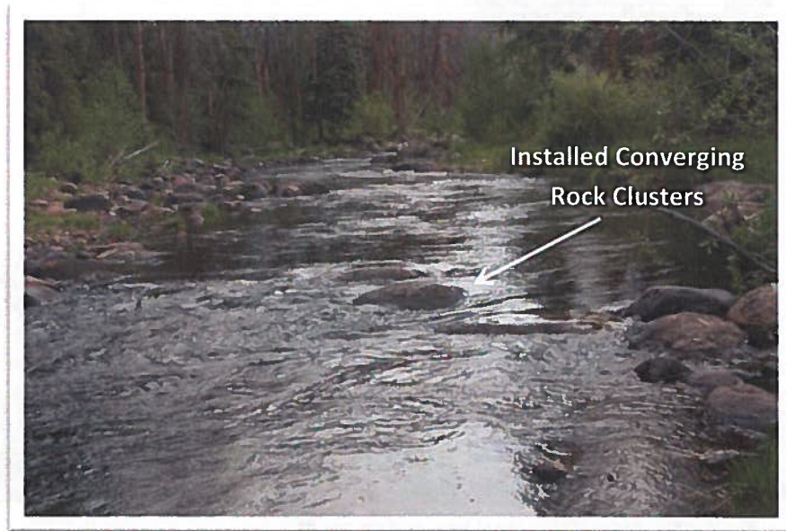
Figure 38. Installed converging rock clusters at low flow on the Laramie River, Colorado. These structures create excellent holding cover for trout.
