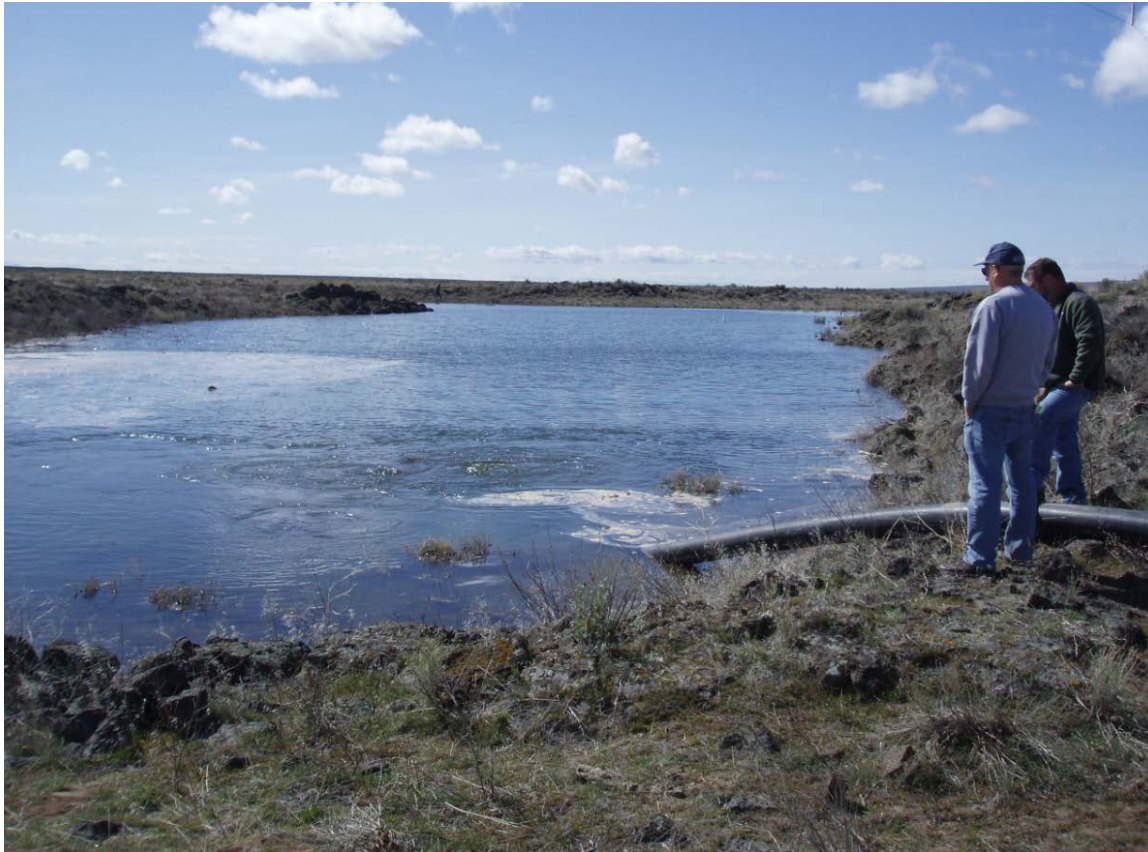
Basin #3 at full pool and steady state leakage rate of 4.8 cfs.
