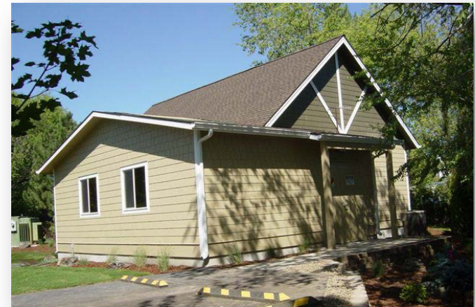
Swift ASR well house
