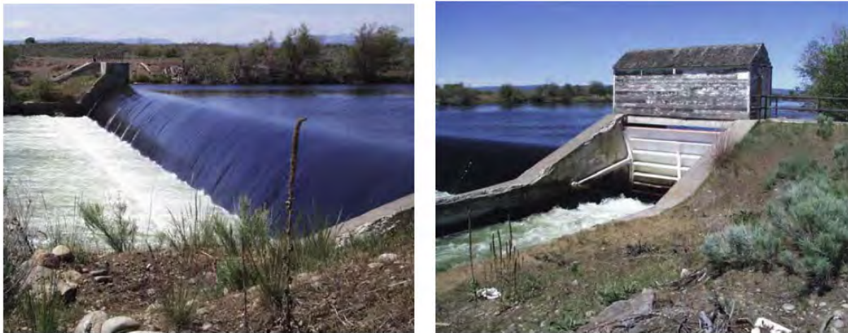
Figure 13. Cross Cut Diversion Dam and radial headgate on the Henrys Fork River.
