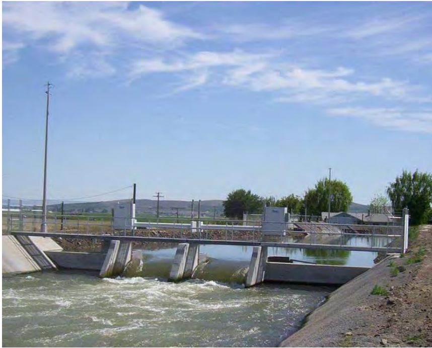
Figure 30. Photo of an automated canal system with a Langemann gates structure.
