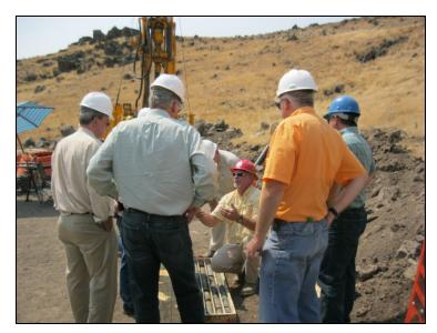
**Photo:** *IWRB* members examining core drilling investigation work at the proposed Galloway dam site to determine the site's suitability for development of a large dam and reservoir project.
