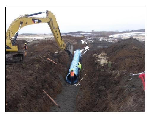
**Photo:** The North Fremont Canal System, Inc. received a \$2,500,000 loan to construct Phase 4 of Marysville project to convert open canals to gravity-pressurized pipelines.
