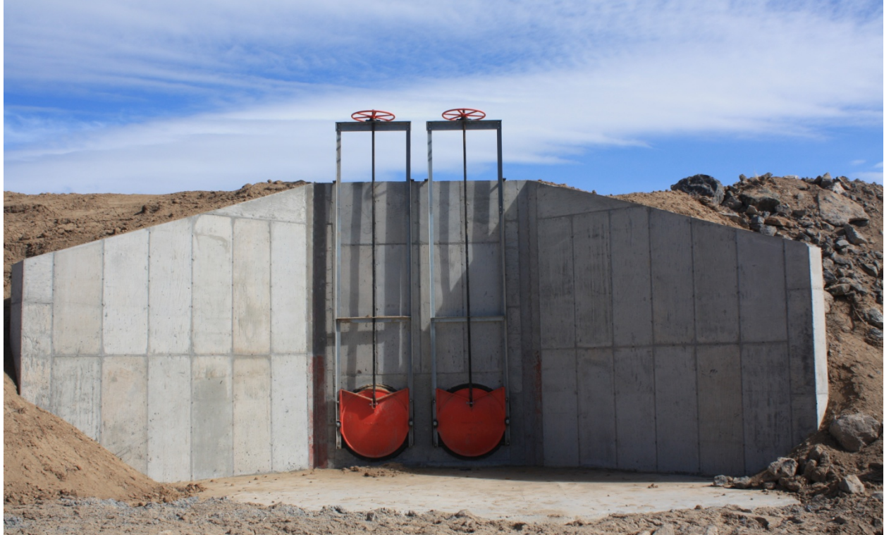
Photo 2 – Diversion structure concrete head gate and twin 36-inch diameter canal gates.
