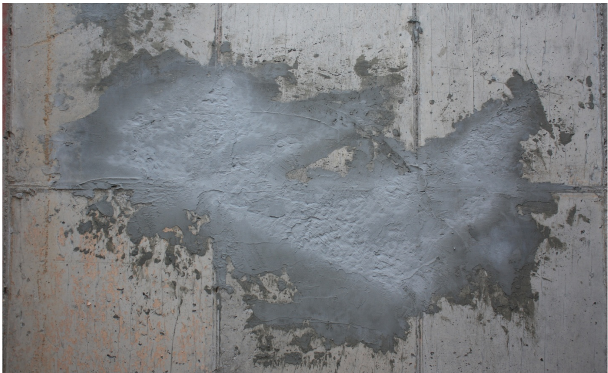
Photo 9 – Detail of grouted concrete patch on face of concrete wall on the downstream face of the diversion structure. This picture is typical of several large patches. The reason for the grouting is unknown.
