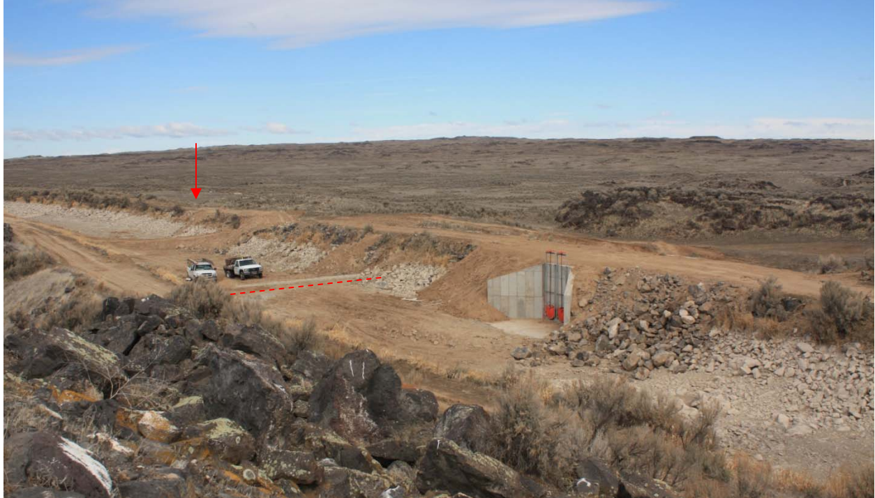
Photo 12 – Photo of Milner-Gooding canal and diversion structure head gates. Note the footing for the canal check dam structure in front of the pickup trucks running perpendicular to the flow of water (dashed red line). Also, 8-inch diameter recharge turn-out previously located downstream of check dam has been removed from the north canal bank (red arrow).
