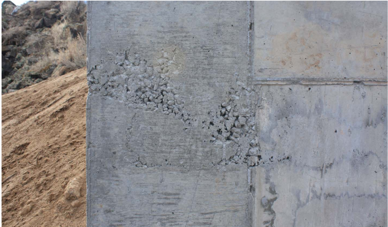
Photo 8 – Detail of exposed aggregate on the downstream face of the diversion structure.
