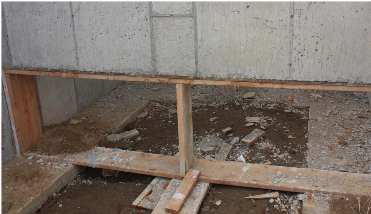
Photo 4 – Concrete outlet and control structure Milner-Gooding canal is located behind the concrete wall. Note baffle wall and block-out for submerged orifice.
