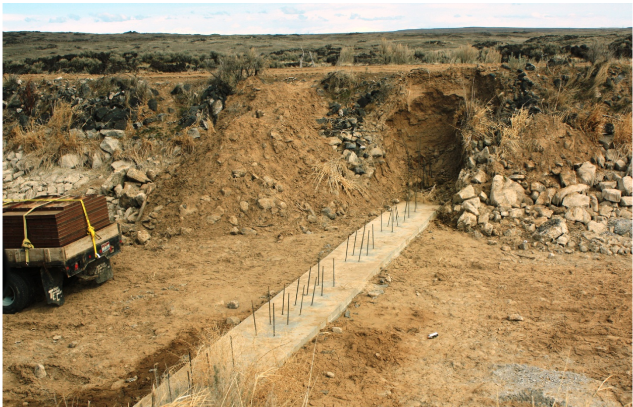
Photo 13 – Detail of canal check dam concrete footing.
