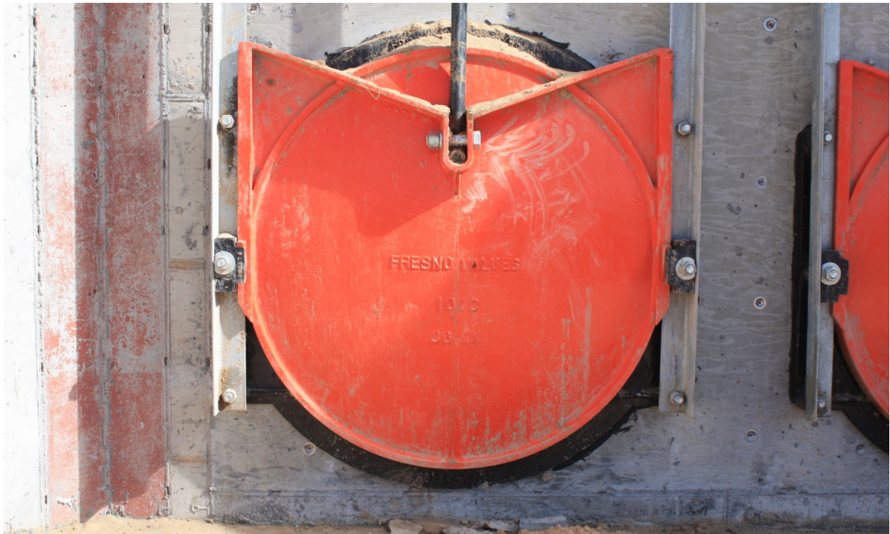
Photo 3 – Detail of 36-inch diameter canal gate seated on left 36-inch diameter turnout.
