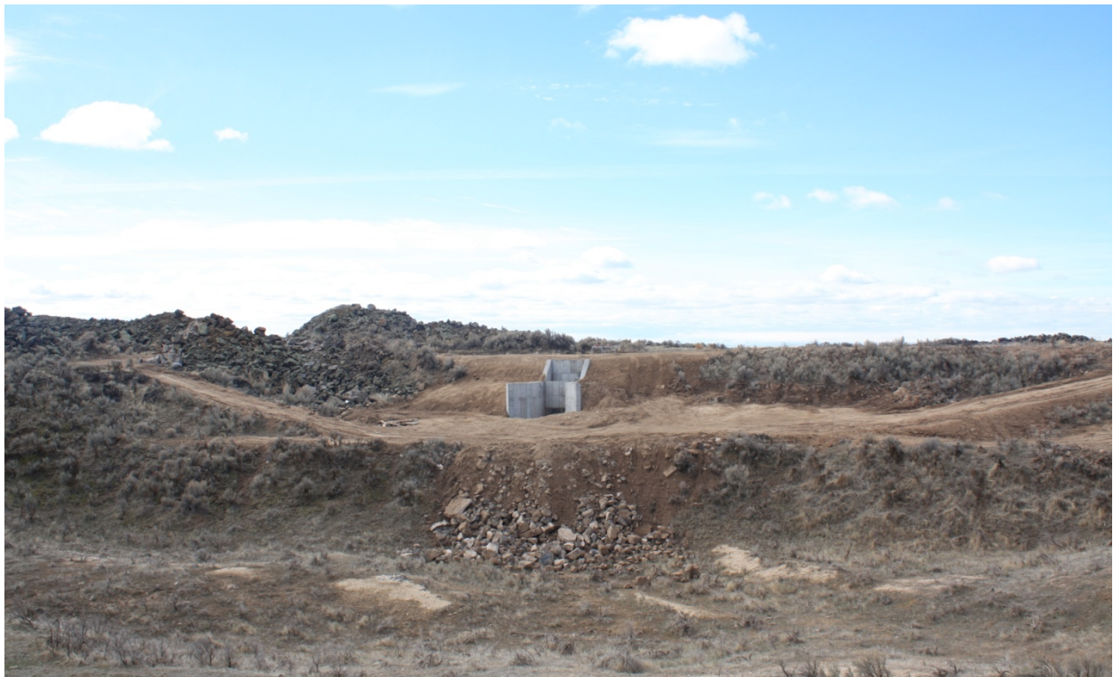
Photo 11 – Photo of outlet diversion structure and recharge basin. No rip-rap or other energy dissipation improvements were installed at the time of the site visit.
