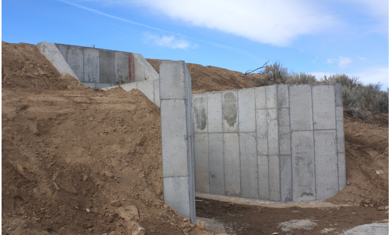
Photo 10 – Photo of outlet diversion structure. At the time the picture was taken backfill appeared to be comprised exclusively of native barrow material.
