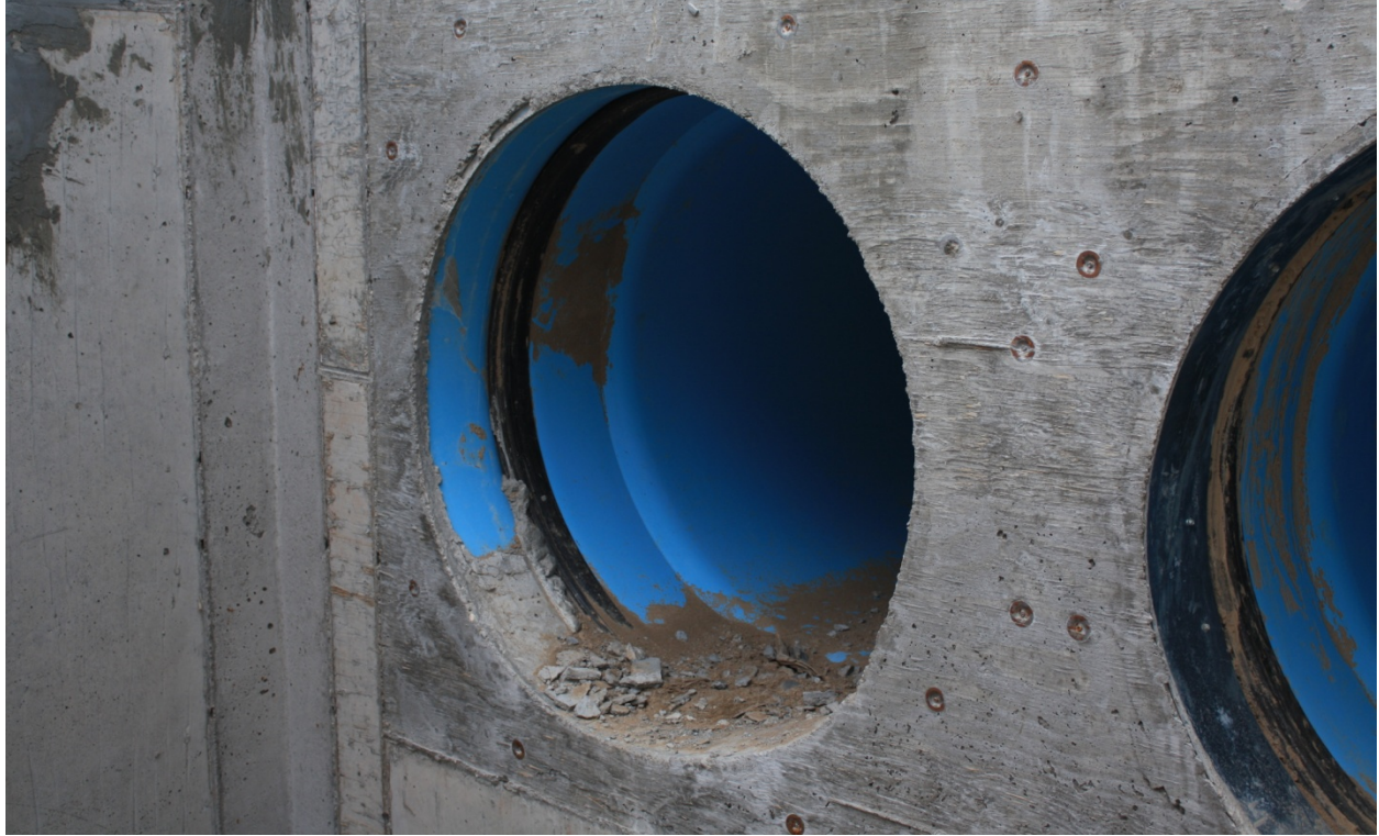
Photo 6 – Picture of the 36-inch diameter pipe outlets located upstream of the baffle wall.
