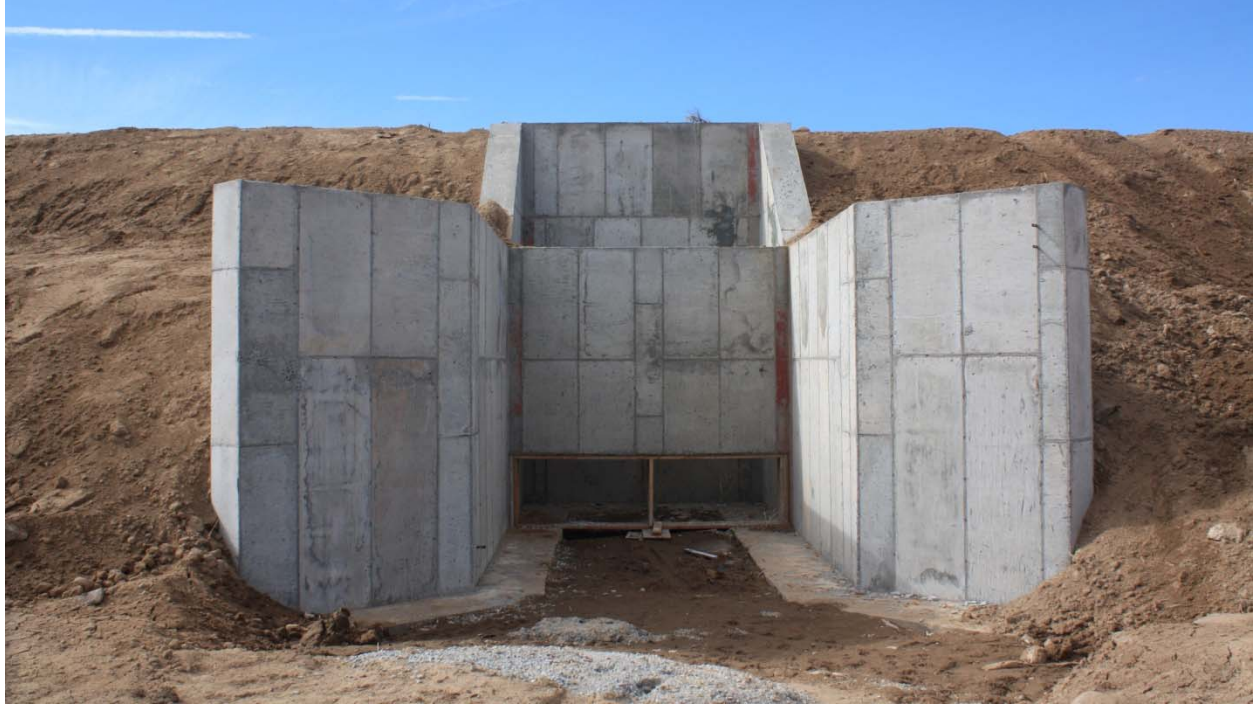
Photo 4 – Concrete outlet and control structure Milner-Gooding canal is located behind the concrete wall. Note baffle wall and block-out for submerged orifice.
